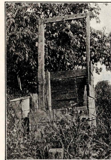
Fig. 15. An Open Bucket Well.
