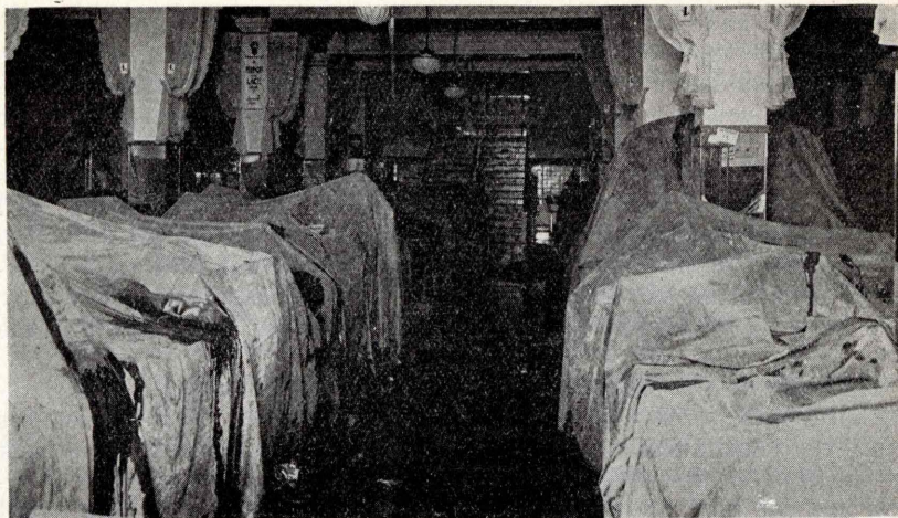
Courtesy Fire Engineering and Int. Assoc. Fire Chiefs Cutting down the loss in a dry goods store fire by coverage.
