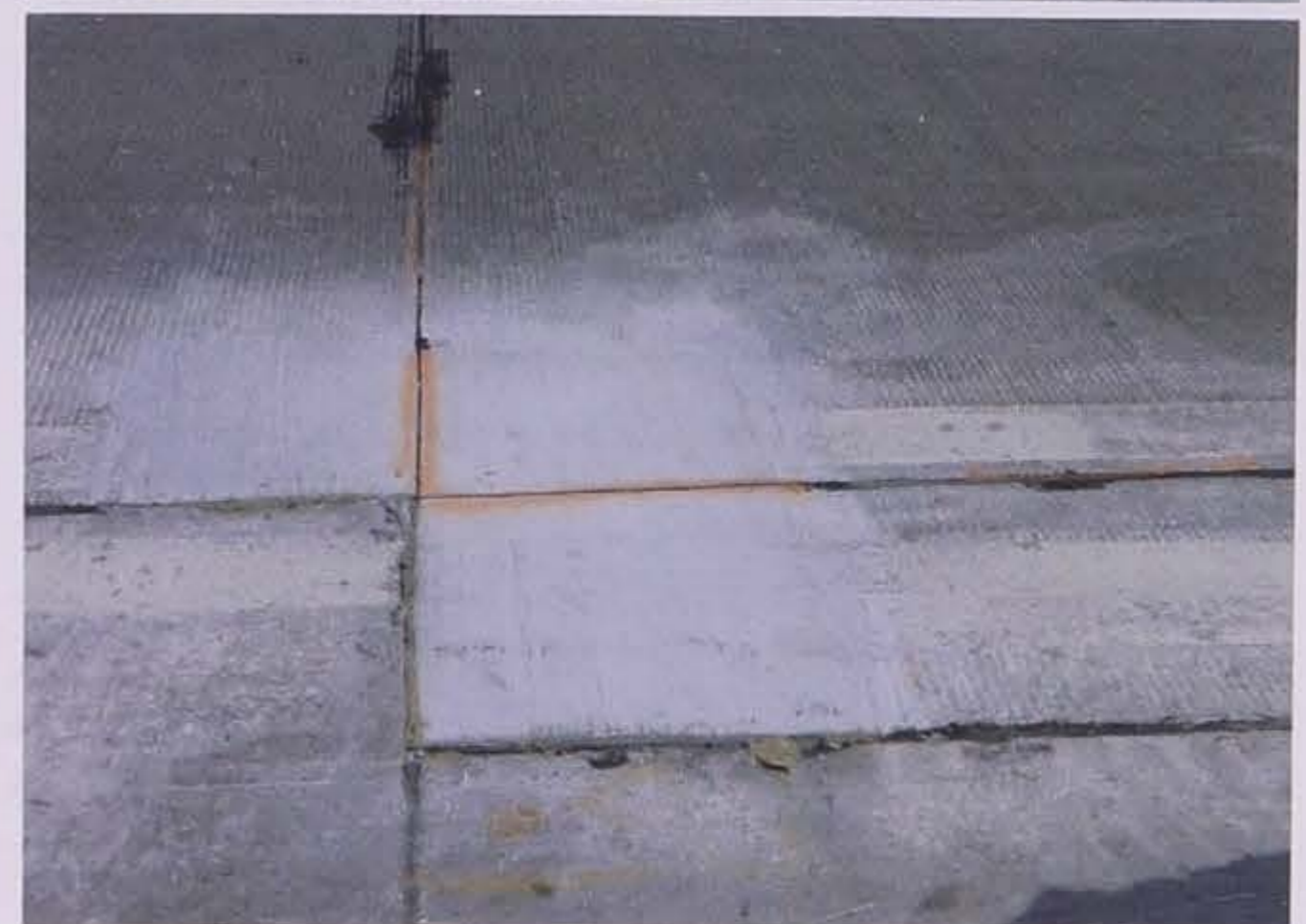
Figure 5.23. Completed joint repairs (Frentress and Harrington 2012)
