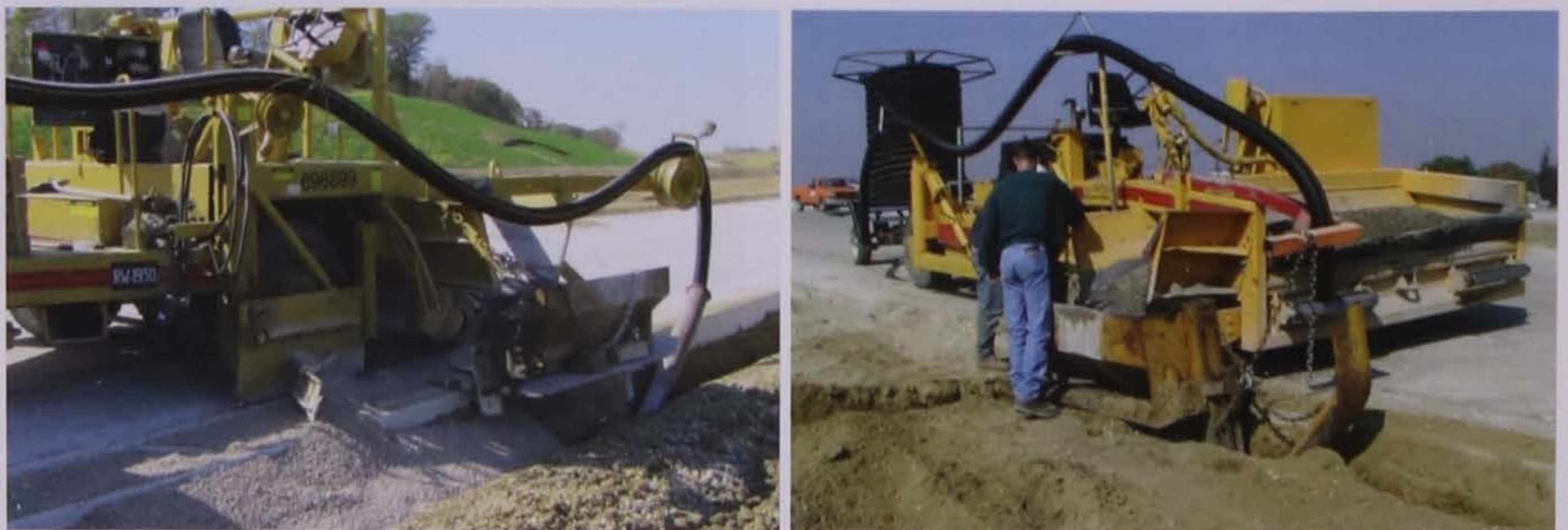
Figure 7.13. Automated equipment installing CPE edgedrains (courtesy of Kevin Merryman, Iowa DOT)
