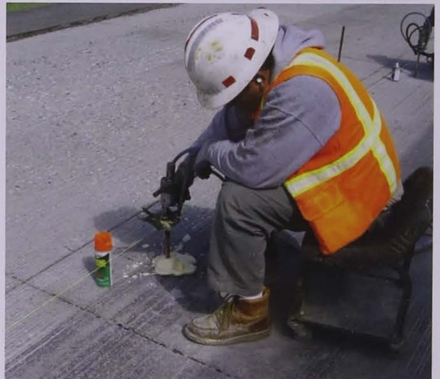
Figure 4.10. Injecting polyurethane (photo courtesy of WSDOT)
