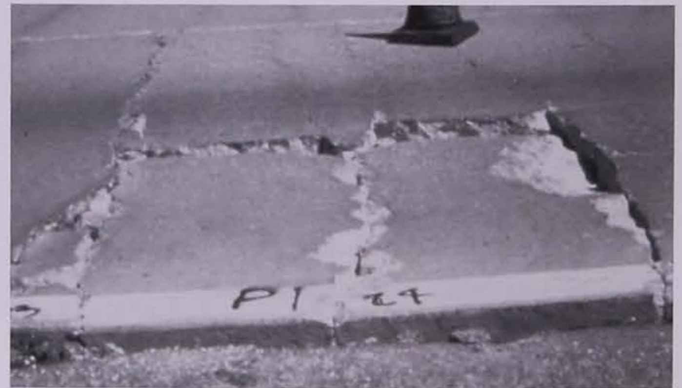
Figure 6.3. Schematic illustration (left) and photograph (right) of CRCP punchout distress
