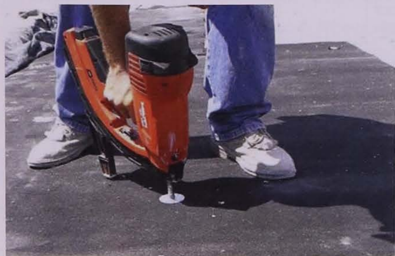
Figure 11.18. Fastening nonwoven geotextile interlayer (Harrington and Fick 2014)
