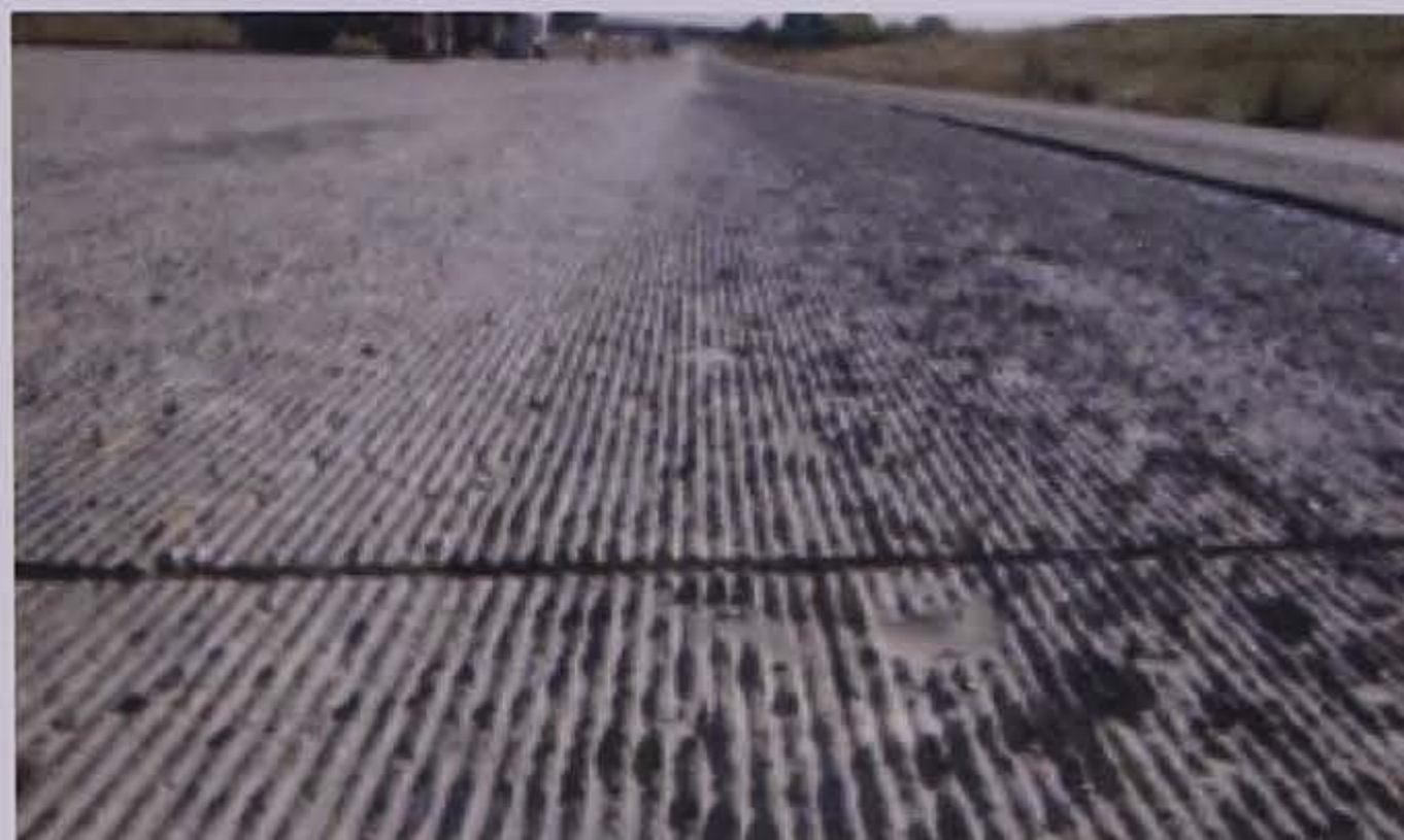
c. Conventional diamond ground surface
