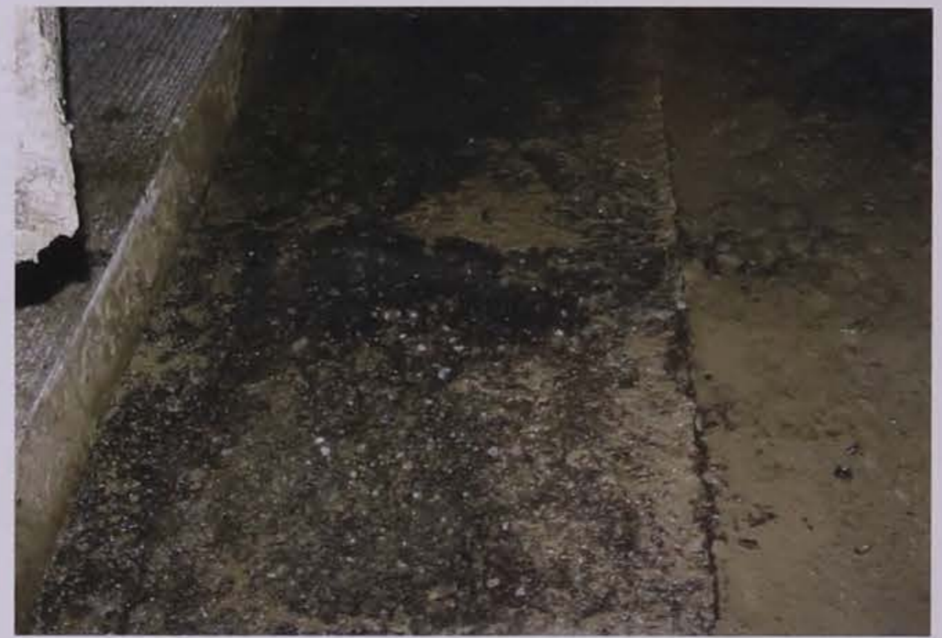
Figure 11.9. Stripping of asphalt interlayer (photo courtesy of Dan DeGraaf, Michigan Concrete Association)
