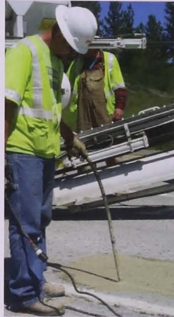
a. Consolidating the patching material
