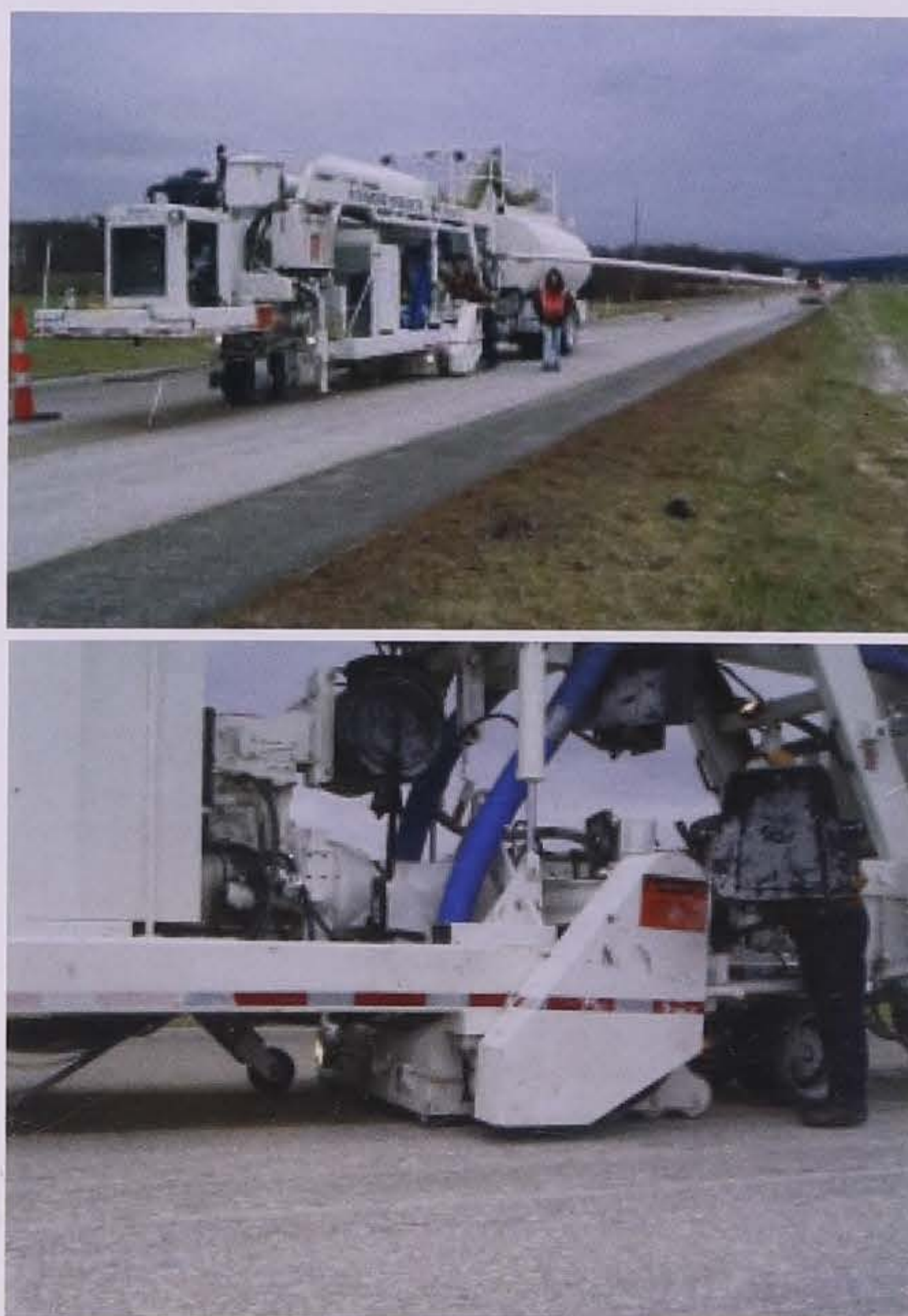
Figure 9.13. Diamond grinding machine (top) and cutting head (bottom) (courtesy of John Donahue, Missouri DOT)
