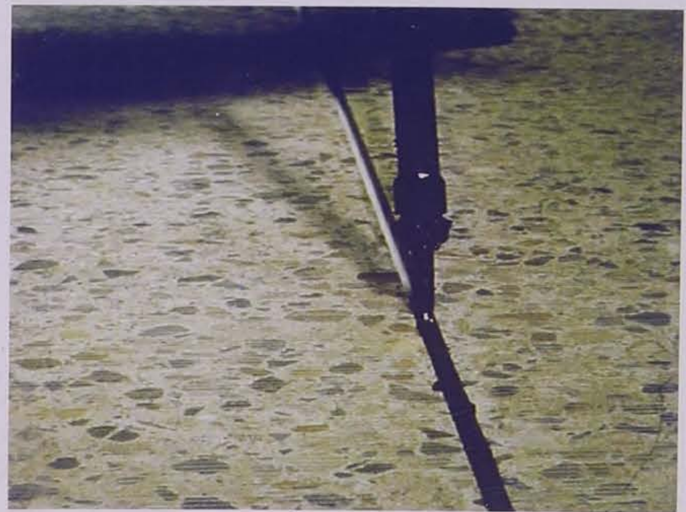
Figure 10.11. Installation of hot-applied joint sealant
