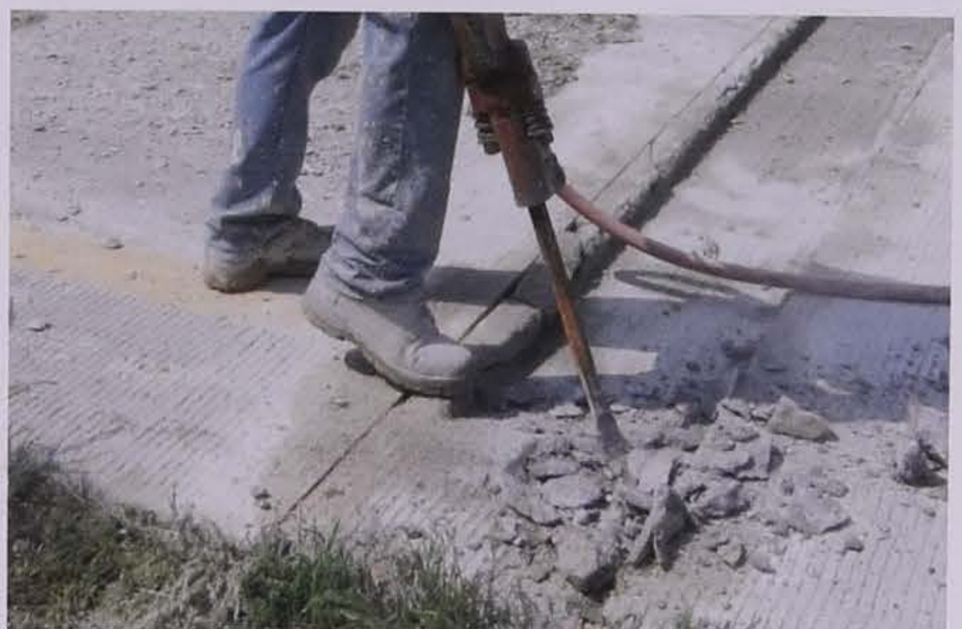
Figure 5.12. Repair area prepared using the chip-and-patch (Types 1 and 3) procedure
