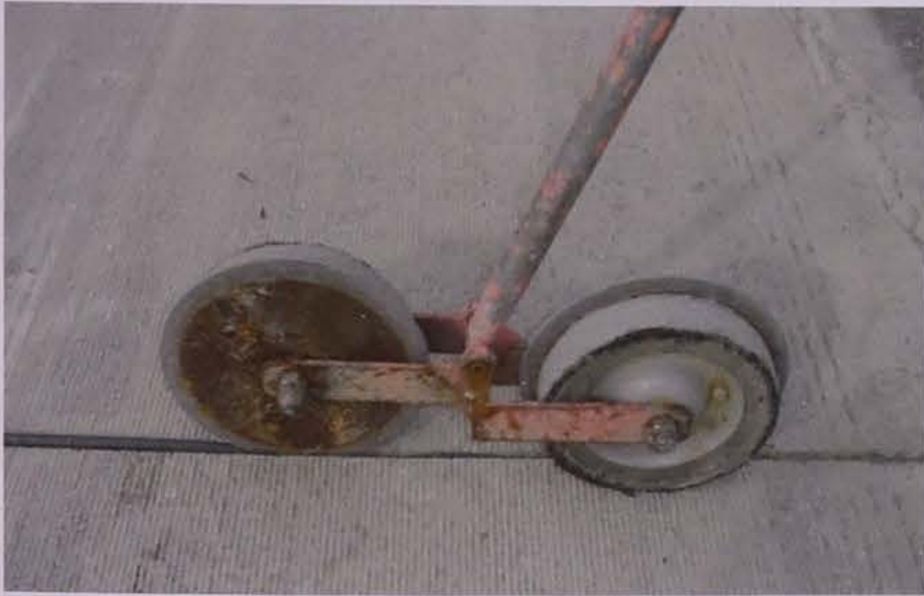
Figure 10.10. Installation of the backer rod
