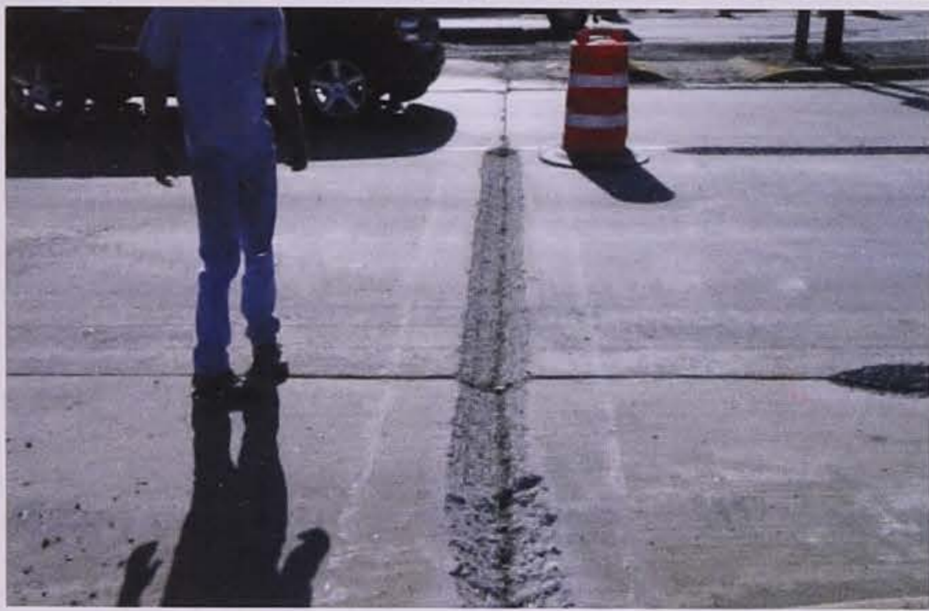
Figure 5.14. "V" shape milling head (top) and milling pattern (bottom) (Frentress and Harrington 2012)
