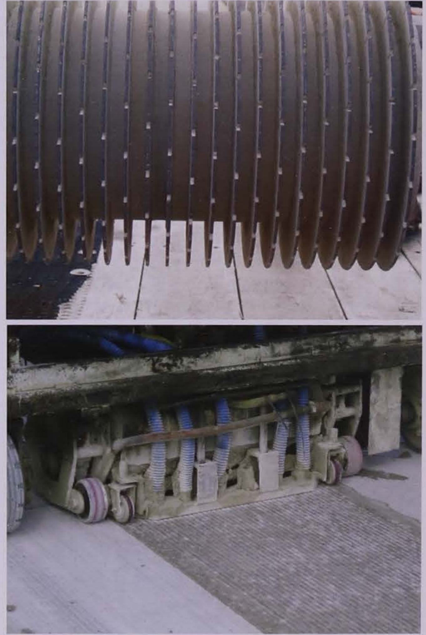
Figure 9.18. Diamond grooving head (top) and grooving operation (bottom)
