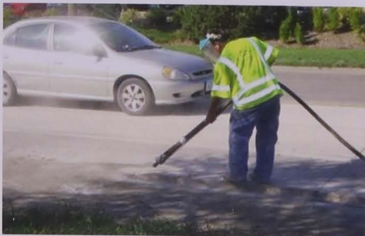
Figure 5.17. Sandblasting to remove loose debris
