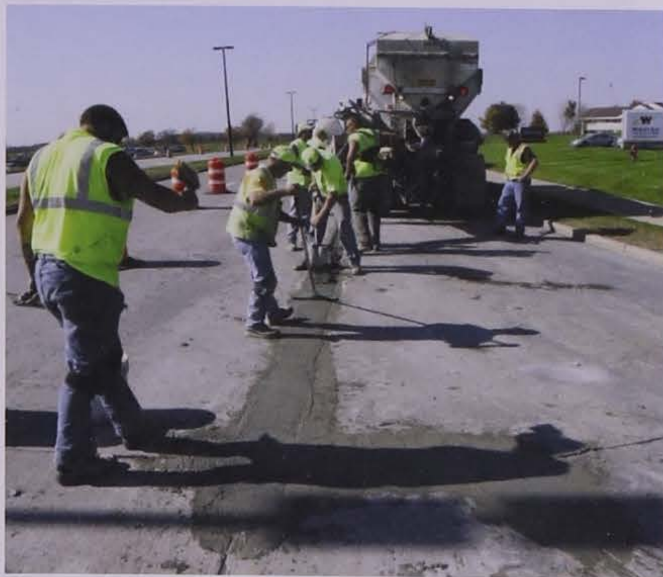
Figure 5.21. Placement of repair material for long joints using mobile concrete truck (Frentress and Harrington 2012)
