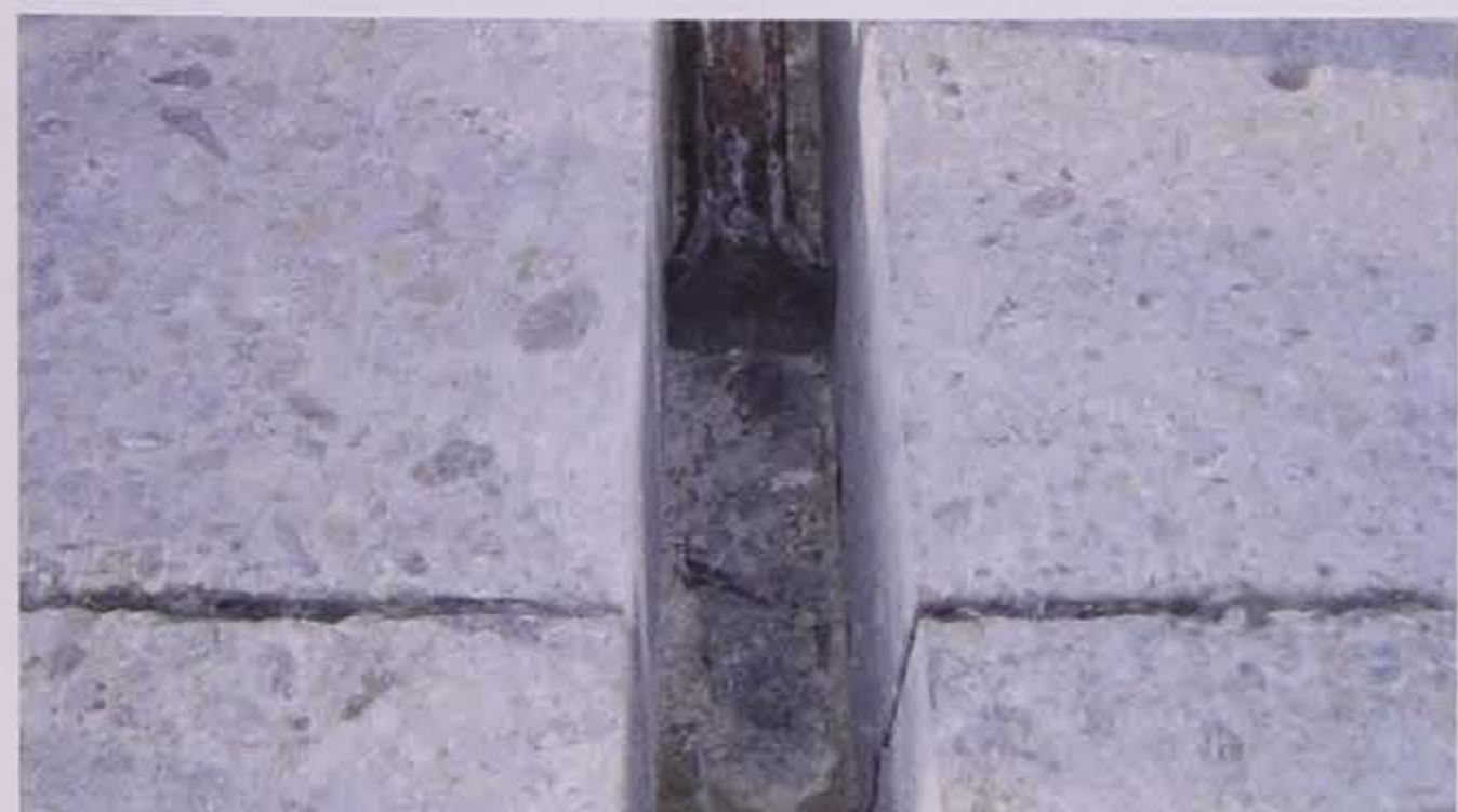
Figure 8.10. Leveling the bottom of the dowel bar slot (Pierce, Uhlmeier, and Weston 2009)
