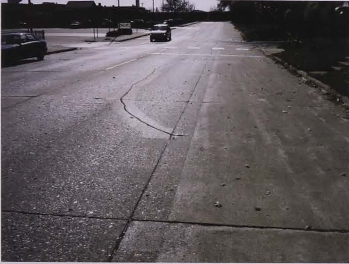
Figure 5.25. Diamond grinding of PDR (Frentress and Harrington 2012)
