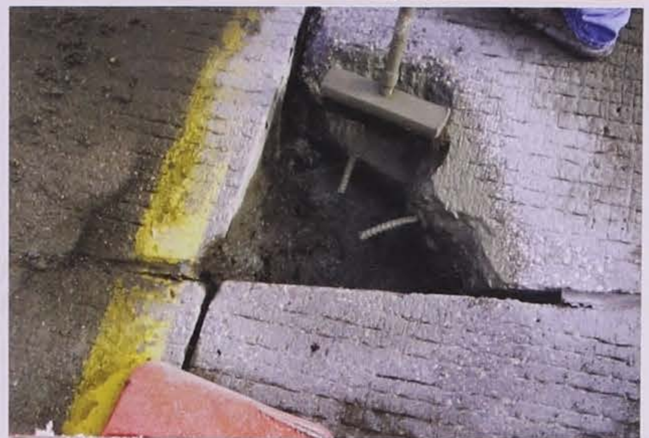
Figure 5.20. Application of cement grout as bonding agent (Frentress and Harrington 2012)
