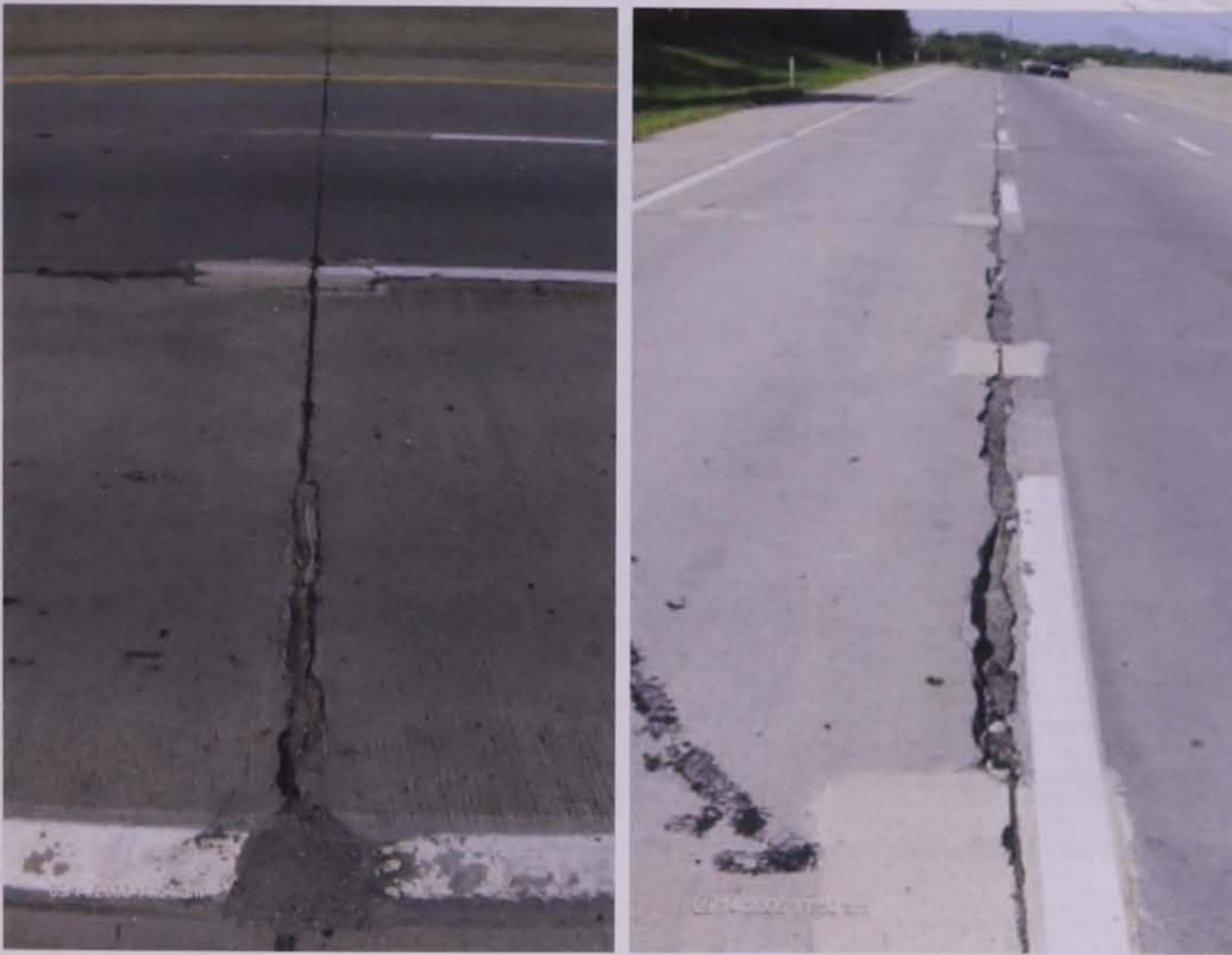
Figure 5.3. Candidates for Type 2 repairs (Frentress and Harrington 2012)
