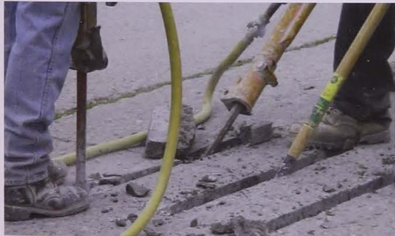
Figure 8.9. Operating jackhammers at no more than a 45-degree angle (Pierce, Uhlmeier, and Weston 2009)
