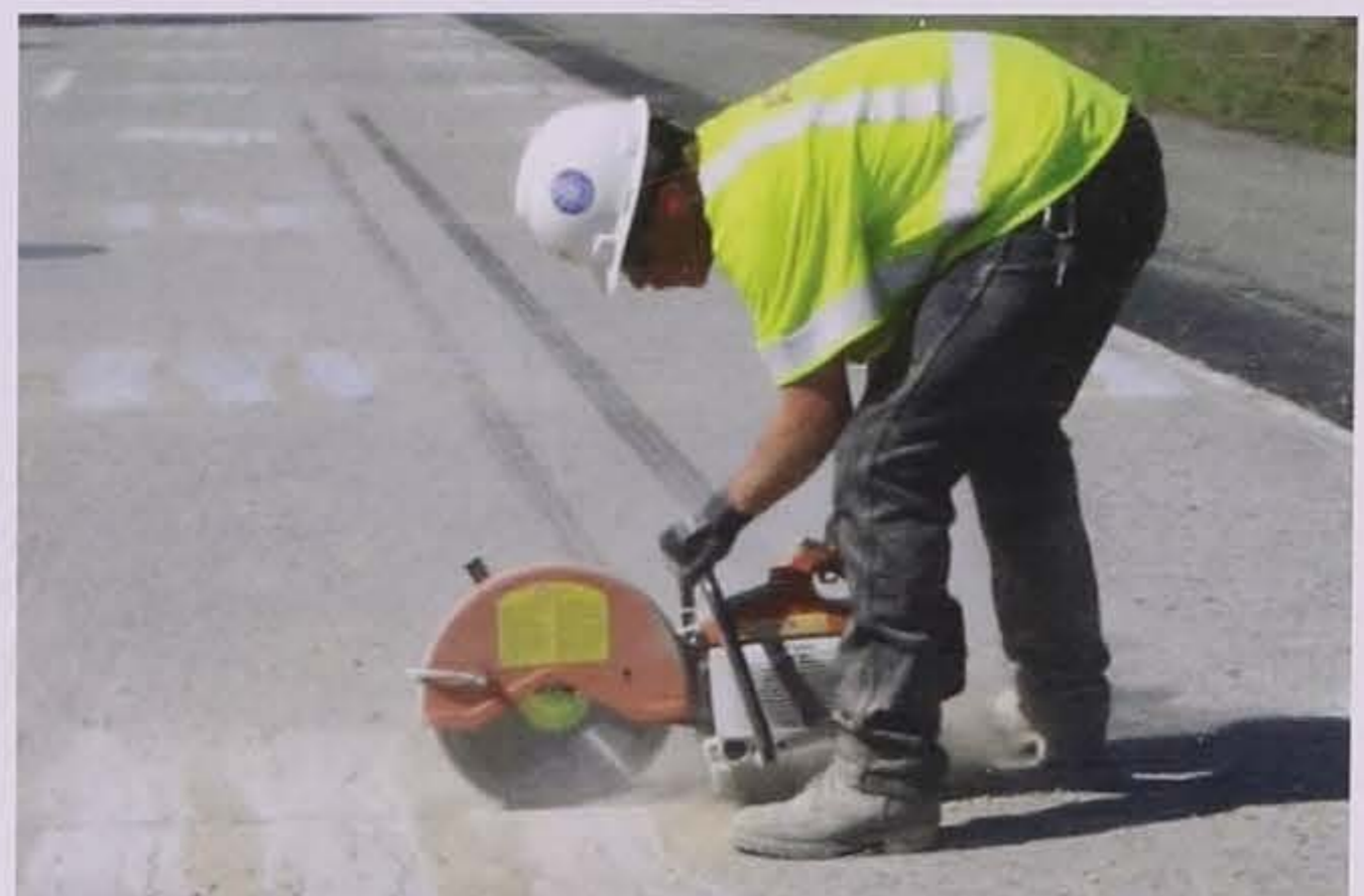
Figure 8.17. Re-establishing the transverse joint in patching material (Pierce, Uhlmeyer, and Weston 2009)
