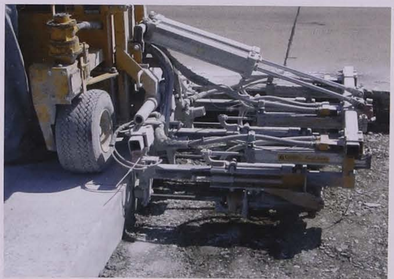
Figure 6.12. Example of gang drill used for dowel bar installation
