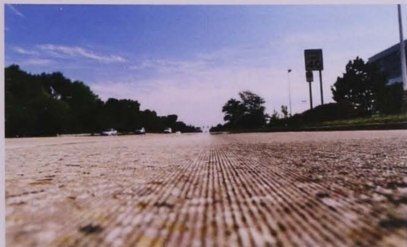
Figure 9.2. Surface texture provided by diamond grinding (courtesy of John Roberts, IGGA)
