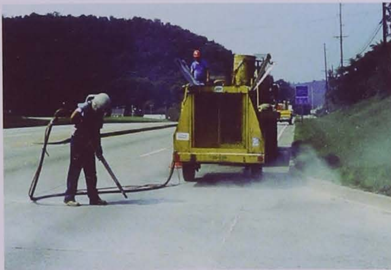
Figure 10.9. Sandblasting along a transverse joint
