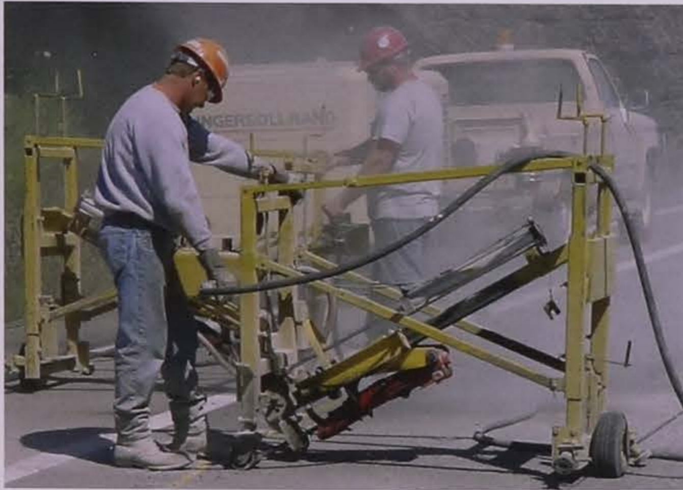
Figure 8.19. Drilling holes for cross stitching
