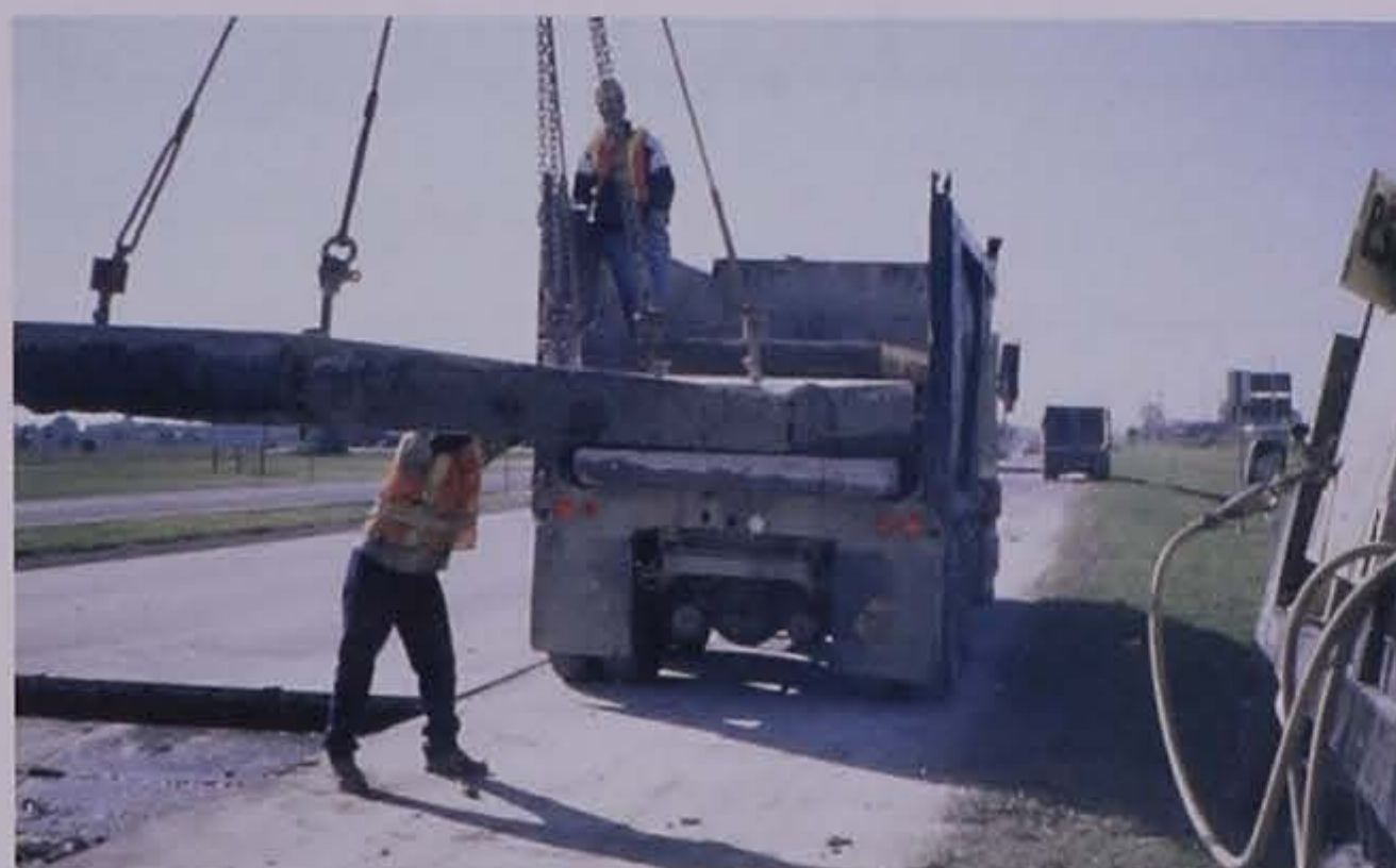
Figure 6.10. Lift-out method of slab removal
