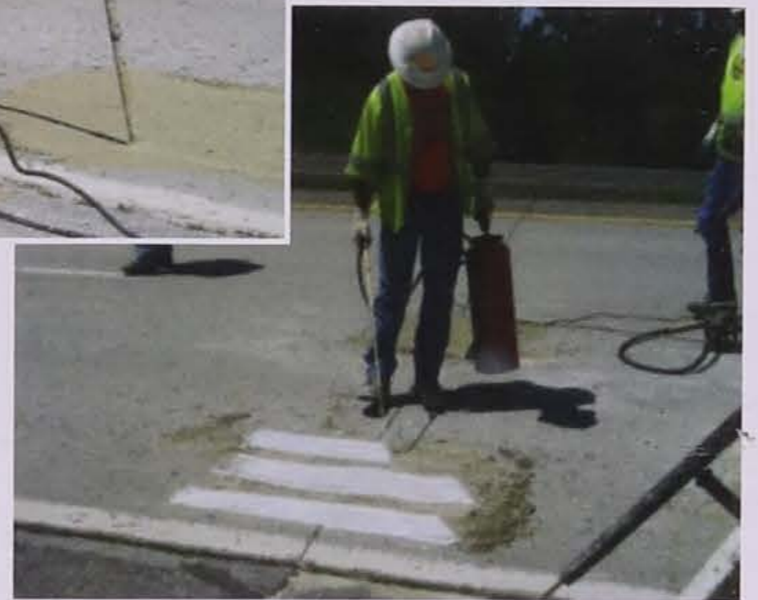
c. Applying curing compound
