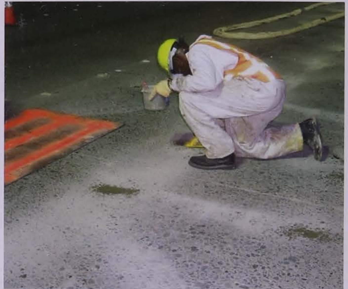
Figure 4.9. Patching drill holes (photo courtesy of WSDOT)
