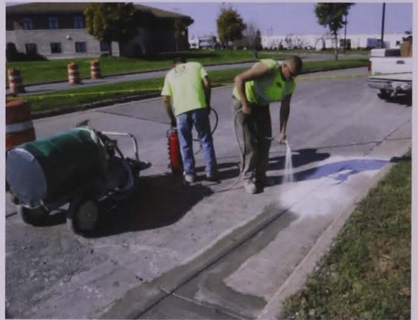
Figure 5.24. Repair material curing operation (Frentress and Harrington 2012)
