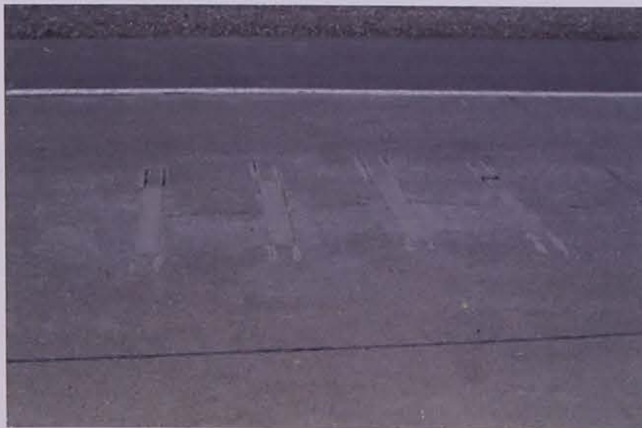
Figure 8.22. Completed slot stitching on longitudinal crack (courtesy of John Donahue)
