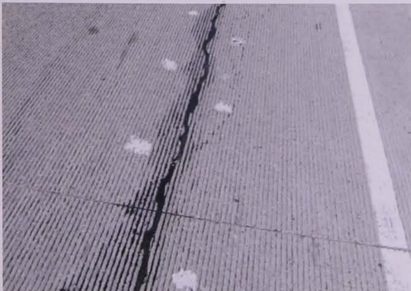
Figure 8.20. Completed cross stitching
