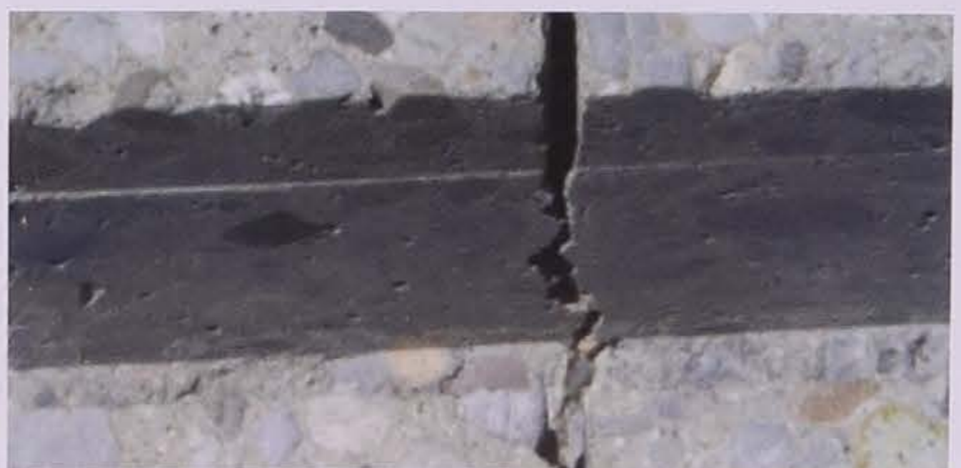
b. Final cleaned slot surface
