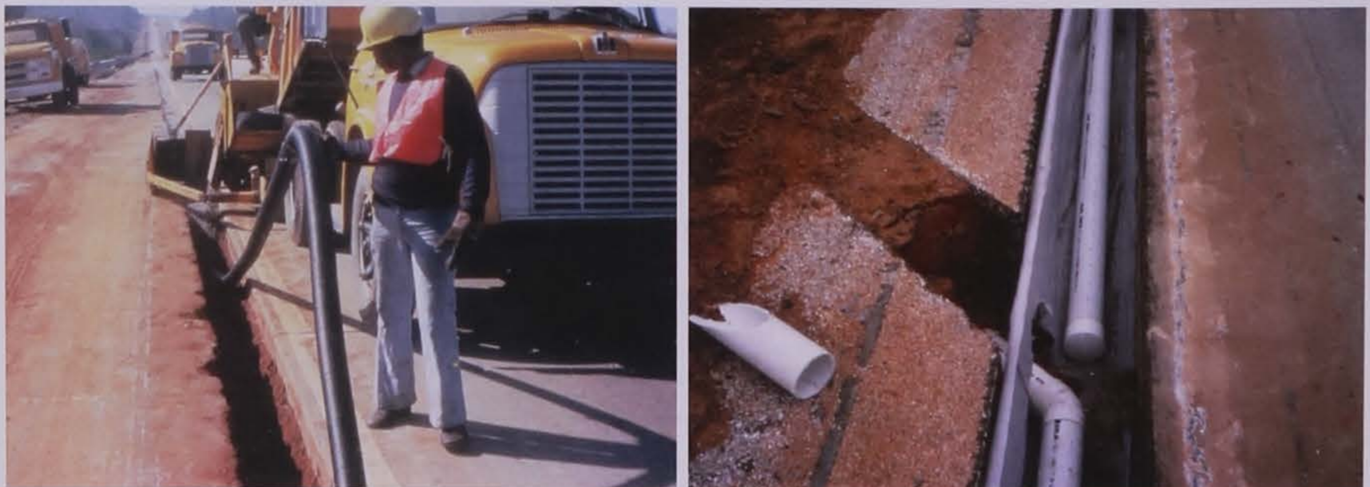
Figure 7.7. Corrugated (left) and rigid (right) pipe edgedrains
