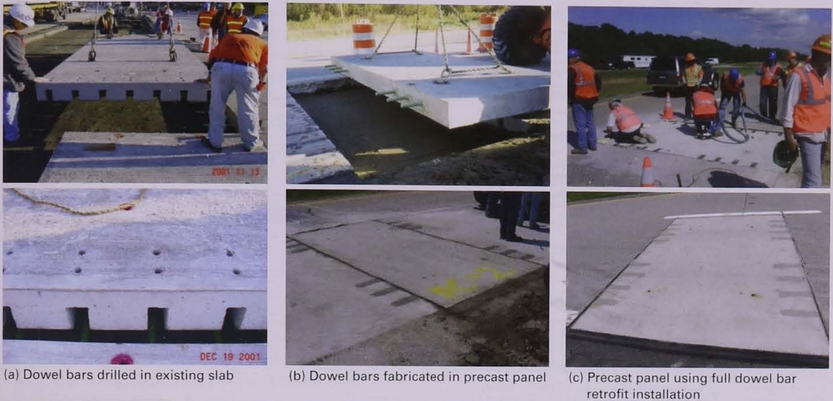
Figure 6.17. Placement of different precast repair systems (Tayabji, Ye, and Buch 2012)
