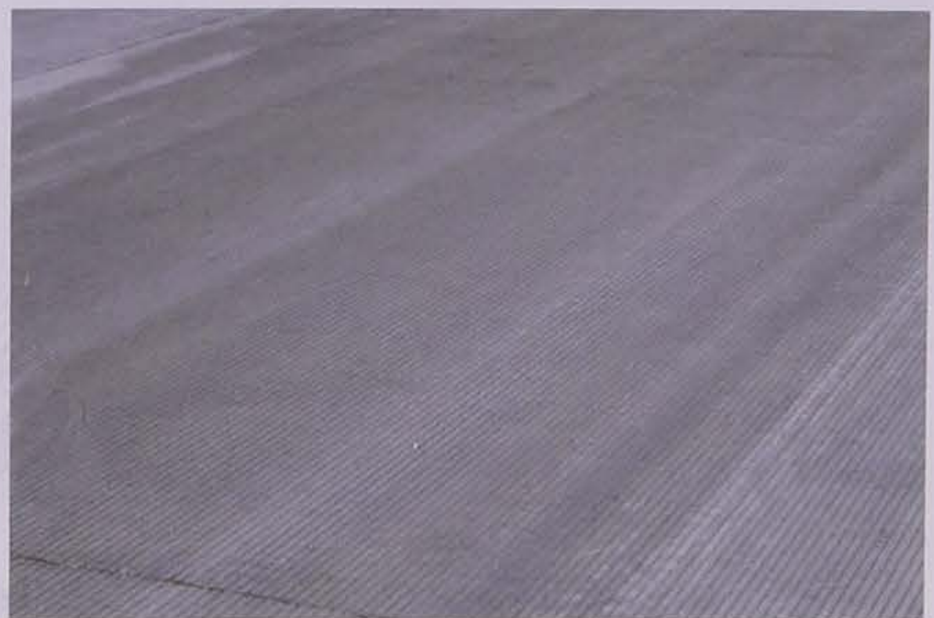
Figure 9.6. Longitudinally grooved surface
