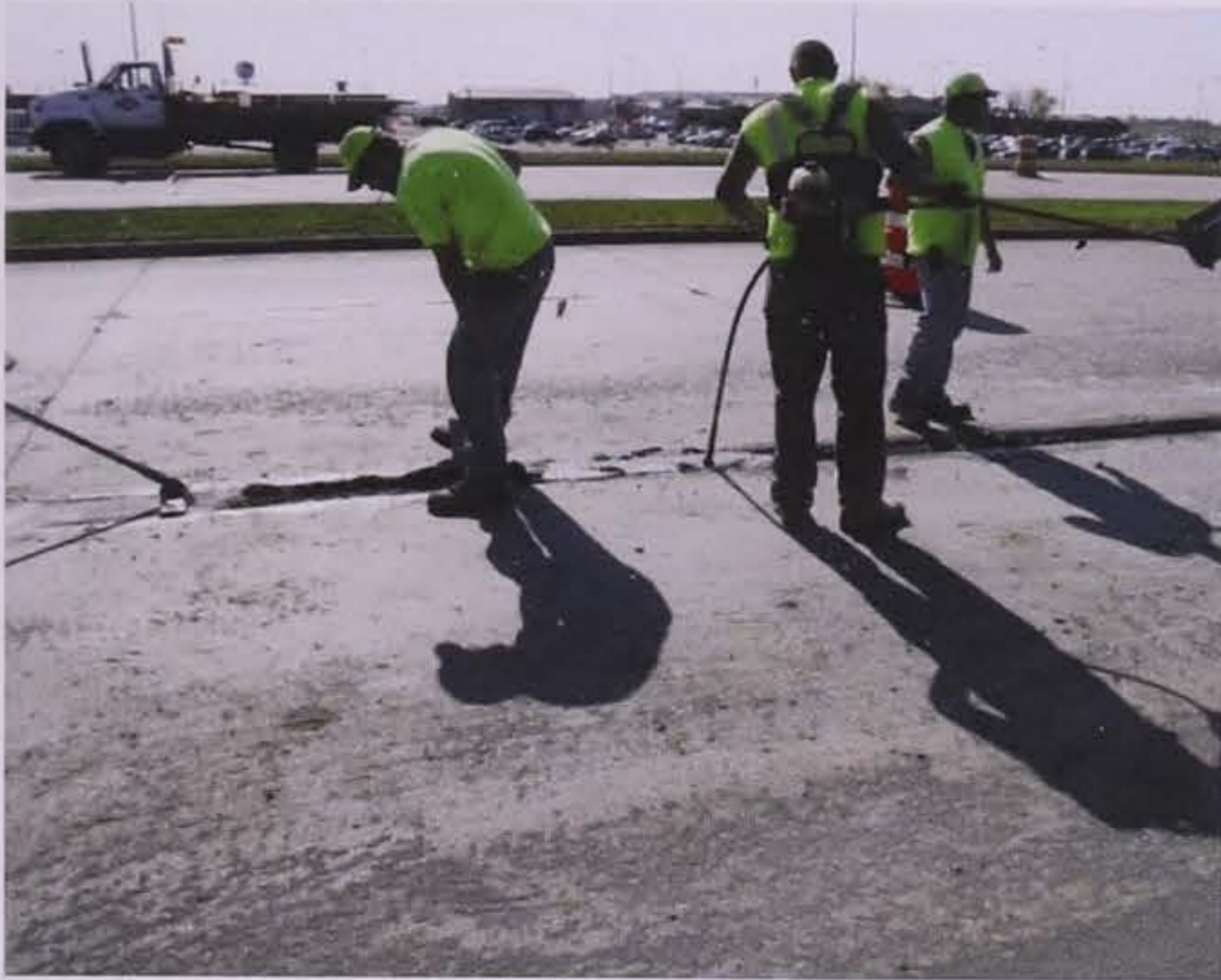
Figure 5.22. Consolidation of repair material using internal vibrator (Frentress and Harrington 2012)
