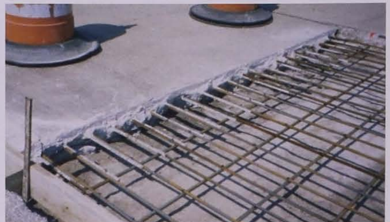
Figure 6.14. CRCP repair with longitudinal and transverse steel.
