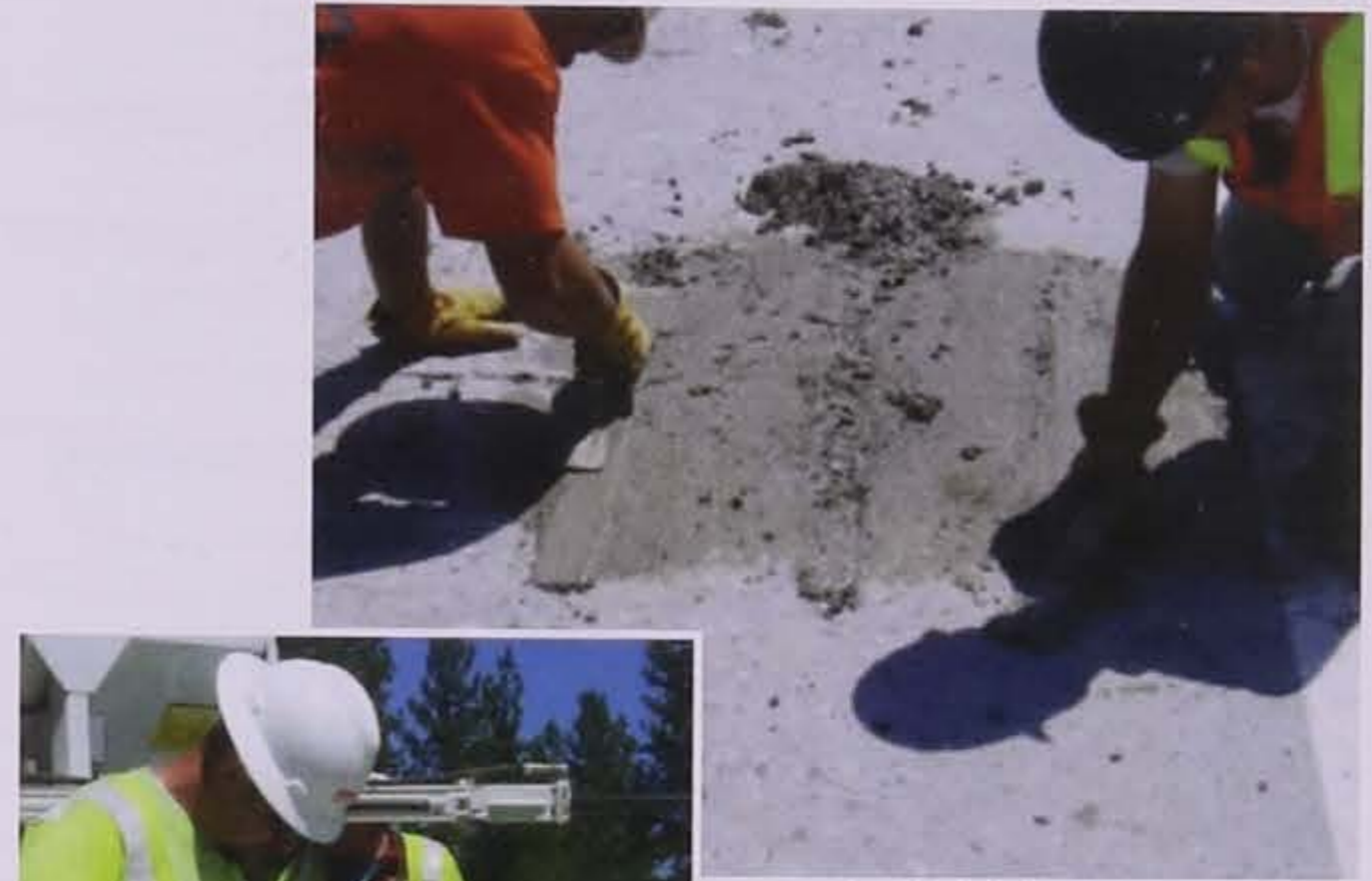
b. Finishing the patching material
