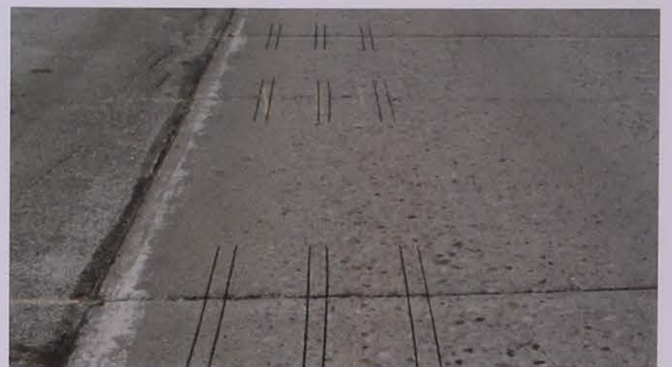
a. Nonskewed transverse joints
