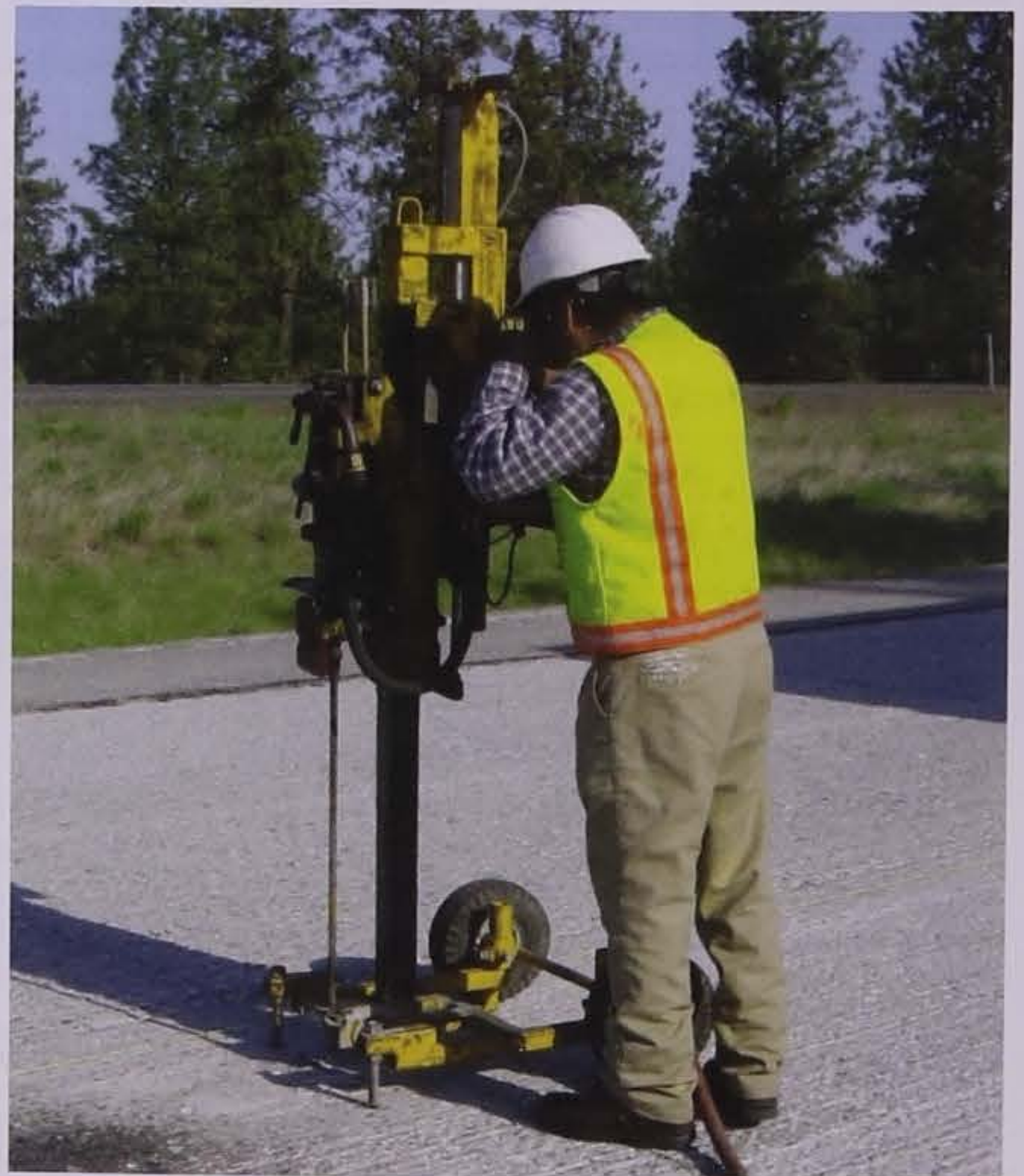
Figure 4.8. Drilling injection holes (photo courtesy of WSDOT)
