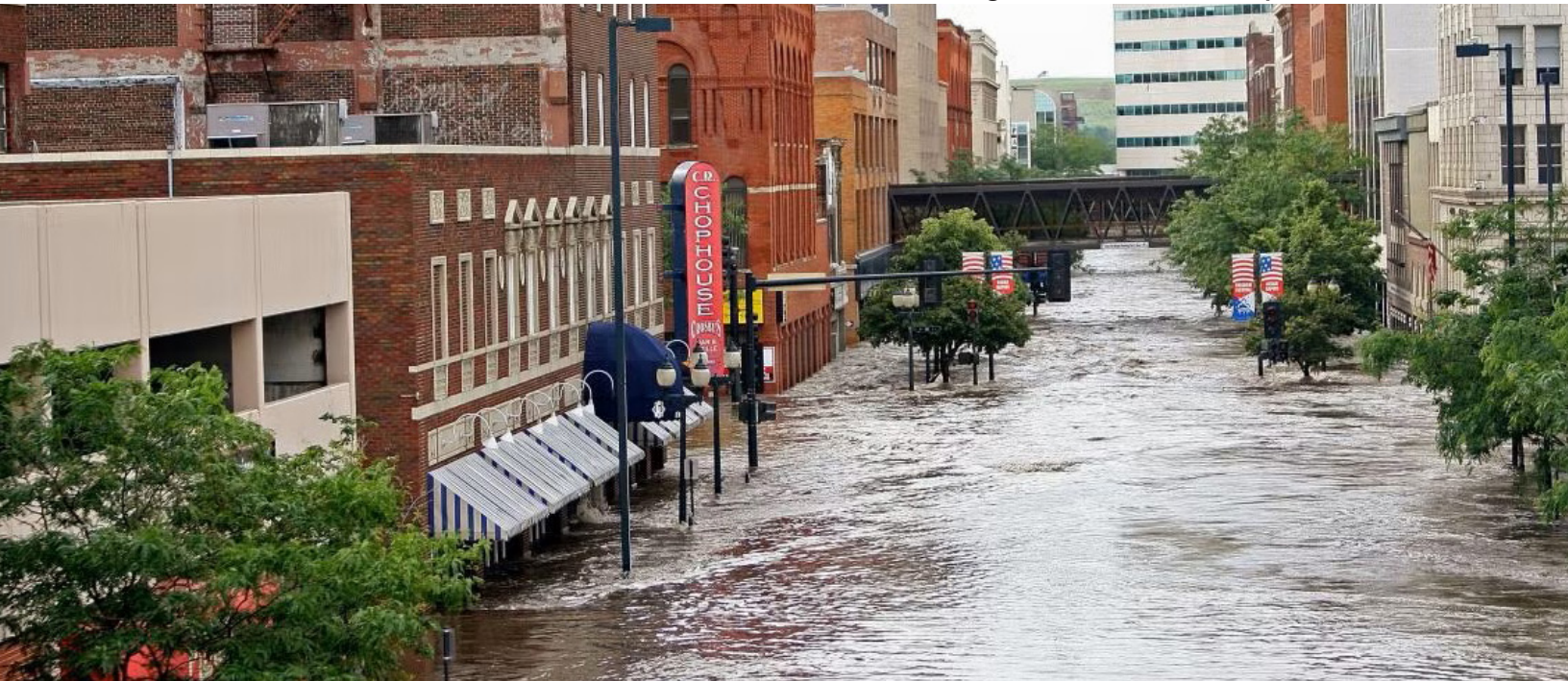
Flooding in downtown Cedar Rapids in June 2008.
