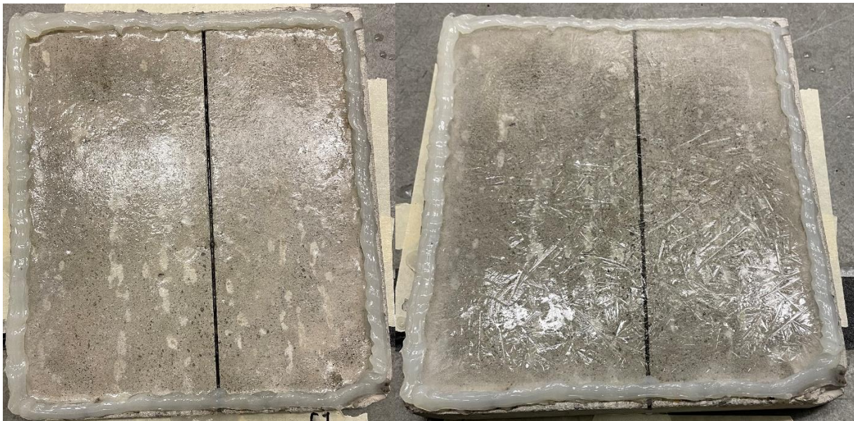
Figure 3. Concrete sample with a thin black ice layer (left) and a thicker ice layer (right)
