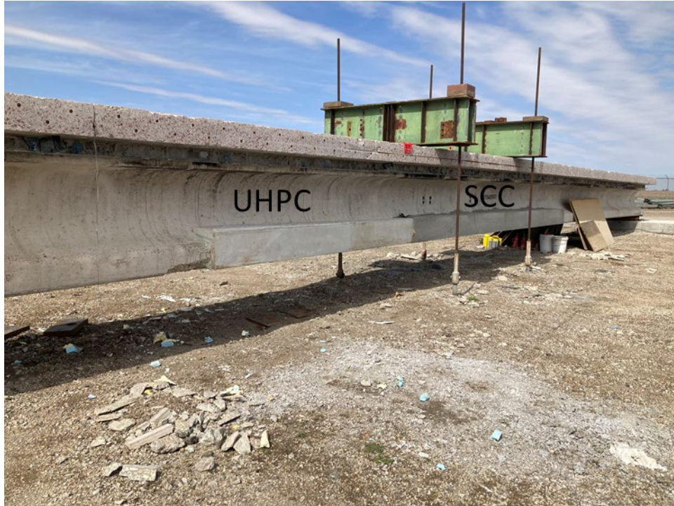
Figure 81. UHPC and SCC repair sections fully cast
