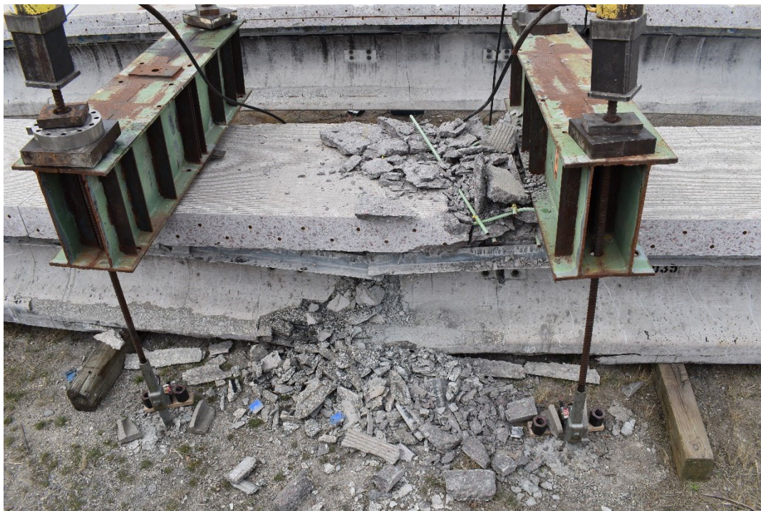
Figure 59. Girder E after failure at midspan
