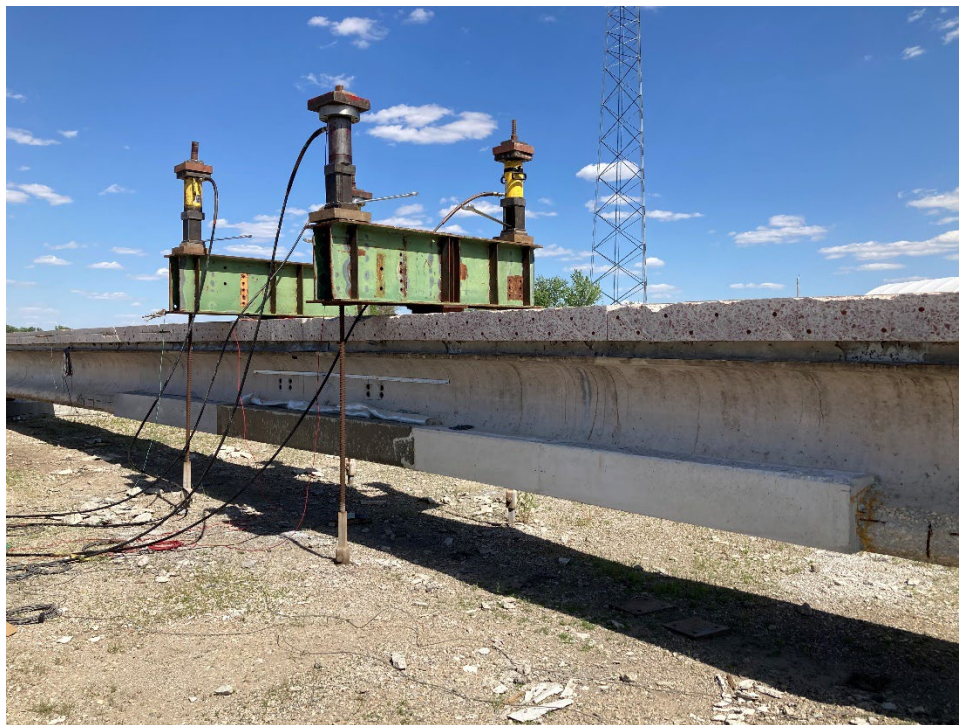
Figure 88. Load test of repaired girder
