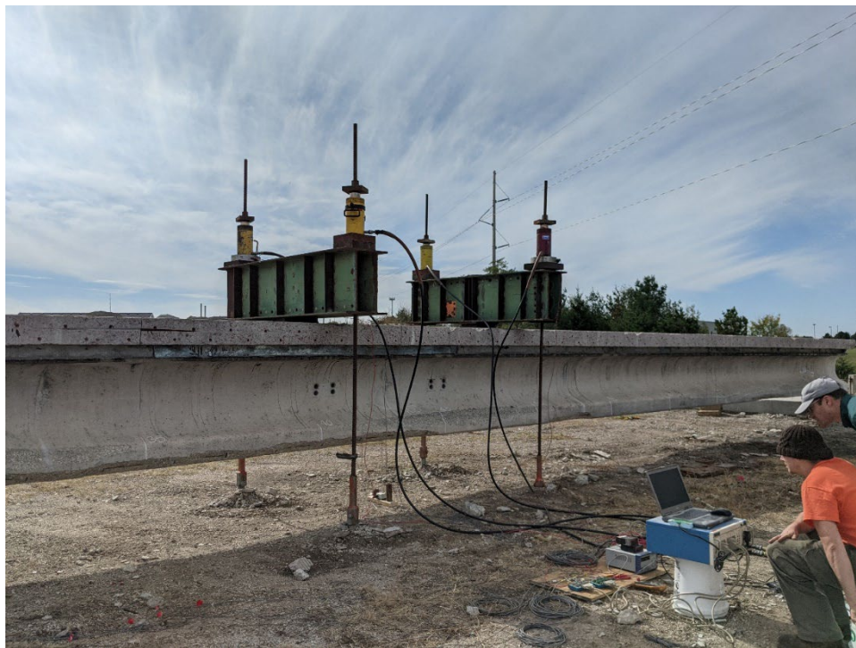
Figure 63. Girder G bending load test
