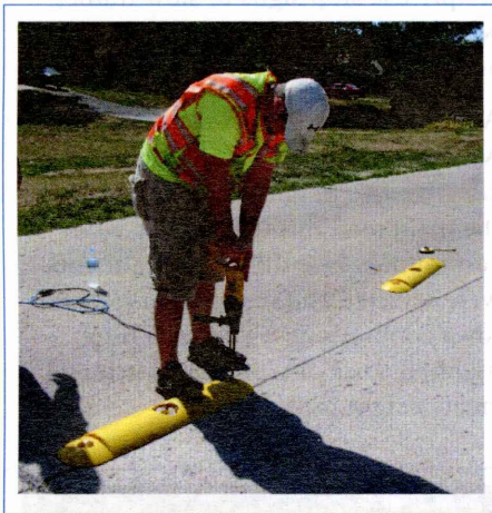
Installation of raised curbing using bolts
