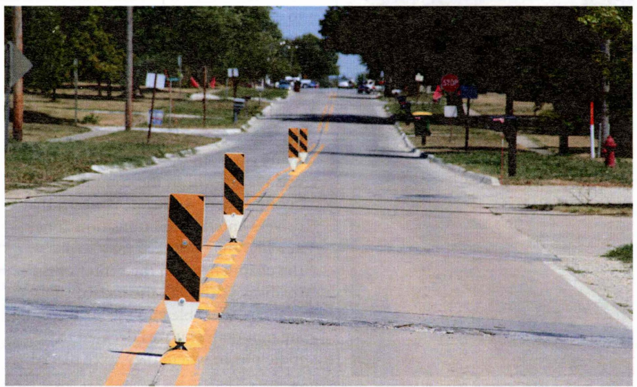
Mountable curbing at south entrance to St. Charles
