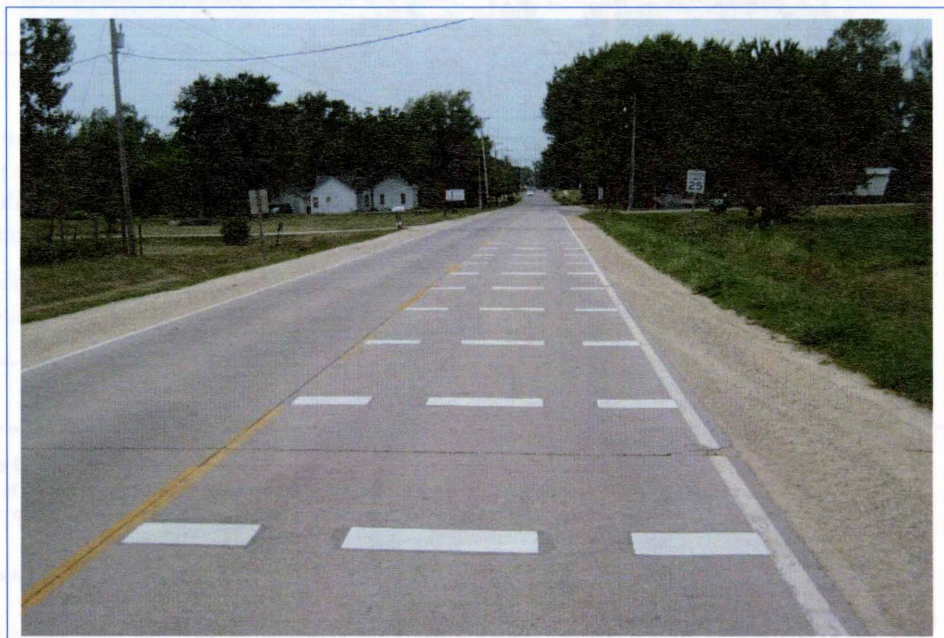
Transverse bar treatment at Hazleton east entrance
