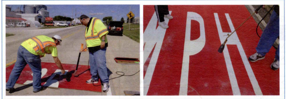
Installation of colored entrance treatment
