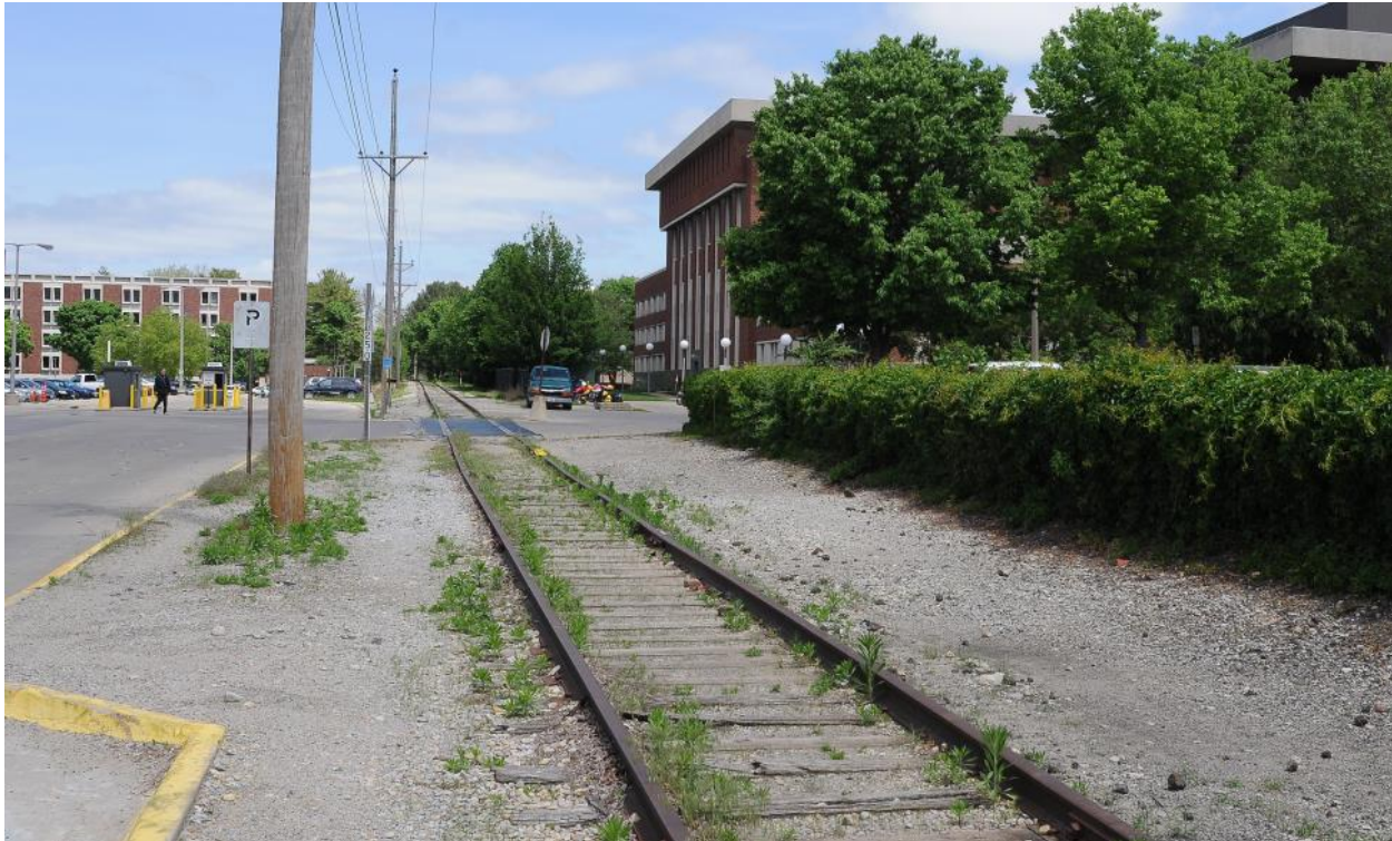
Figure 14. Typical Section of Narrow CRANDIC Corridor Right-of-Way in Urban Areas as Shown at Front Street in Iowa City
