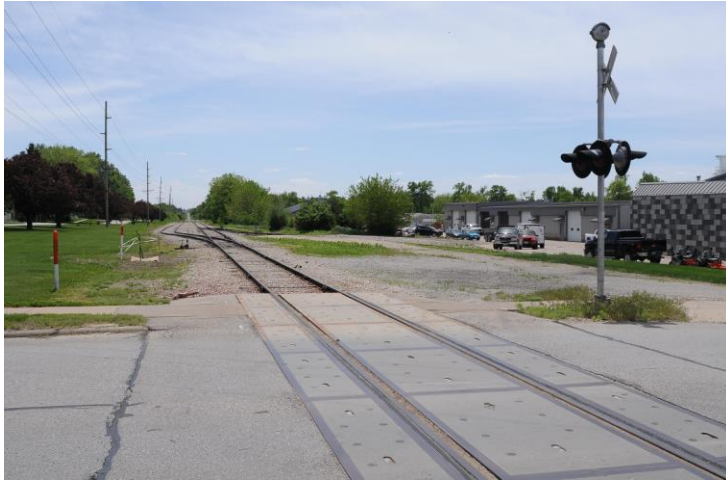
Figure 2. Typical CRANDIC Corridor Right-of-Way Usage
