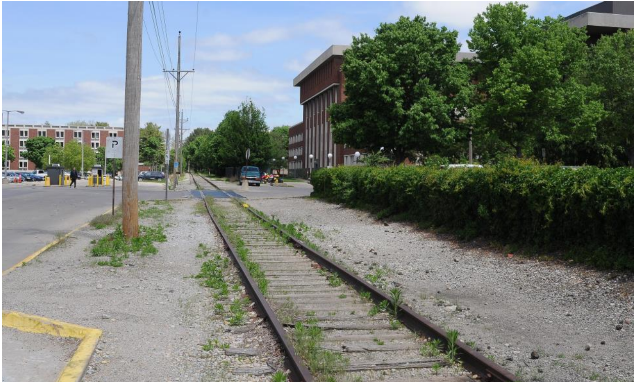
Figure 3. Typical Section of Narrow CRANDIC Corridor Right-of-Way in Urban Areas as Shown at Front Street in Iowa City
