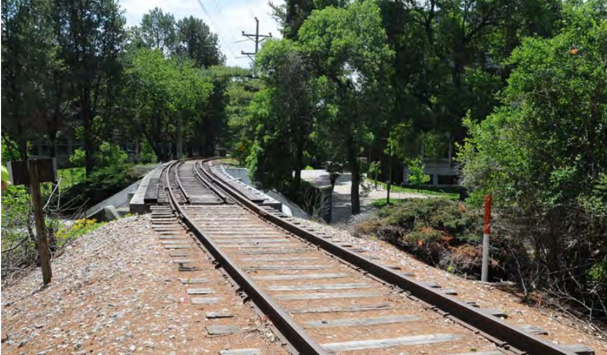
Figure 6 – Railroad Curvature and Grade in the CRANDIC Corridor Right-of-Way at Iowa Avenue in Iowa City
