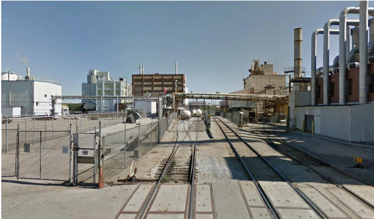
Figure 8. Typical Section of Constrained Active Freight Railroad Corridor as Shown on CRANDIC Line at 1st Street SW in Cedar Rapids
