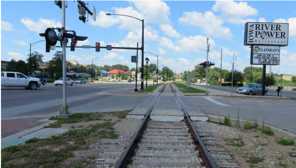
Figure 7 – Proximity of the CRANDIC Corridor Right-of-Way to Public Roadways at First Avenue in Coralville
