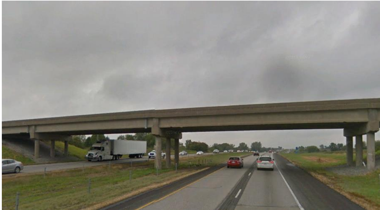
Figure 11. Typical Overpass in the Interstate 380 Corridor at Johnson County Highway F12 near Swisher
