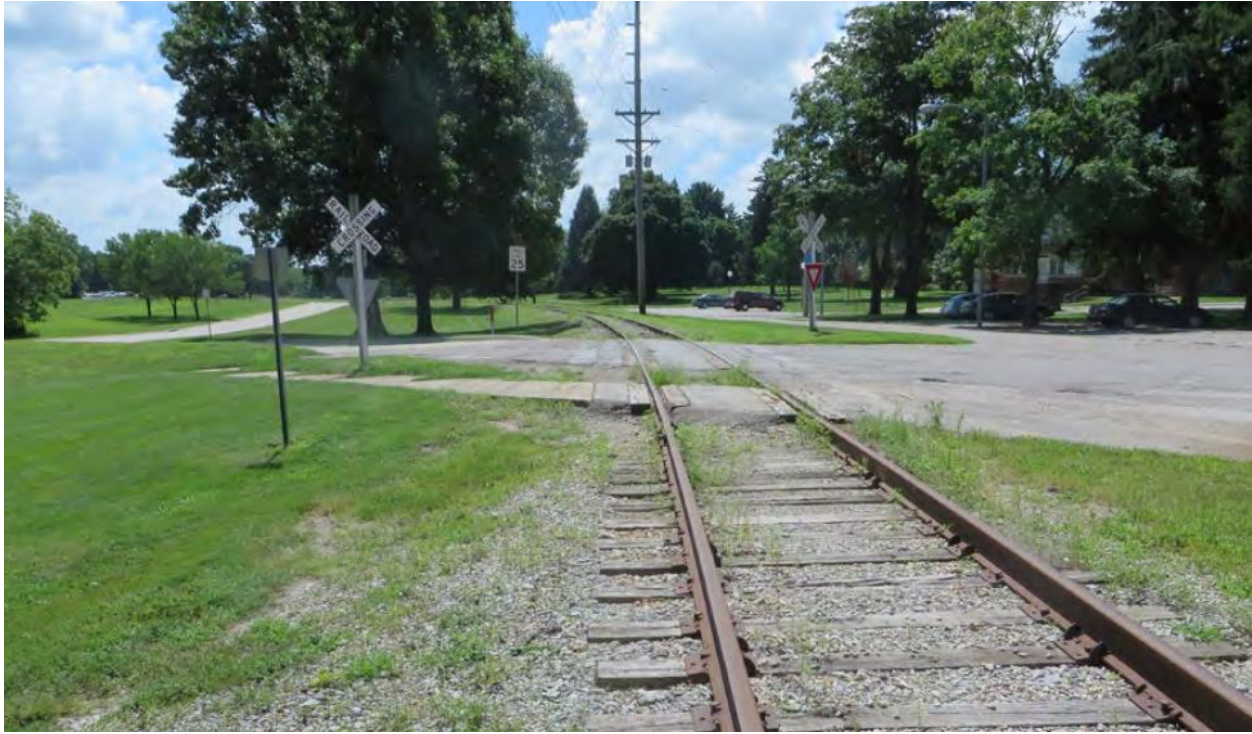
Figure 12 – Typical CRANDIC Corridor Passive Grade Crossing at Postal Road in Oakdale
