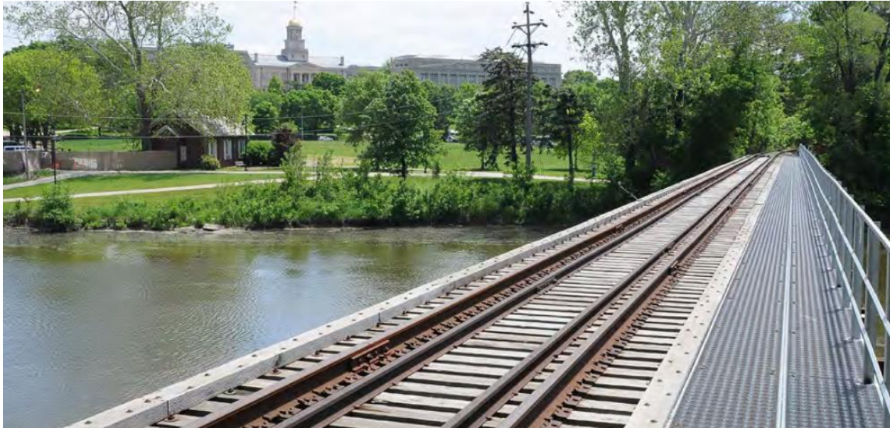
Figure 10 – Iowa River Bridge in Iowa City
