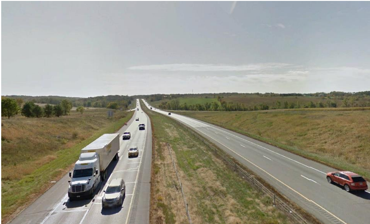
Figure 5. Typical Rural Section of Interstate 380 Corridor Right-of-Way with Four Lanes, Median, and Shoulders at Johnson County Highway F12 near Swisher
