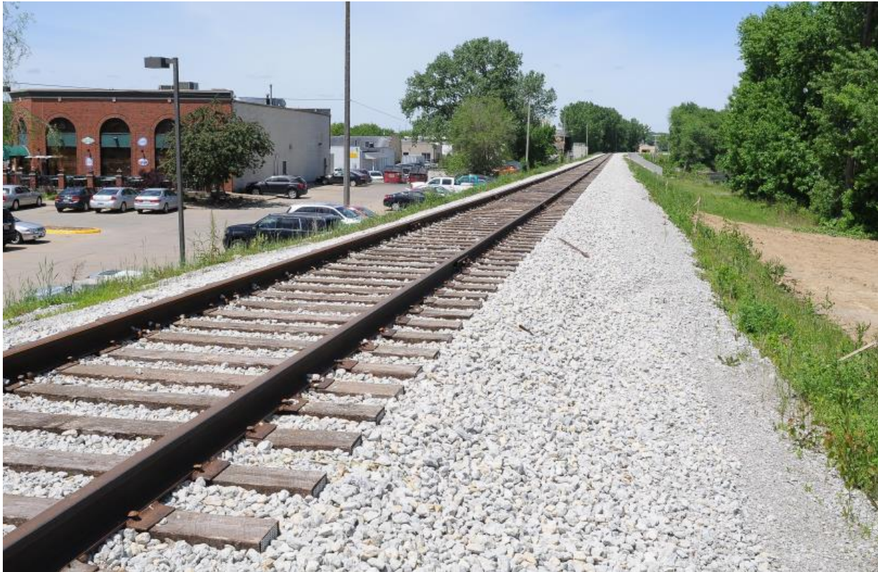
Figure 13. Typical Section of CRANDIC Corridor Right-of-Way at Rocky Shore Drive in Iowa City
