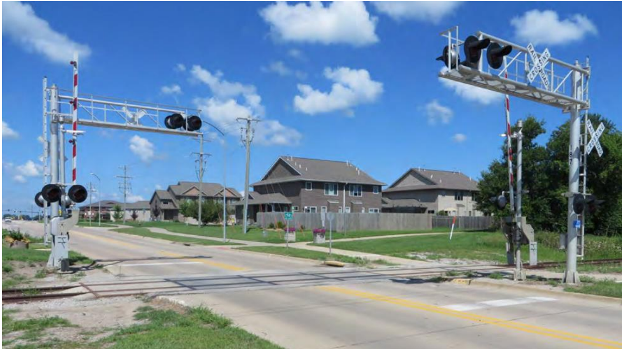
Figure 11 – Typical CRANDIC Corridor Active Grade Crossing at Forever Green Road in North Liberty
