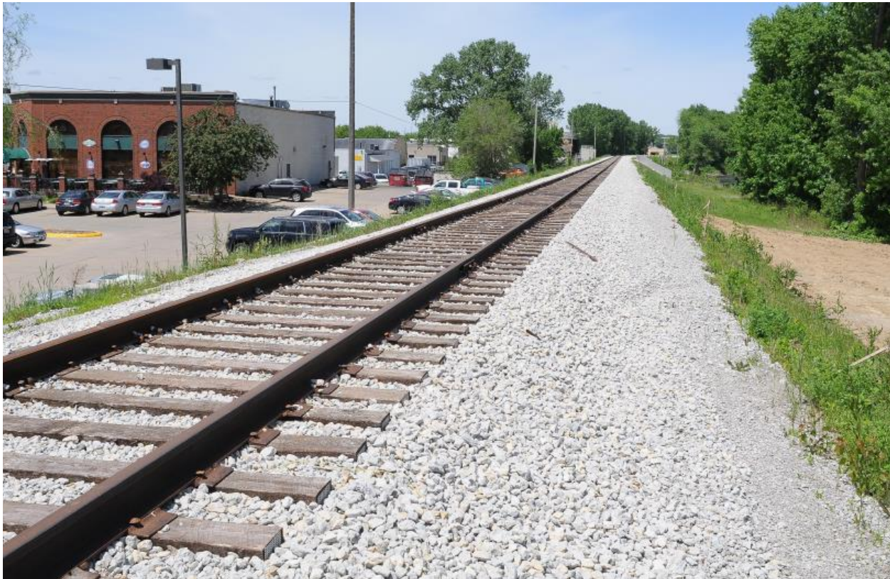
Figure 2. Typical Section of CRANDIC Corridor Right-of-Way at Rocky Shore Drive in Iowa City
