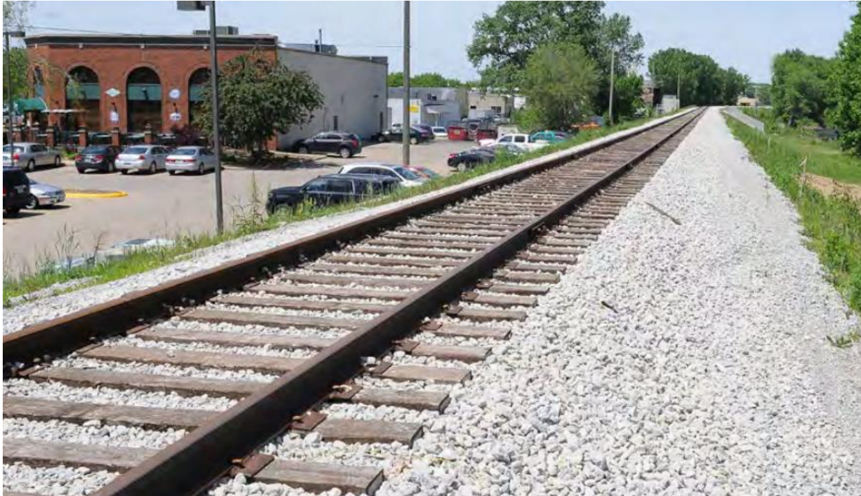
Figure 9 – CRANDIC Corridor Main Track Structure in Iowa City
