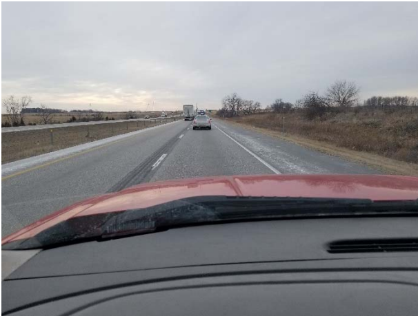
Photo 7. I-380 NEAR MP 3 (SNOW, BLIZZARD, HIGH TEMPERATURE CHANGE) – SOUTHBOUND LANES LOOKING SOUTH
