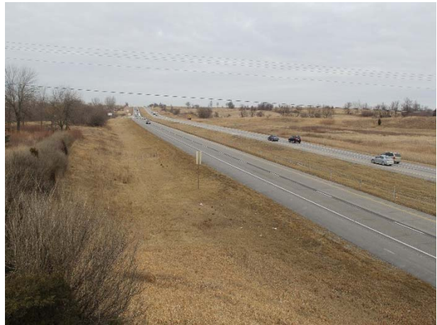
Photo 20. I-380 FROM COUNTY ROAD F-12 NEAR MP 11 (SNOW, BLIZZARD, HIGH TEMPERATURE CHANGE) – LOOKING NORTH FROM OVERPASS
