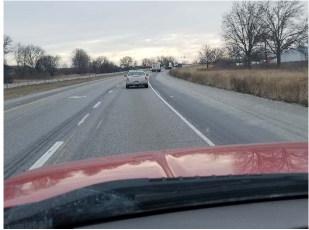
Photo 14. I-380 NEAR MP 7.5 (FLOODING, SNOW, BLIZZARD, HIGH TEMPERATURE CHANGE) – SOUTHBOUND LANES LOOKING SOUTH
