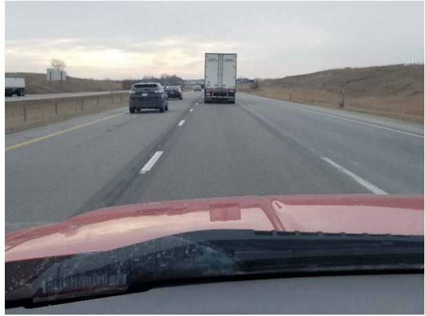
Photo 22. I-380 NEAR MP 13 (SNOW, BLIZZARD, HIGH TEMPERATURE CHANGE) – SOUTHBOUND LANES LOOKING SOUTH
