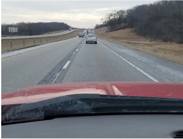
Photo 17. I-380 NEAR MP 10 (SNOW, BLIZZARD, HIGH TEMPERATURE CHANGE) – SOUTHBOUND LANES LOOKING SOUTH
