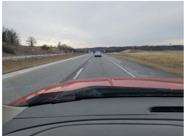
Photo 4. I-380 NEAR MP 2 (SNOW, BLIZZARD, HIGH TEMPERATURE CHANGE) – SOUTHBOUND LANES LOOKING SOUTH
