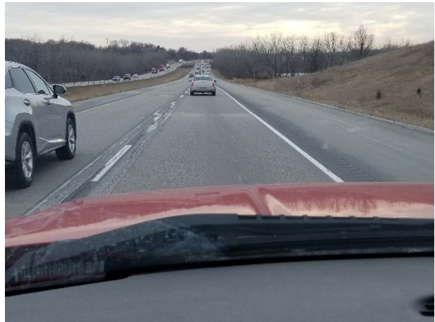
Photo 16. I-380 NEAR MP 8.5 (FLOODING, SNOW, BLIZZARD, HIGH TEMPERATURE CHANGE) – SOUTHBOUND LANES LOOKING SOUTH
