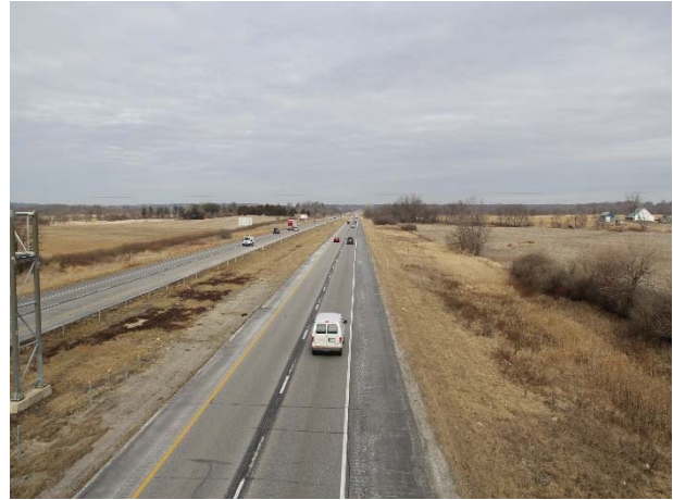
Photo 10. I-380 FROM SWAN LAKE ROAD (NEAR MP 5.5) (SNOW, BLIZZARD, HIGH TEMPERATURE CHANGE) – LOOKING NORTH FROM OVERPASS
