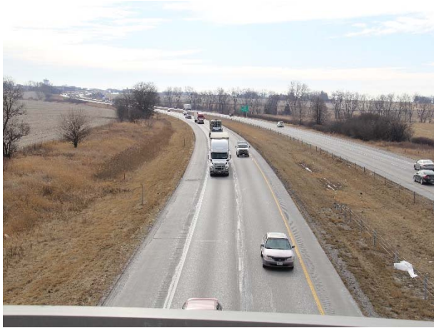
Photo 9. I-380 FROM SWAN LAKE ROAD (NEAR MP 5.5) (SNOW, BLIZZARD, HIGH TEMPERATURE CHANGE) – LOOKING SOUTH FROM OVERPASS
