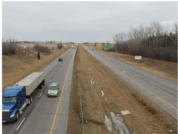
Photo 24. I-380 FROM WRIGHT BROTHERS BLVD. NEAR MP 14 (SNOW, BLIZZARD, HIGH TEMPERATURE CHANGE) – LOOKING NORTH FROM OVERPASS
