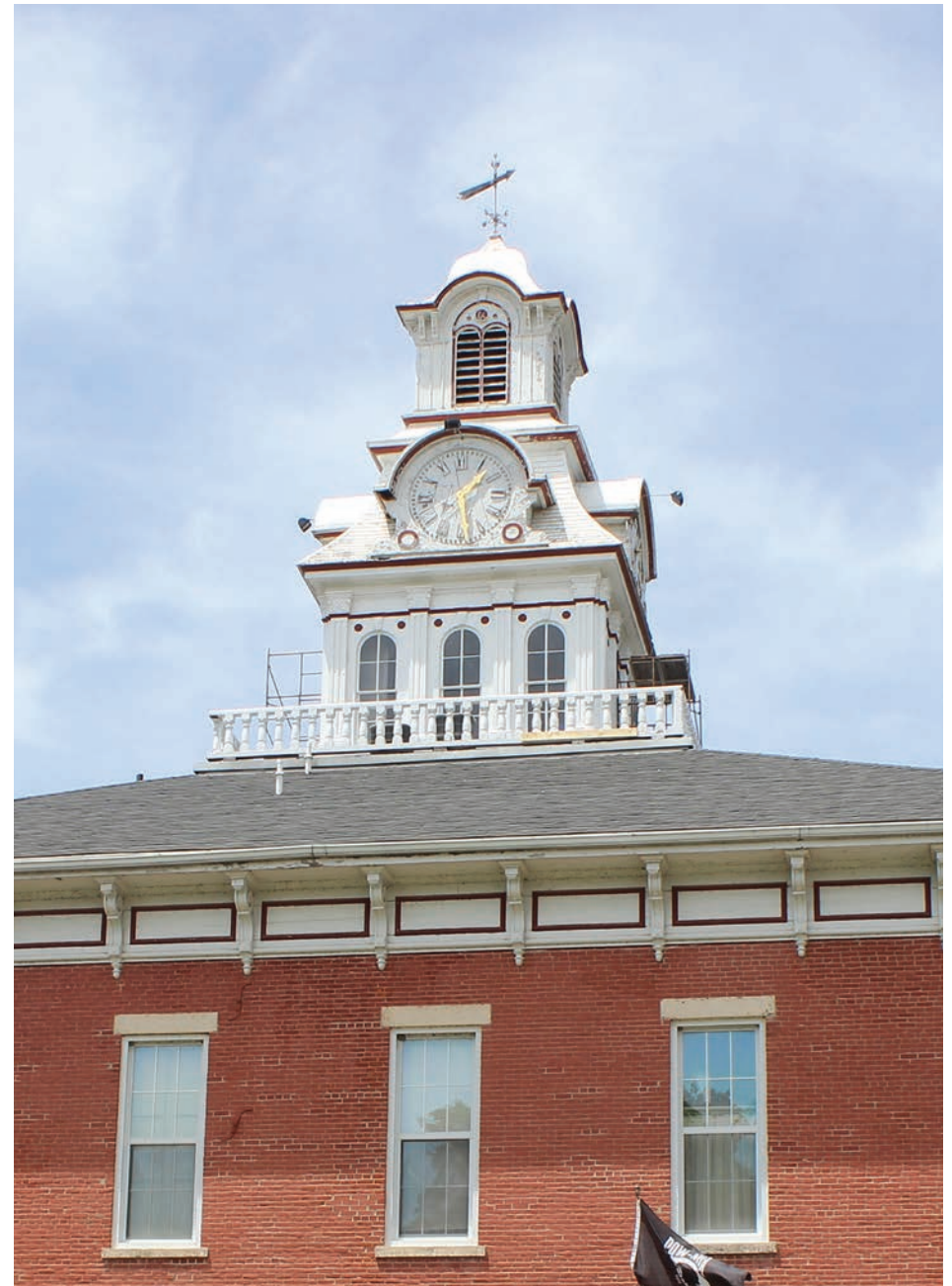
Clayton County Courthouse & Clock Tower Restoration
