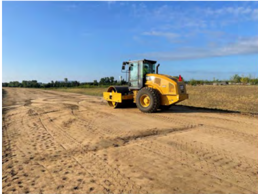
Figure 29. Photo of mapping on Subgrade (Sand) on I-380 Ramp C.
