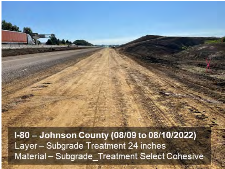
Figure 6. I-80, Subgrade Treatment 24 inches, Subgrade_Treatment Select Cohesive.
