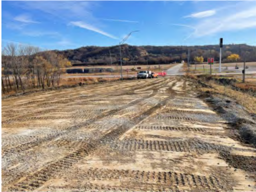
Figure 49. Photo showing east side approach embankment on G12.
