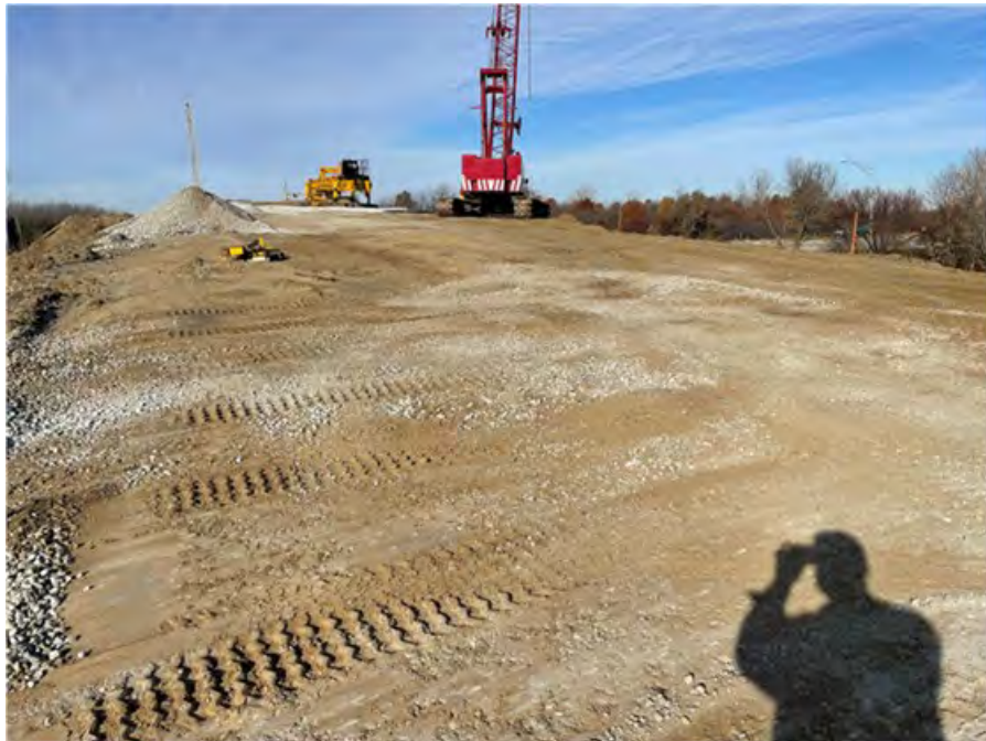
Figure 50. Photo showing east side approach embankment on G12.
