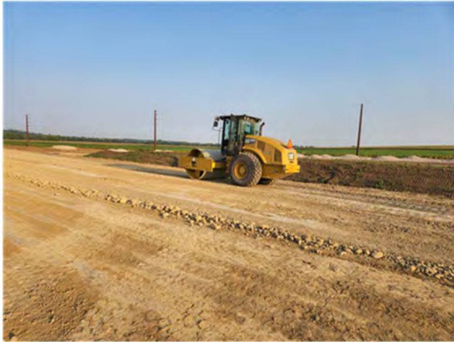
Figure 37. Photo of US 30 Top of 24 Inch Select Soil Subgrade Treatment.
