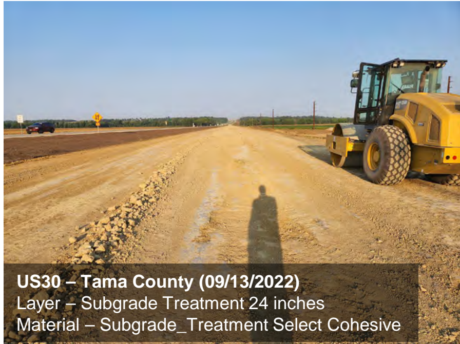
Figure 9. US30, Subgrade Treatment 24 inches, Subgrade_Treatment Select Cohesive.
