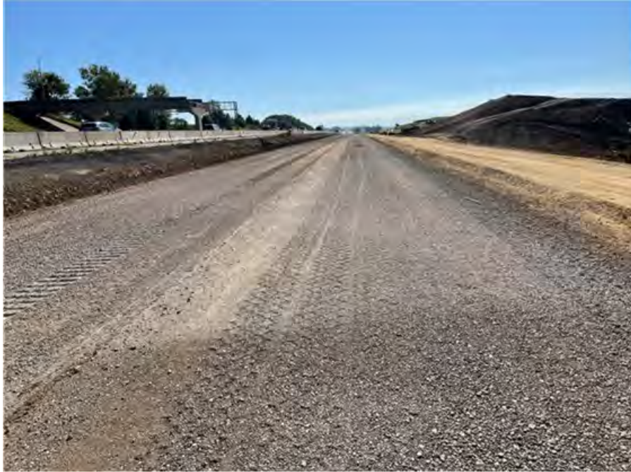
Figure 23. Photo Top of 6 Inch Granular Subbase Recycled PCC.
