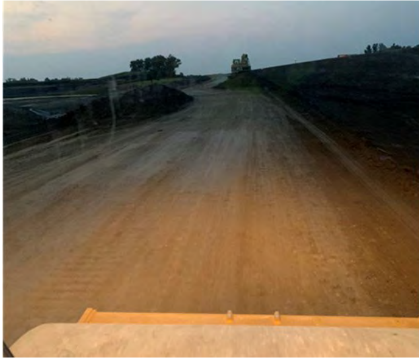
Figure 43. Photo showing mapping of Subgrade Class 10 (Clay) on Ramp C.
