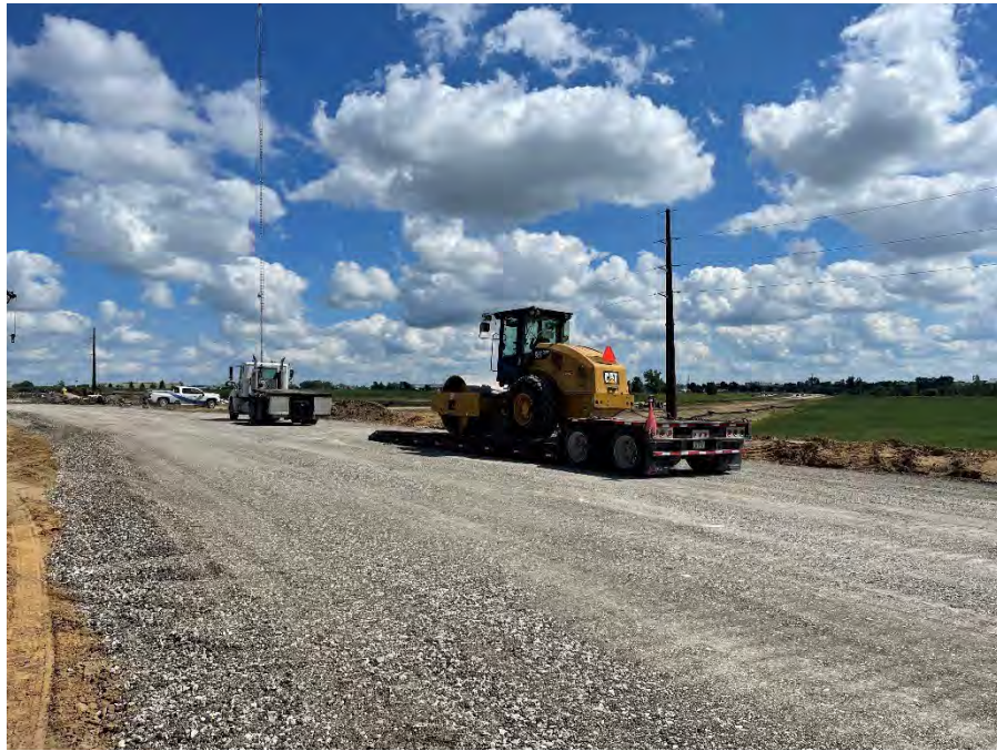
Figure 3. Instrumented roller mobilized to project sites.
