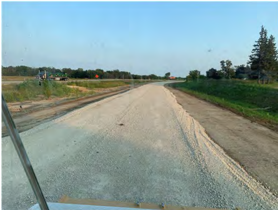
Figure 44. Photo showing mapping of Modified Subbase Recycled PCC on Eastbound Mainline.
