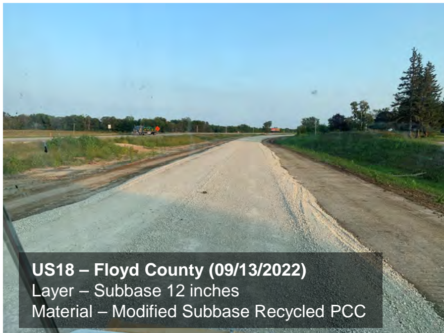
Figure 10. US18, Subbase 12 inches, Modified Subbase Recycled PCC.
