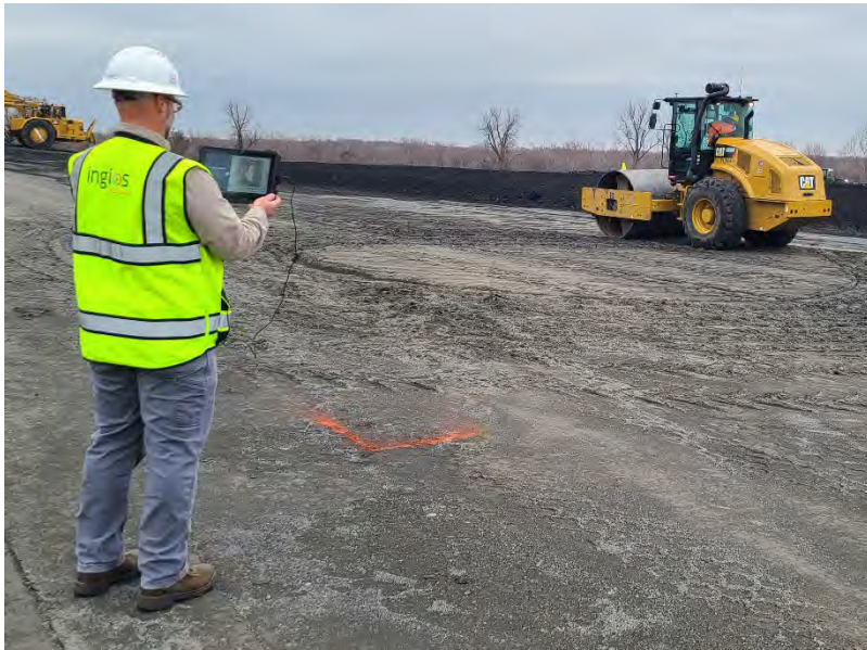
Figure 16. Inspector viewing Comp-Score(R) e-Compaction report using INSPECTOR application.
