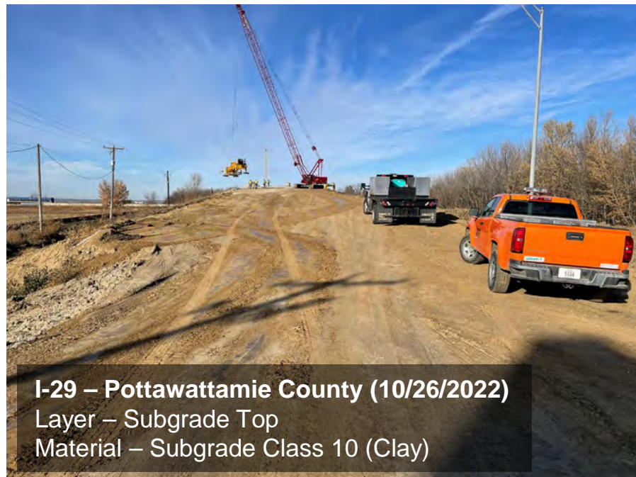
Figure 12. I-29, Subgrade Top, Subgrade Class 10 (Clay).
