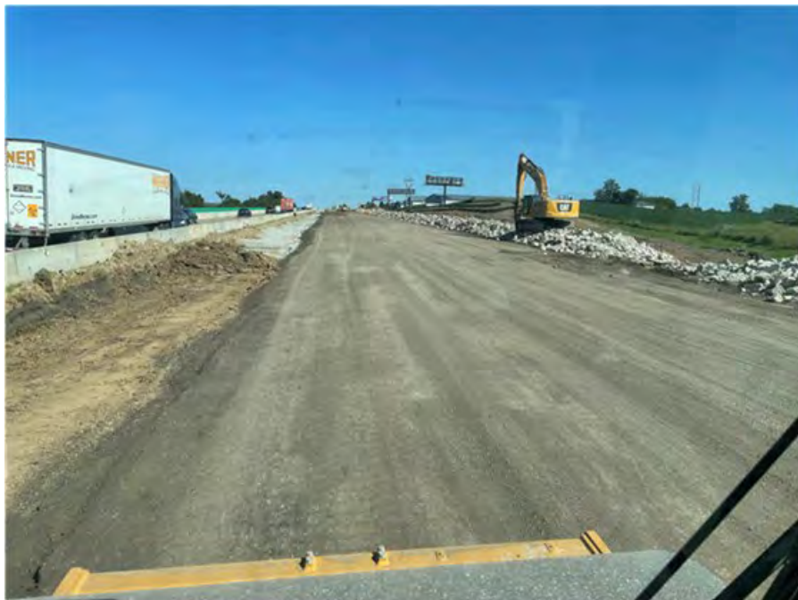
Figure 22. Photo I-80 Top of 12 Inch Special Backfill RAP Subgrade Treatment.
