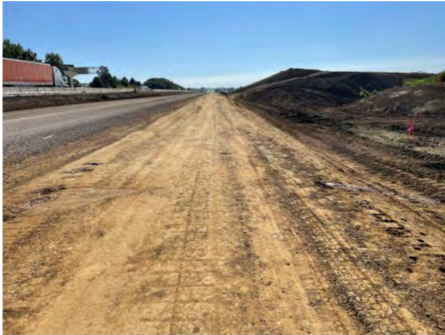
Figure 21. Photo I-80 Top of 24 Inch Select Soil Subgrade Treatment.
