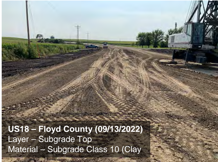
Figure 11. US18, Subgrade Top, Subgrade Class 10 (Clay).
