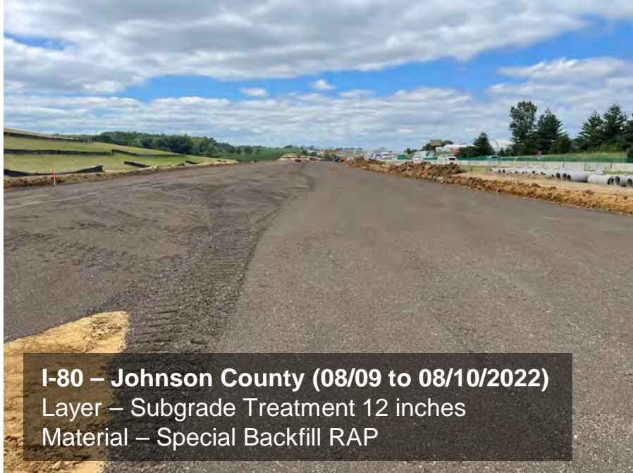
Figure 5. I-80, Subgrade Treatment 12 inches, Special Backfill RAP.
