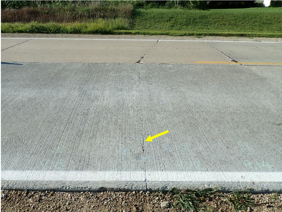
Figure 6.16. Patch No. 5 typical condition. No cracks observed. Transverse joint in good condition with very minor raveling (Yellow arrow).
