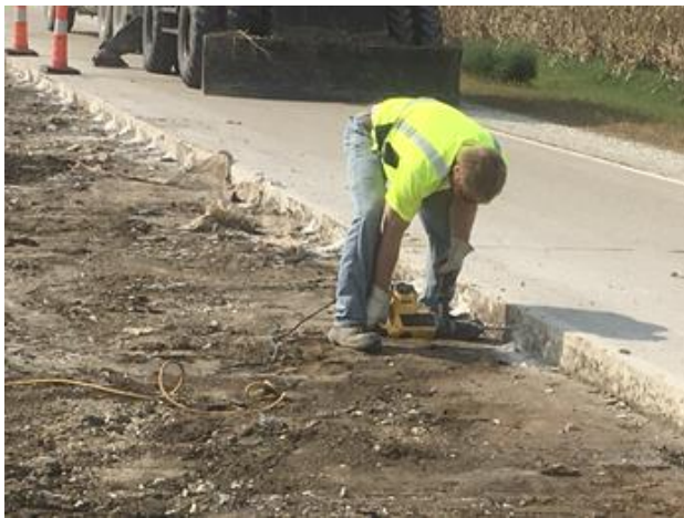
Figure 5.3. Tie bar hole drilling (Patch 2).
