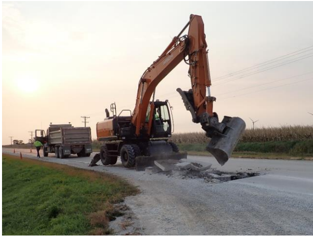
Figure 5.1. Concrete breaking and removal (Patch 1).
