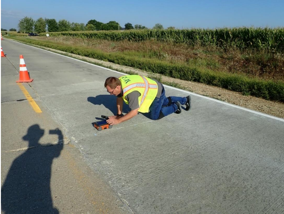
Figure 6.2. Locating dowels at transverse joints using GPR.
