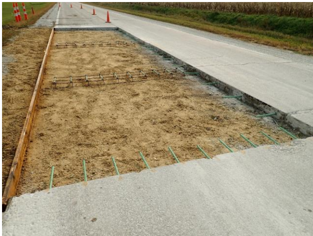
Figure 5.7. Tie bars, dowels and dowel baskets installed (Patch 1)
