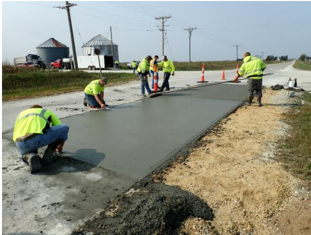
Figure 5.9. Concrete finishing (Patch 1)
