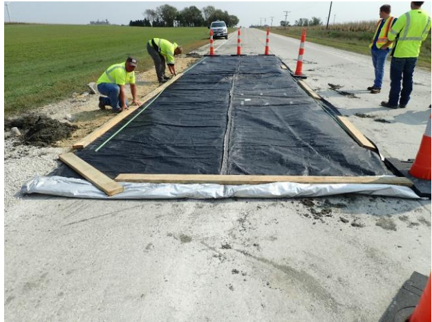
Figure 5.10. Concrete curing with insulation blanket (Patch 1)
