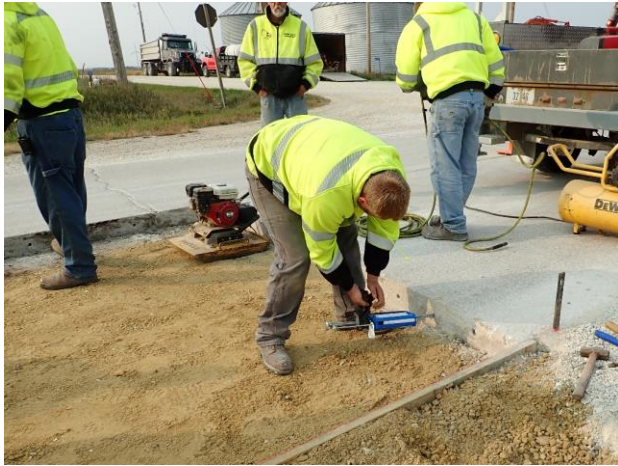
Figure 5.5. Filling hole with epoxy (Patch 1)
