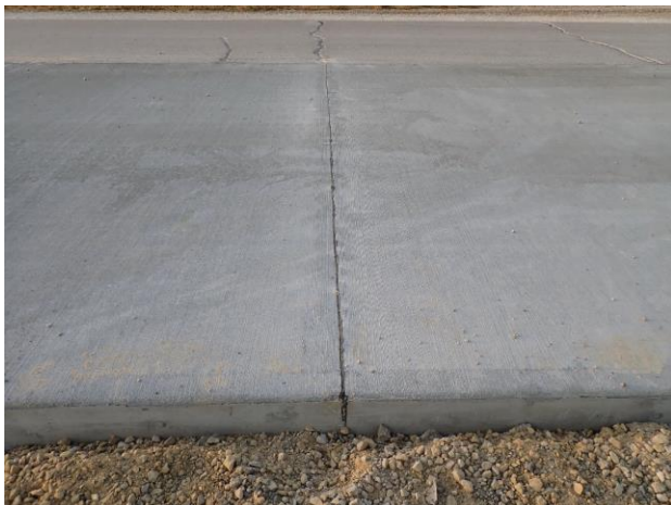
Figure 5.11. Cut and sealed transverse joint (Patch 1)
