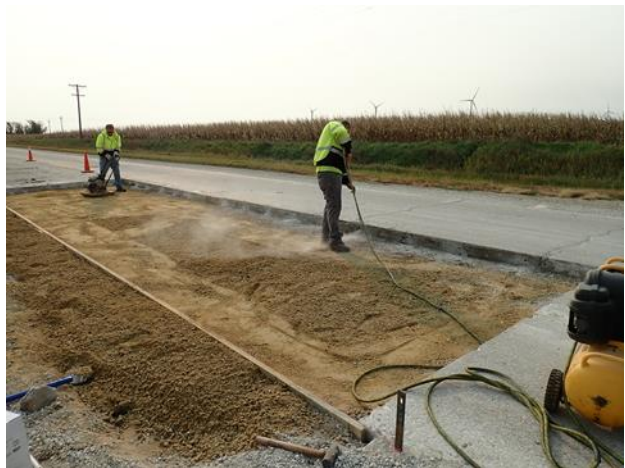
Figure 5.4. Hole cleaning using compressed air (Patch 1).
