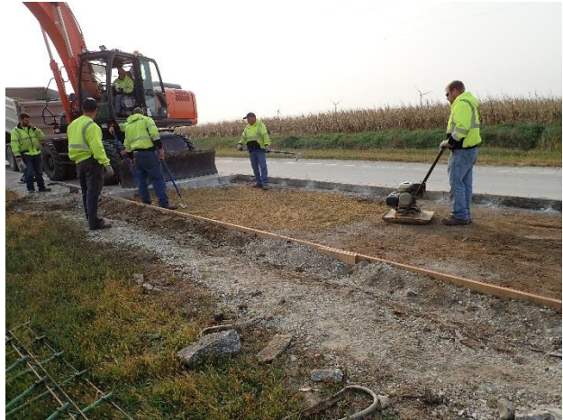
Figure 5.2. Subbase preparation (Patch 1).
