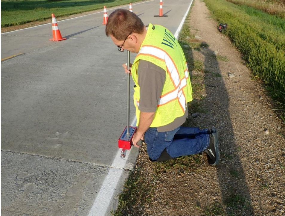
Figure 6.1. Elevation measurements using a floor profiler.
