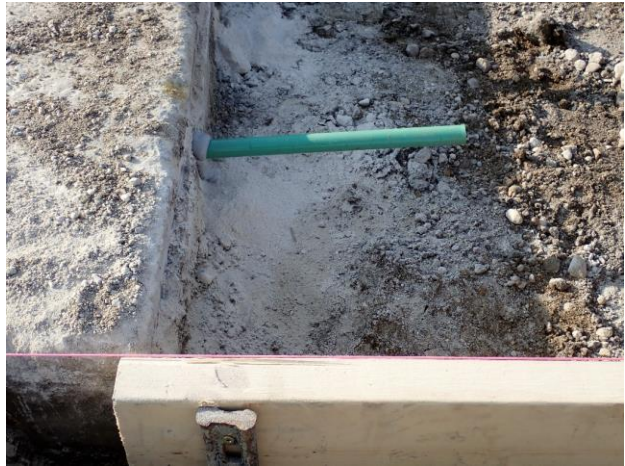
Figure 5.6. Inserted dowel
