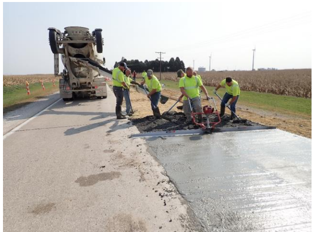
Figure 5.8. Concrete placement and screeding (Patch 2)
