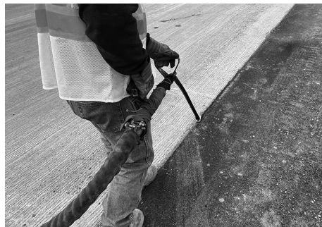
Sealing of a longitudinal joint ( Scott Eilken, Quality Saw & Seal, Inc. )
