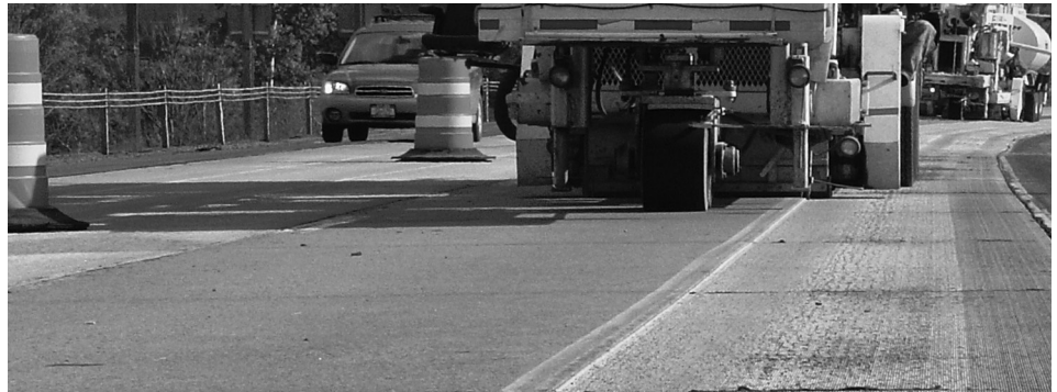
Concrete pavement diamond grinding ( International Grooving and Grinding Association )
