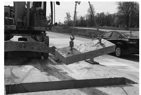
Chain lift-out method of slab removal ( John Donahue, MoDOT )
