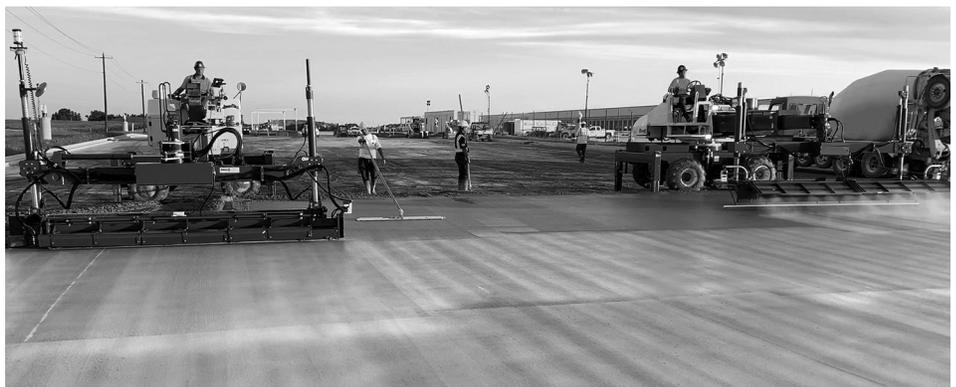
Placement using a laser-guided screed, with the screed on the left and the texturing and curing equipment on the right (Michael Hoeft, K & M Concrete Construction, Inc.)
