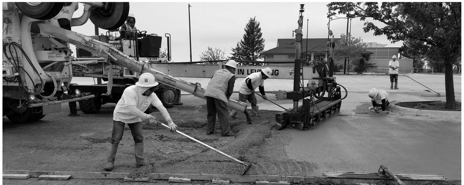
Active concrete pavement construction site on a parking lot showing several crew members working on various stages of the concrete overlay paving operation (City of Thornton, Colorado)
