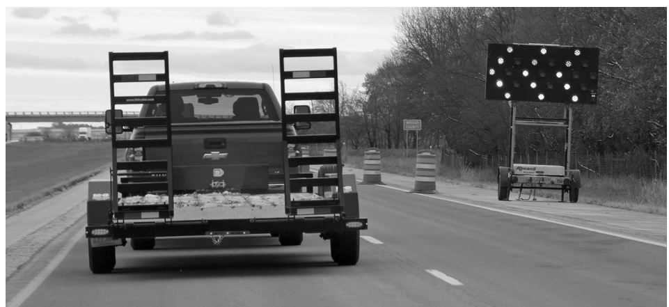
Smart arrow board at the beginning of a work zone in Iowa
