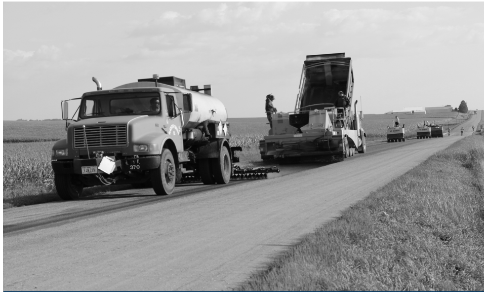
Otta seal construction process: binder spraying, aggregate application, and rolling compaction
