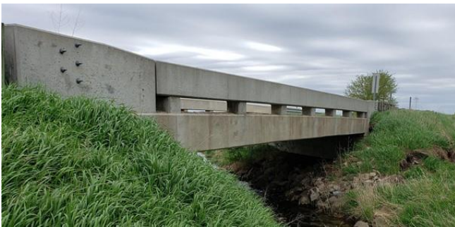
Figure 1. An example of a single span concrete slab bridge.
