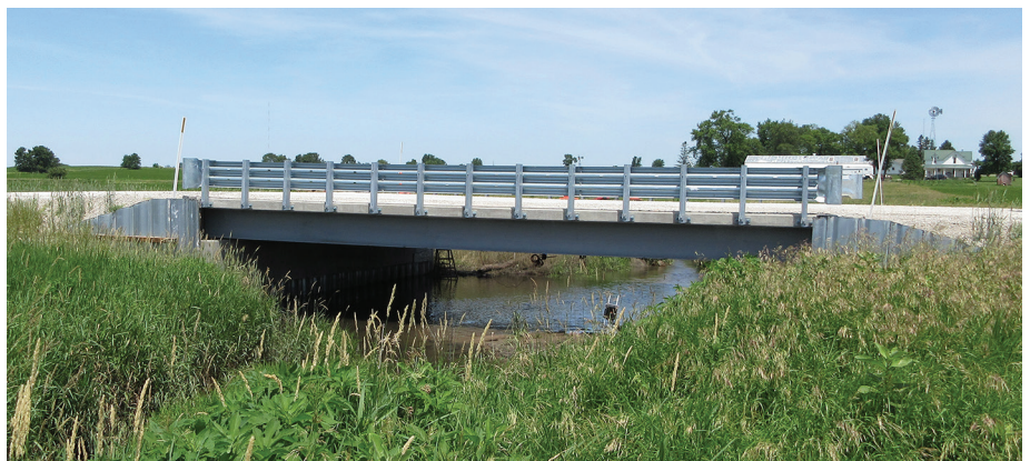
First bridge project in the US utilizing A709 Grade QST 65 steel: Buchanan County Sand Creek Bridge
