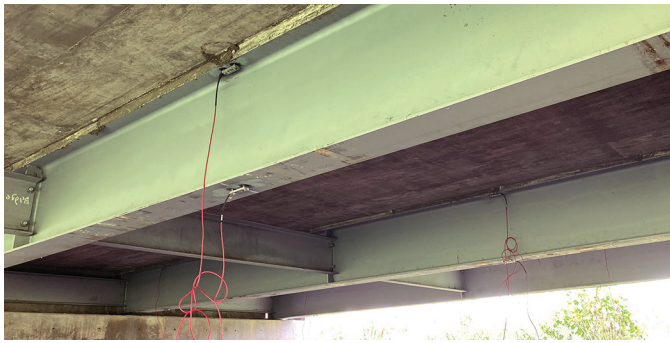
Sand Creek Bridge strain gauges at midspan
