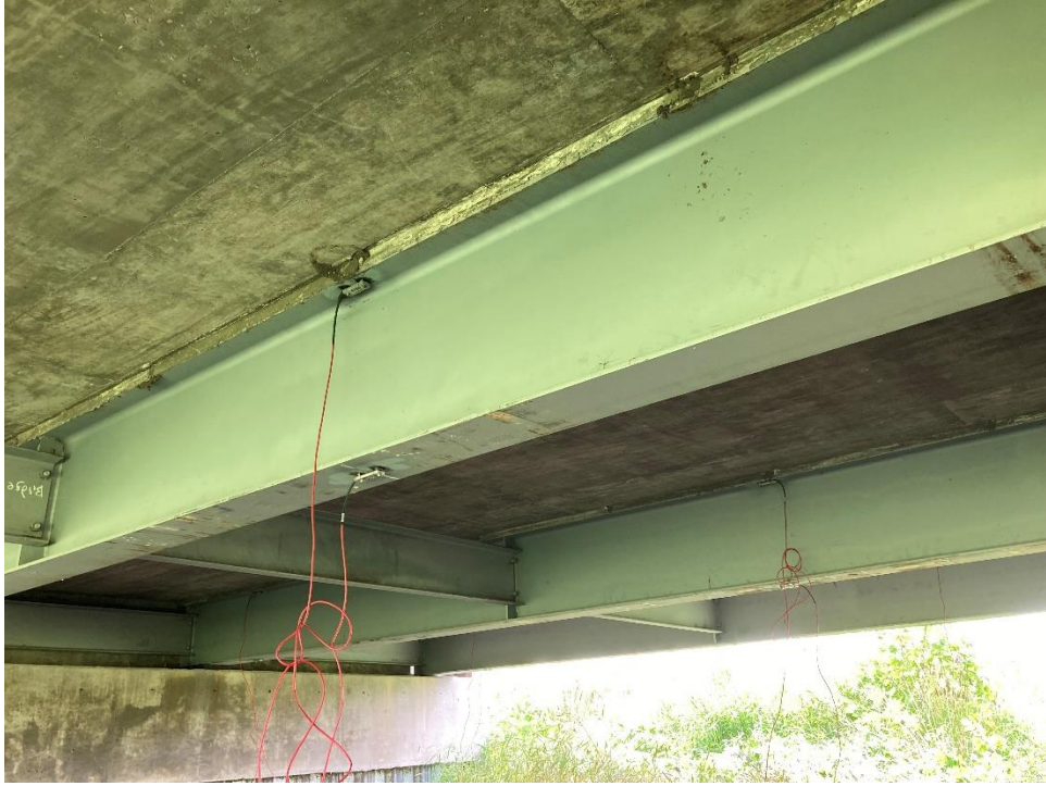
Figure 51. Strain gauges at midspan
