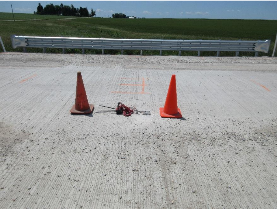
Figure 53. Deck strain gauges
