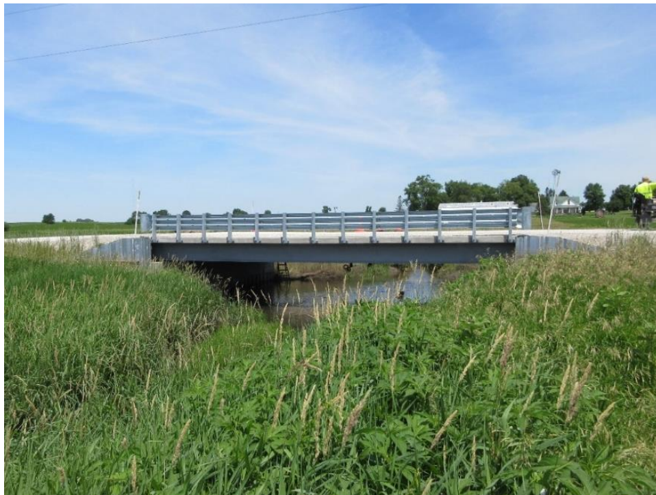
Figure 40. Buchanan County Sand Creek Bridge
