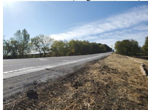
Road Above Culvert (September 30, 2020)
