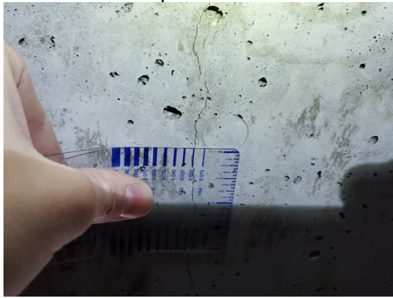
c. Crack gauge
