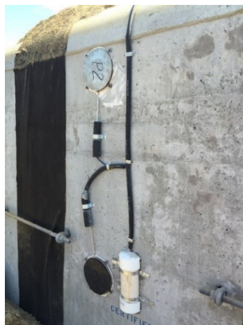
a) Strain and earth pressure gauges
