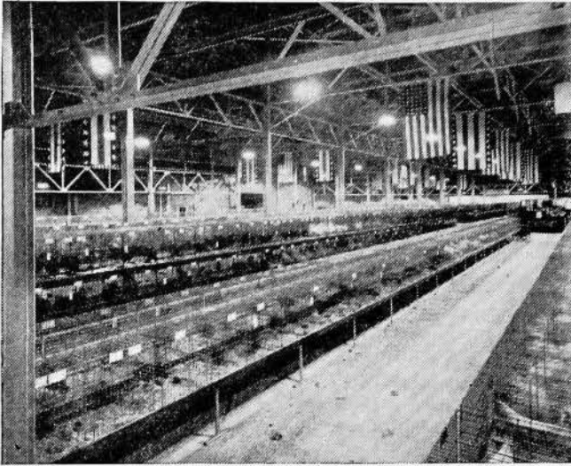
A partial view of the interior of the Iowa State Fair Poultry Building. It will accommodate more than 6,000 birds on exhibition, but State Fair entries were so large last year that some of the entries had to be placed in open-air pens.
