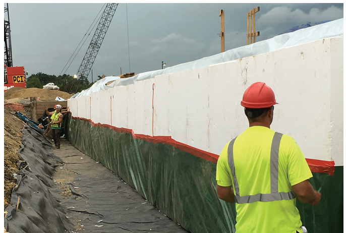
Installation of EPS isolation barrier
