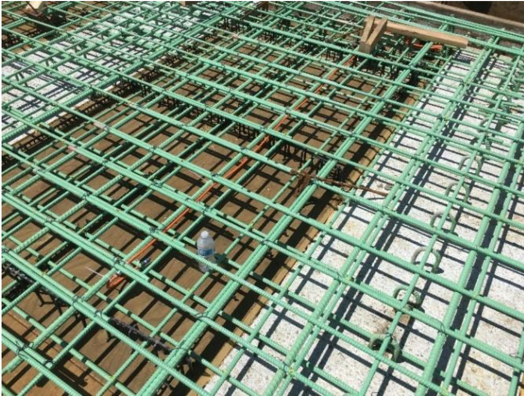
Figure 16. Thermistor placement along deck reinforcement
