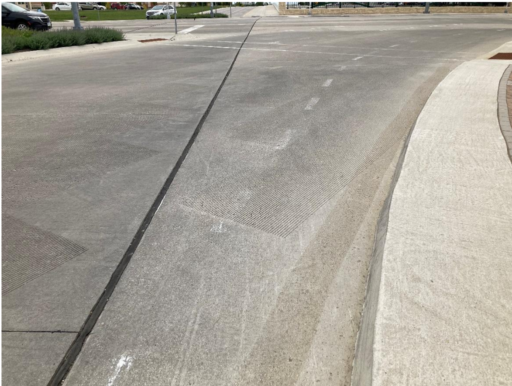
Figure 35. Deck inspection May 2022 East abutment
