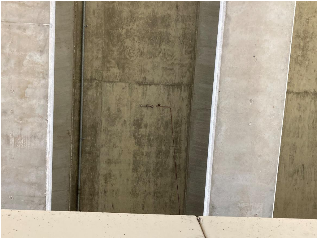
Figure 41. Deck inspection May 2022 Bay PQ
