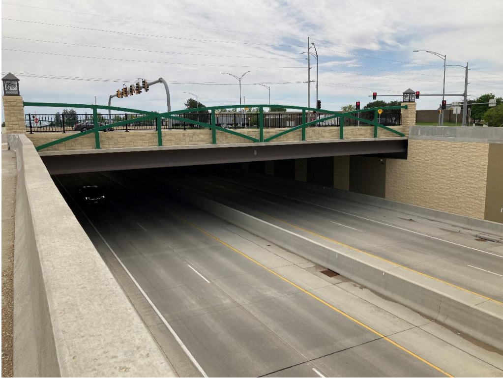
Figure 1. Viking Road Bridge over IA 58
