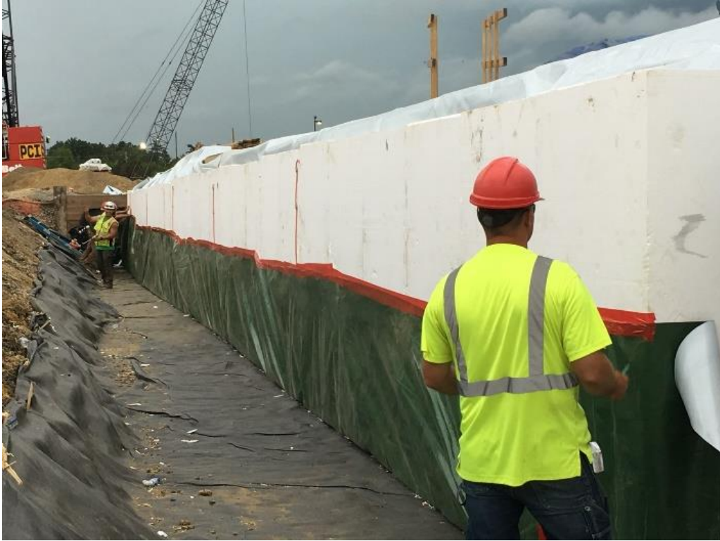
Figure 8. Installation of EPS isolation barrier
