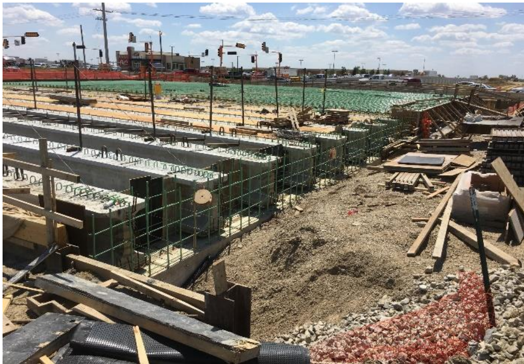
Figure 13. Prestressed girder placement
