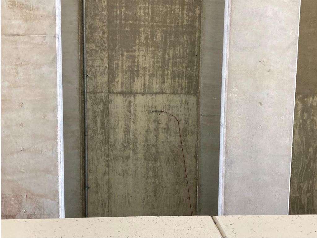
Figure 40. Deck inspection May 2022 Bay MN
