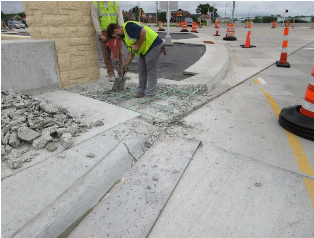
Figure 45. Raised island repair at southeast corner
