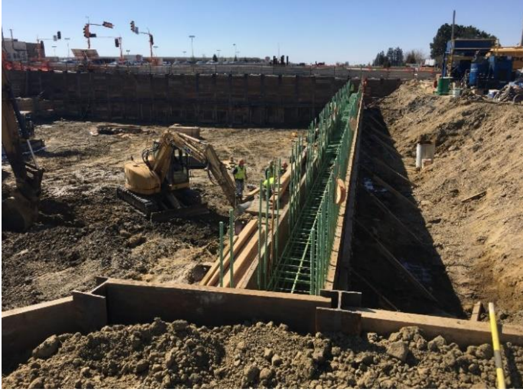
Figure 17. Abutment formwork
