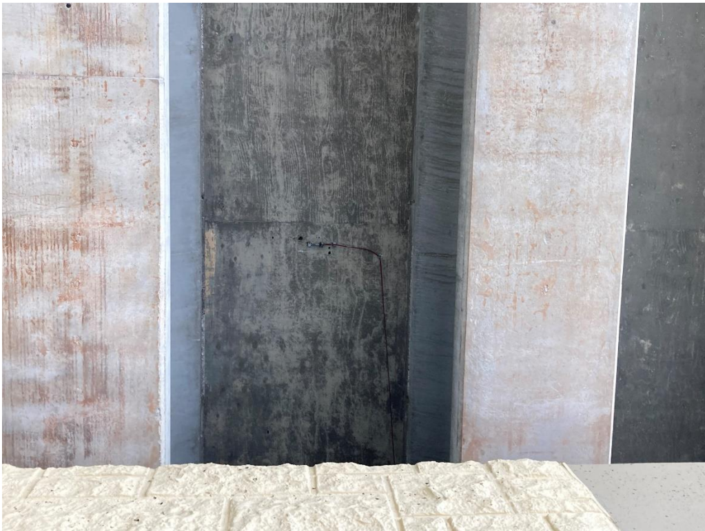
Figure 37. Deck inspection May 2022 Bay DE
