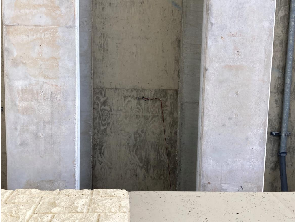
Figure 38. Deck inspection May 2022 Bay GH
