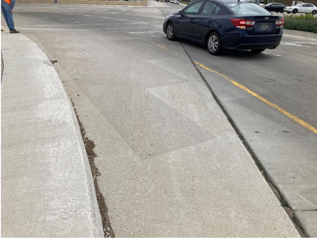
Figure 34. Deck inspection May 2022 West abutment
