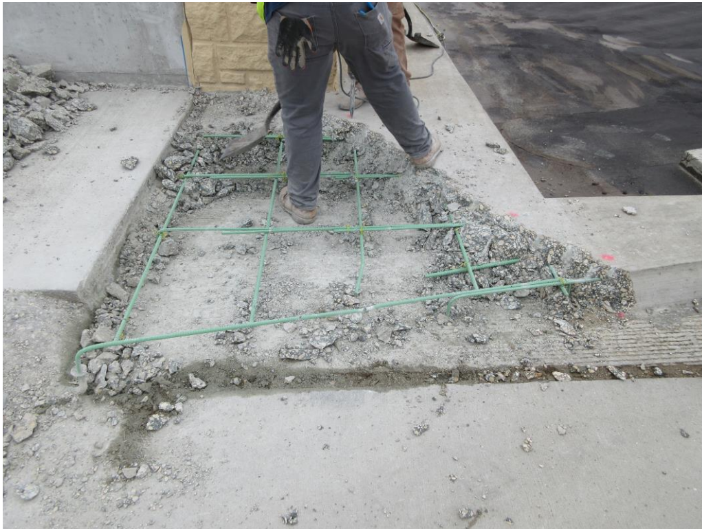
Figure 46. Raised island repair
