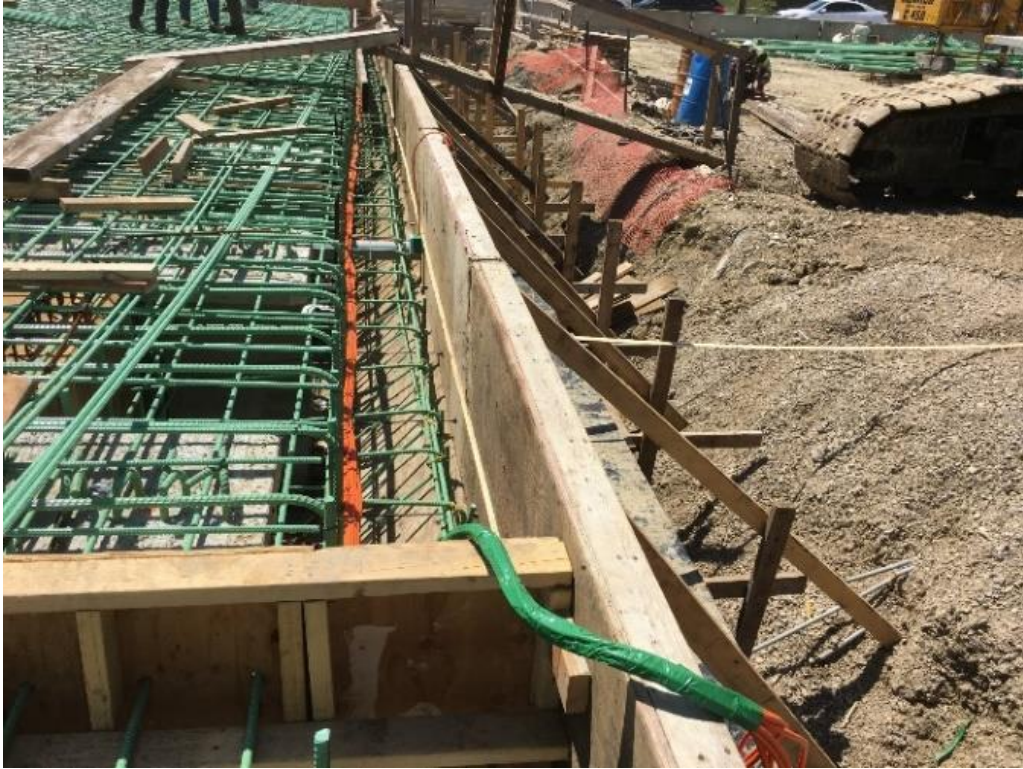
Figure 14. Thermistor wires placed in abutment formwork
