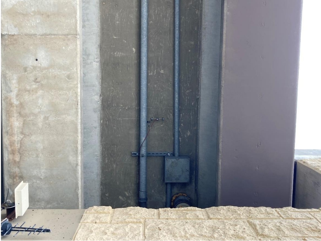
Figure 36. Deck inspection May 2022 Bay AB
