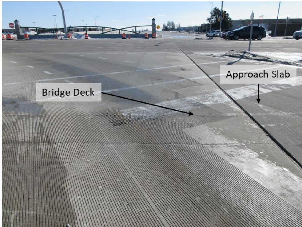
Figure 9. Deck end at West abutment
