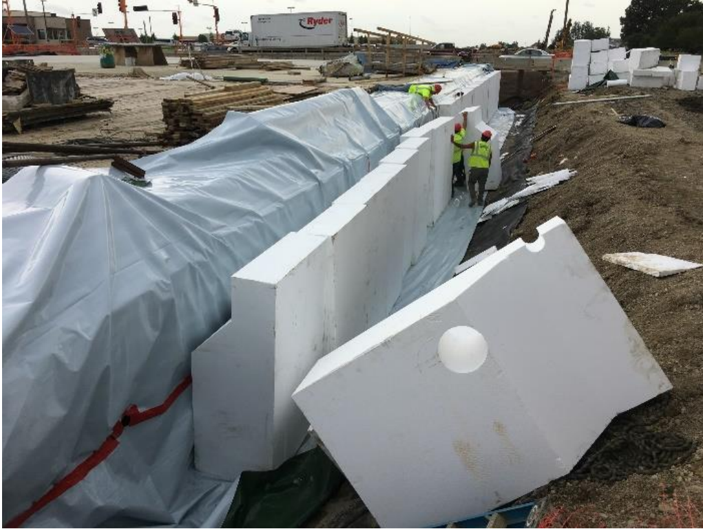
Figure 7. Preparing for placement of EPS isolation barrier
