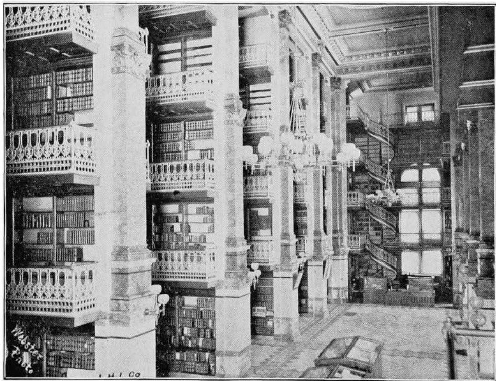
INTERIOR VIEW OF STATE LIBRARY—FROM NORTH GALLERY.
