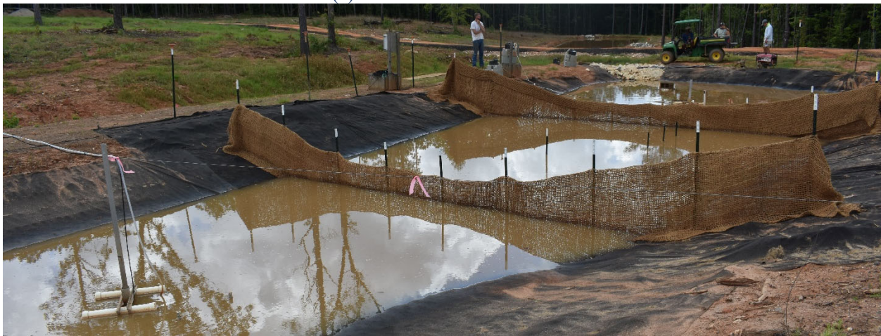
(b) coir baffles during flow
