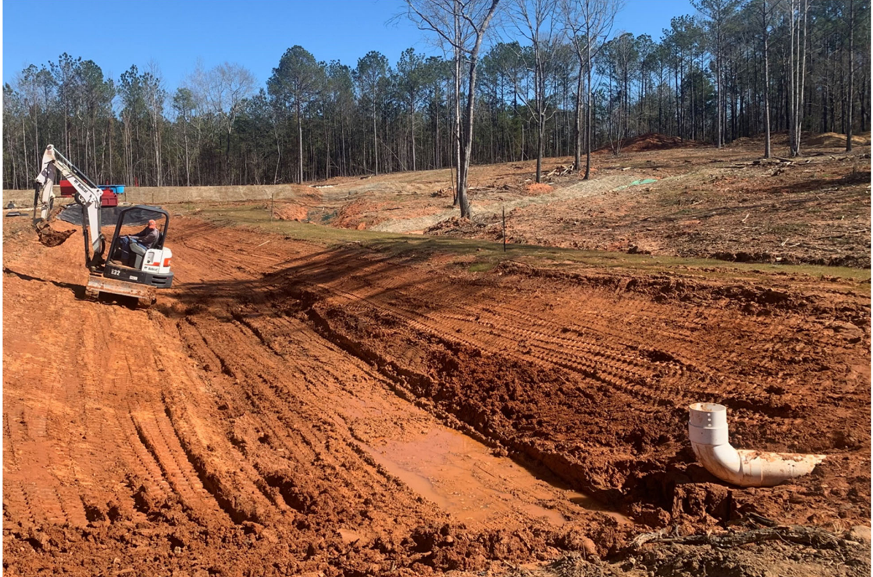
(a) channel grading
