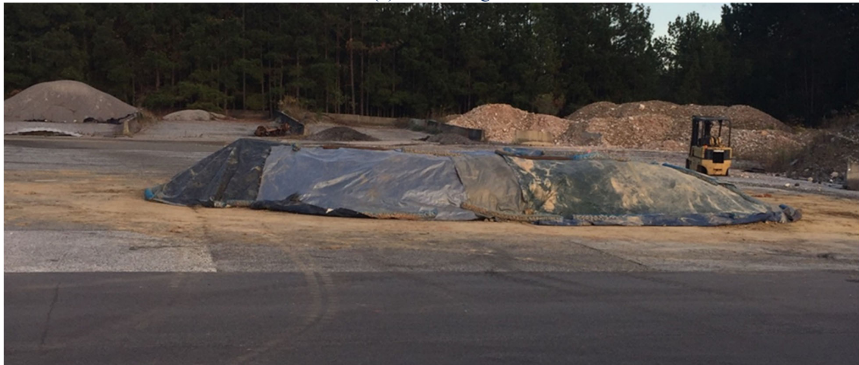
(b) compacted and covered stockpile
