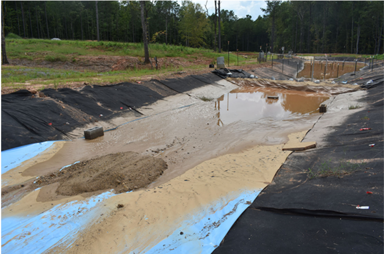
Figure 3.28. In-channel sedimentation due to forebay installation.
