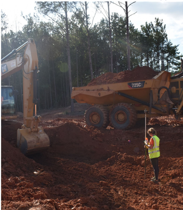
(b) excavating basin and surveying grade
