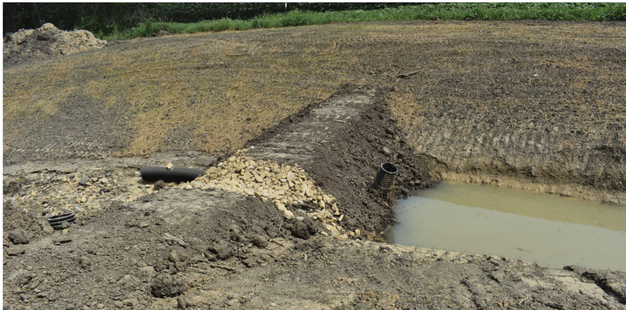
(a) Iowa DOT sediment basin installation
