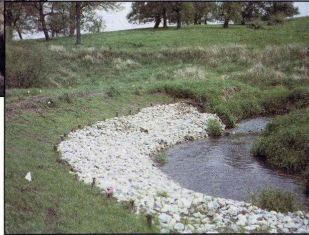
After streambank stabilization
