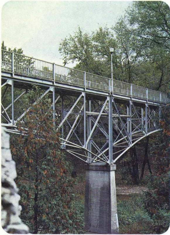
Meredith Wilson footbridge
