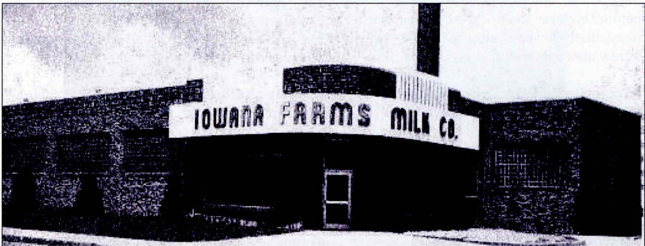
Figure 8. Historical elevation view of the original Iowana Farms Milk Co. plant in 1938. “The entrance doorway is on the corner. It is surmounted by a large neon sign which proclaims to the world ‘Iowana Farms Milk Company.’ Passing through this attractive portal brings the visitor into the salesroom.” /
