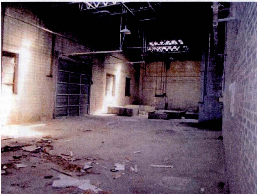
Figure 5. Part of the c.1950-52 Ice Cream Factory addition, Room D-3. Features the smokestack base (bump-out, center right), boiler room access (not shown, but further back on right-side wall on either side of smokestack base), glazed tile walls, two wired-glass skylights, and remnants of concrete machine platforms (toward rear of room). View is to NW / Photo by Tallgrass Historians L.C., September 2010
