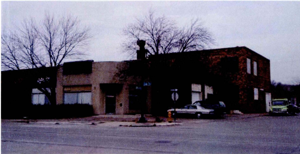
Figure 4. View of the Iowana building to the NW. Shows the SE entrance and two-story addition.
