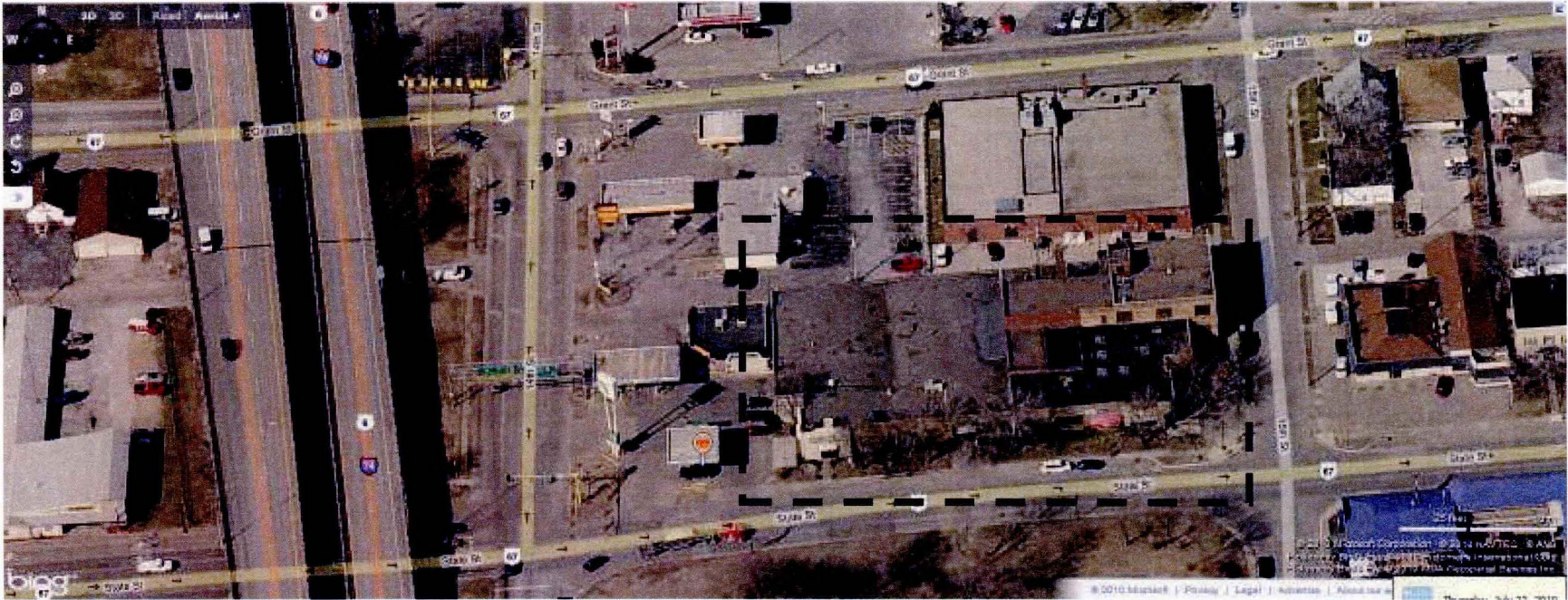
Bird's eye aerial view of the Iowa Farms Milk Co. plant building prior to demolition, 2010. View is to North.
