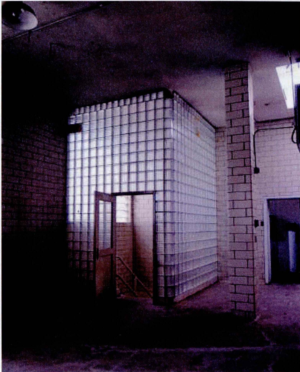
Figure 7. Glass-block-enclosed stairwell, Room D-4, Second Floor, Ice Cream Factory. This room also features glazed tile walls, service elevator access, and a wired-glass skylight (upper right). View to East.
