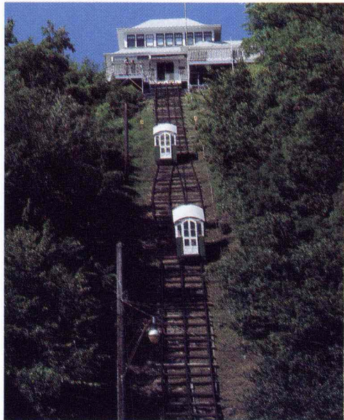
Fenelon Place Elevator (#47)
