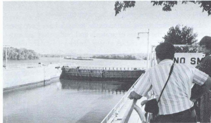
Guttenburg Lock and Dam #10
