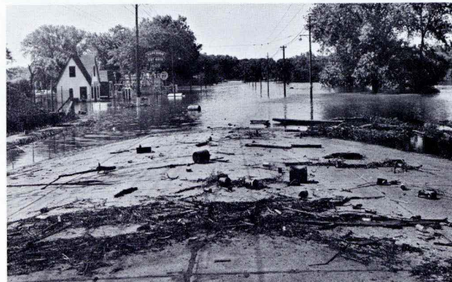
Looking south on Sixth Avenue from New York Avenue — June 26, 1947 flood.
