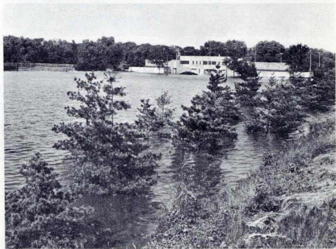
Looking west from Second Avenue at the swimming pool and playground near Franklin Avenue—June 24, 1954 flood.
