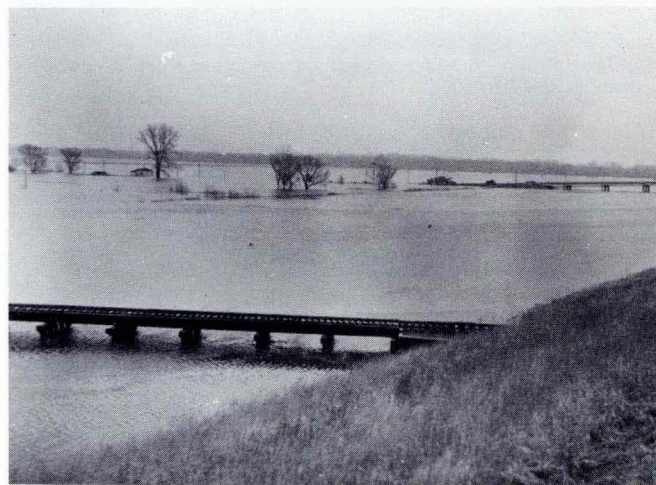
Looking northeast at the D.M. & C.I. R.R. and Beaver road bridges over Beaver Creek — April 10, 1965 flood.
