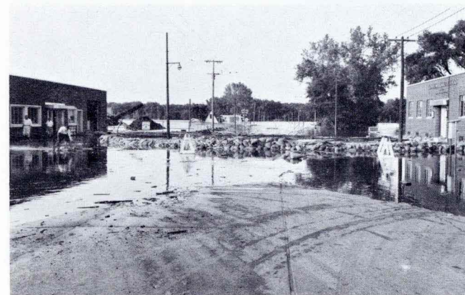
Looking south on Sixth Avenue from New York Avenue — June 24, 1954 flood.
