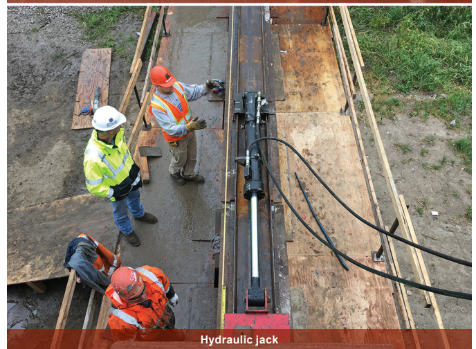
Slide-in equipment for the IA 1 Bridge over Old Man's Creek
