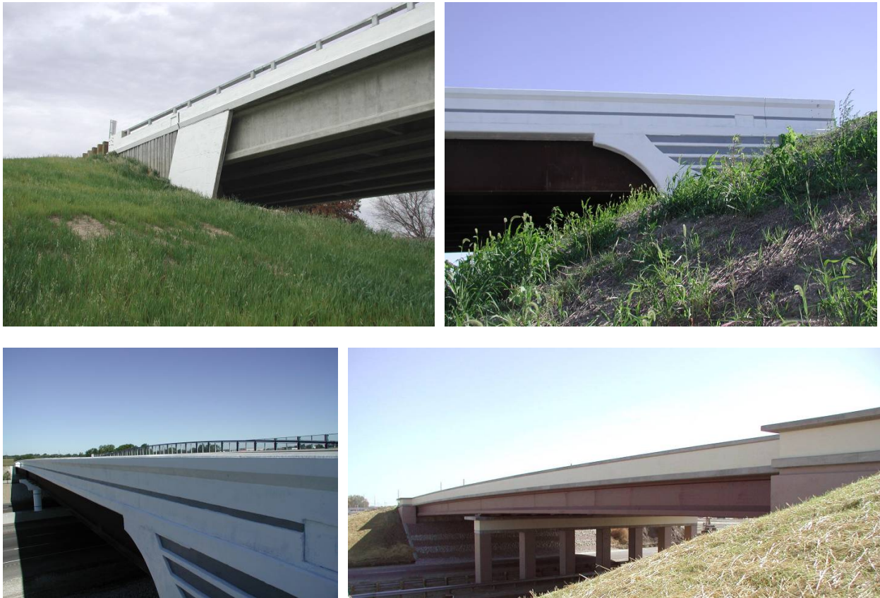
Figure 9.5.3.1. Bridges with long, slender appearance
