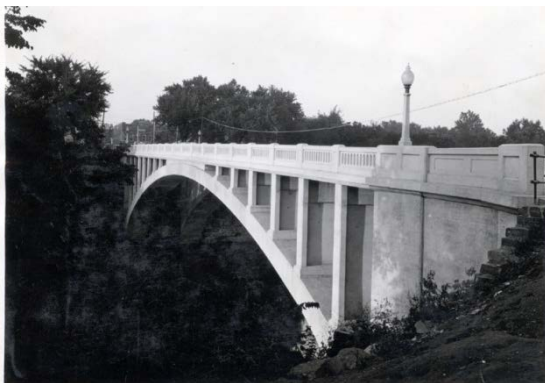
Figure 2.3.1-1 Original Concrete Arch Bridge
