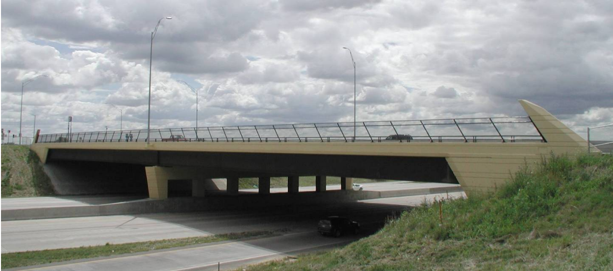
Figure 9.5.3.6. Bridge with sloping mask wall
