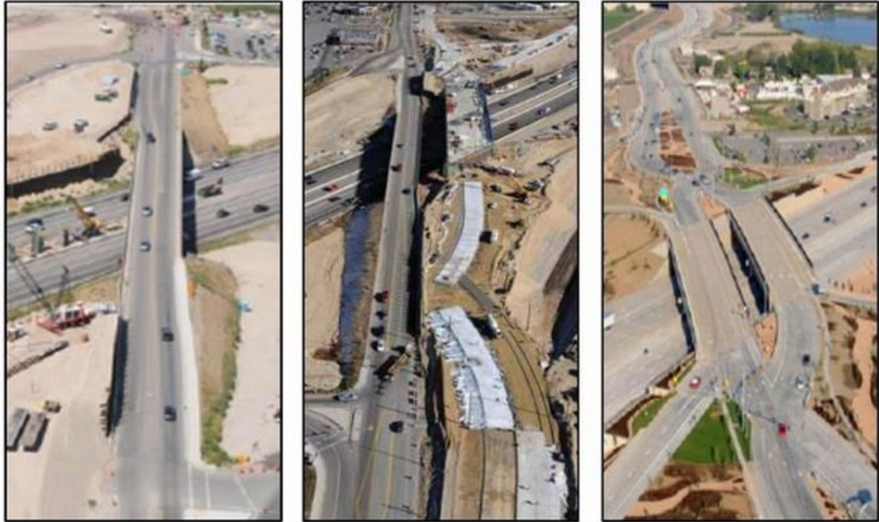
Figure 2.3.3 Construction staging using pre-cast construction methods
