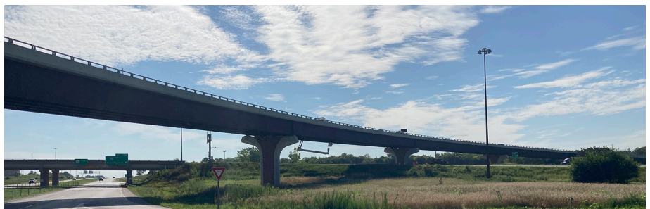
Story County bridge
