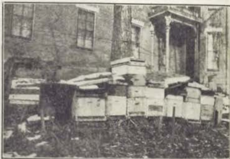
Equipment left to the elements soon loses its value.
