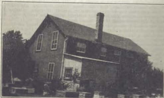
The central extracting plant
