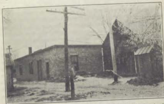
A poorly located city well. Note privies at right and left within few feet of well. Well is under brick building.
