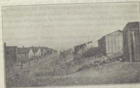
Such conditions should not exist in Iowa. Note mature rubbish, raw privies and well at foot of shops before driveway.
