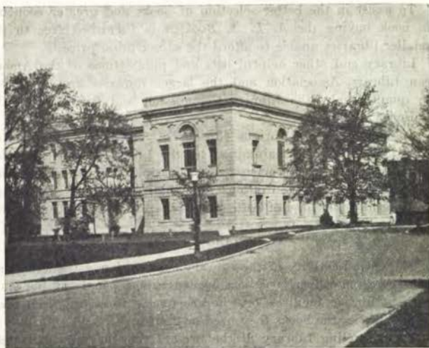
New Library Building at Iowa State College
