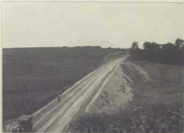
Filling the Hollows—Primary Road No. 37—Turin to Soldier, Monona County.
