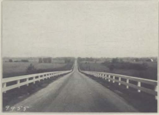
9955 Standard Permanent Guard Rail—Carlisle Road—Looking north from Avon overhead crossing. Polk County.
