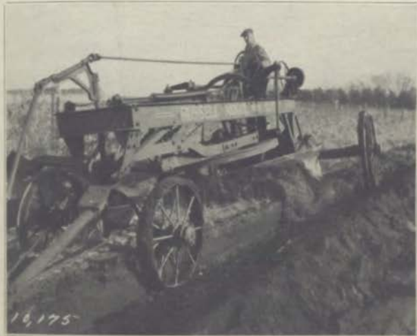
Burying the Sod—Turning the weeds and rubbish into the trench. Story County.
