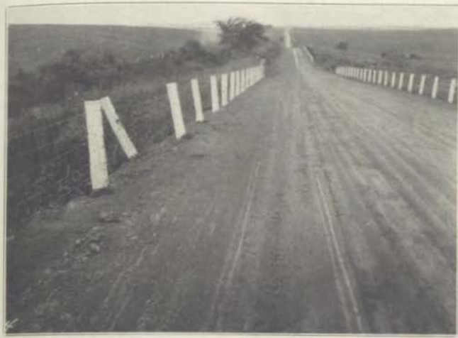
Wire Mesh Distributes Strain When Car hits post on Standard Temporary Type of Guard Rail—Primary Road No. 8. Adams County.
