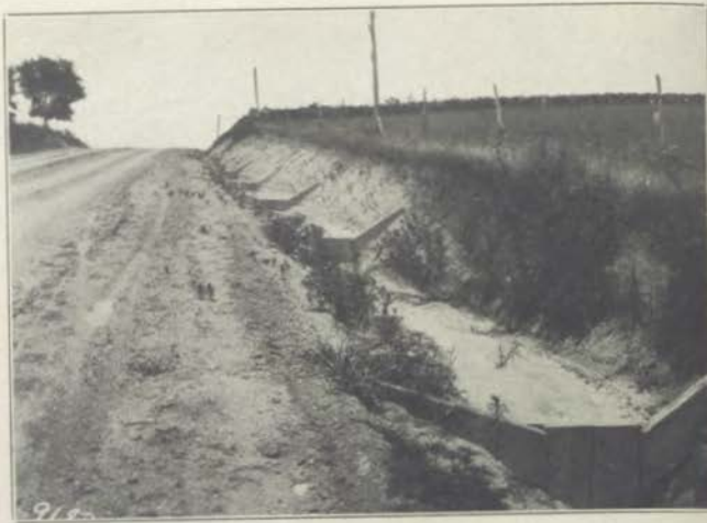
914 Preventing Side Ditch Erosion by Wooden Baffle Walls. Primary Road No. 16—Taylor County.
