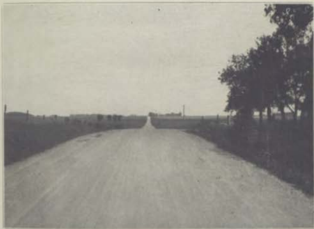
Gravel Road—Perfect Maintenance, Sac County.
