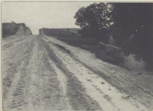
Cutting Through the Hills—Primary Road No. 37—Turin to Soldier, Monona County.
