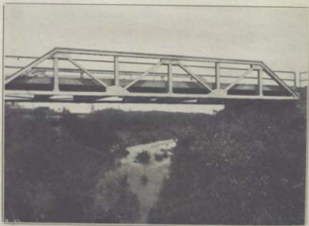
Standard Low Riveted Steel Truss with Concrete Floor.
