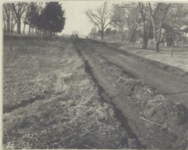
Burying the Sod—Trench made first round trip of grader. Story County.
