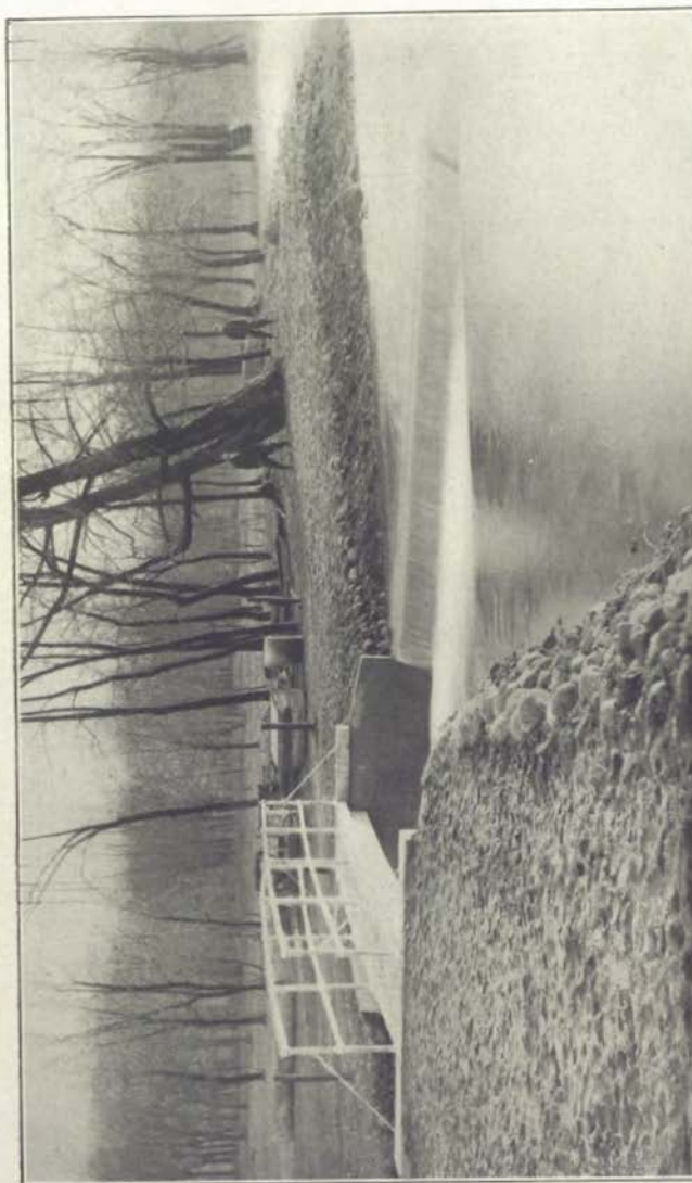
New Dam at Clear Lake with 54-foot spillway for 12-foot outlet. Designed by Highway Commission and Paul Graham, department's engineer, built by Waugh & Sons Construction Co. Similar dams under construction at Rush lake and Silver lake, Palo Alto county; Eagle lake, Hancock county; Trumbull lake, Clay county; Elm and Cornelia lakes, Wright county. Built 1918.
