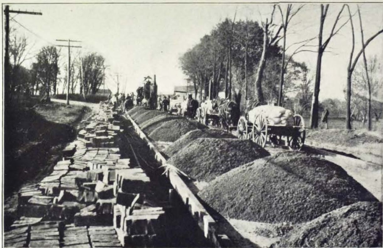
Construction view on road leading from Des Moines to Camp Dodge. This pavement is of monolithic brick construction, 20 feet wide and 8 inches thick. It is five miles in length. The contract was let in September, 1917. This road is being built for the purpose of carrying the excessively heavy military and civilian traffic between the city of Des Moines and the army cantonment. The points were previously connected with a gravel road which, under the ordinary traffic was satisfactory, but which proved wholly inadequate to carry the heavy motor trucks and numerous motor cars after the camp was established.
