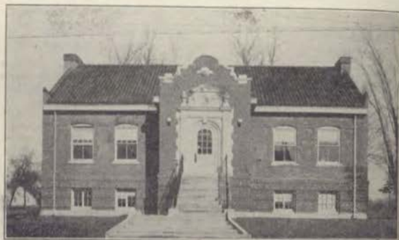
BEDFORD PUBLIC LIBRARY—CARNEGIE BUILDING.
