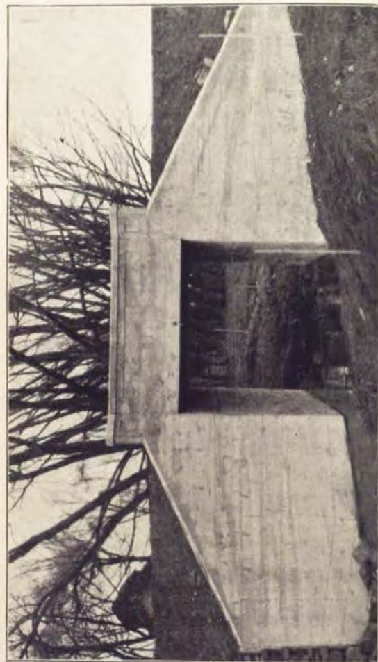
Standard Box Culvert.—This photograph shows a standard design 12"x12" reinforced concrete box culvert. It was constructed by day labor in Fayette county during 1916. The cost complete was $602.40. Careful attention to construction details, produced in this culvert, a completed structure, that not only has the requisite strength, but that is pleasing in appearance. There were 4,800 culverts of this type constructed in Iowa during the season of 1915.
