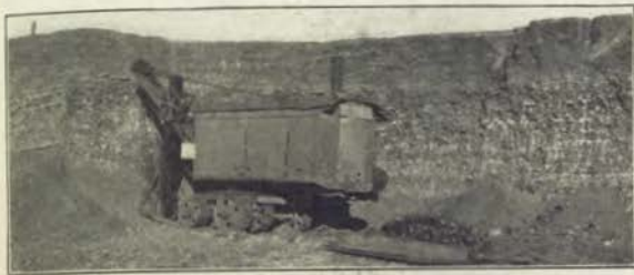
Farley Chert Gravel Pit—The pit from which the surfacing material for the Dubuque-Dyersville post road is being secured, is located 1½ miles north of Farley. The gravel is about 2½ in depth and in the plot purchased by the county there is estimated to be enough material to build another 20 mile road like the post road. The gravel consists of angular fragment concretionary limestone, ranging in size from ¼" up. It contains 25% of clay binder. In the construction of the road it is necessary to add sand or gravel to the surface to take up the excess clay binder.
