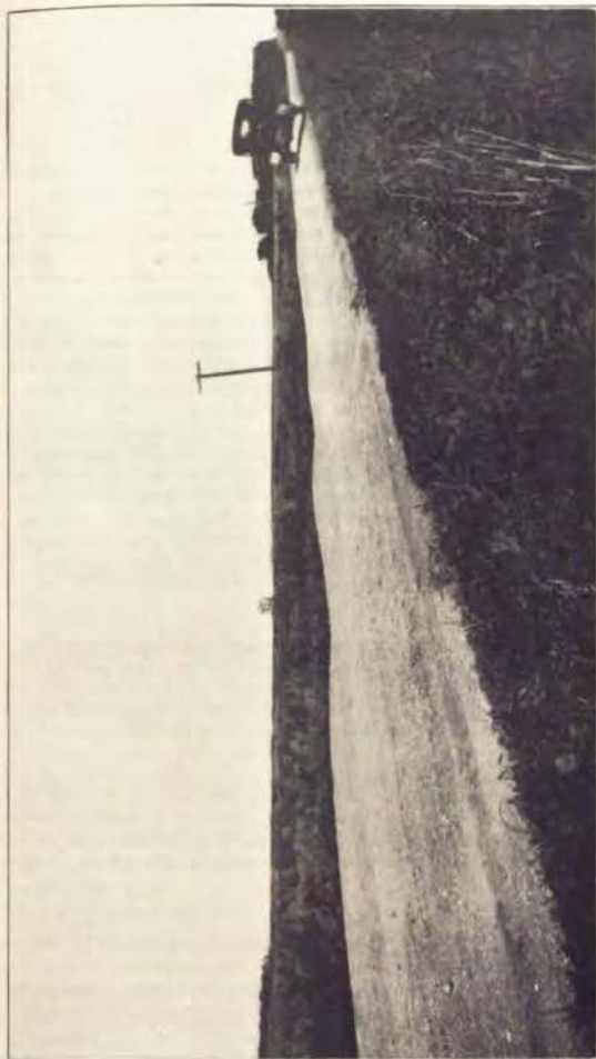
Waxy Gravel Road.—This condition was due to faulty construction together with lack of proper maintenance. Such a road is decidedly unpleasant for travel. It was repaired by scarifying and reshaping.
