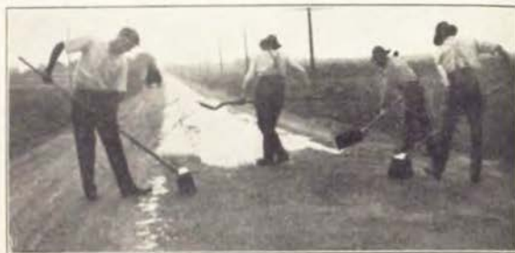
Sanding the Freshly Oiled Gravel Road—This view shows the spreading and brooming of the thin layer of coarse sand which was applied to the freshly distributed oil asphalt on the mile of experimental gravelled road at Ft. Dodge.
