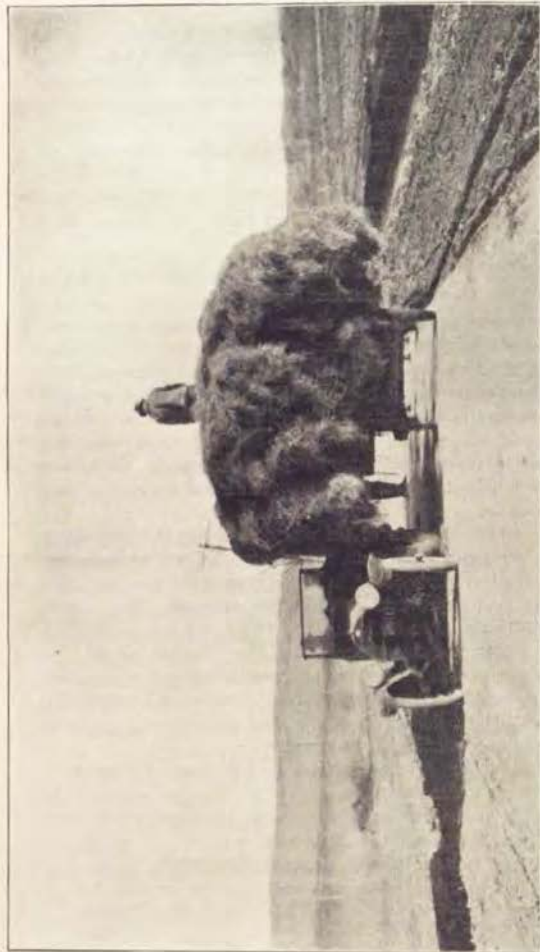
A 16' Concrete Roadway—This photograph shows an automobile and an extremely wide load of hay, passing on one of the 16' concrete roadways leading out of Sioux City. The auto can safely pass the load of hay on this width of roadway. Near cities and towns, double track roads should be provided. In the rural districts single track roads will, for the most part, meet present traffic demands. In some of the eastern states motor trucks have been developed of such width as to render a double track road serviceable only for single track traffic. Iowa should anticipate such a development of the motor truck by passing adequate law limiting the size and weight of such machines.
