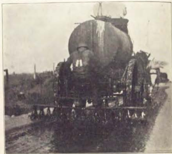
Applying Road Oil on Gravelled Road—This view shows a pressure distributor applying oil asphalt on the mile of experimental gravelled road at Ft. Dodge. The oil asphalt was put on in two applications of \frac{1}{4} gallon each.
