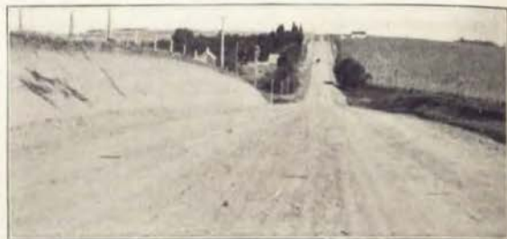
Crawford County Permanently Graded Road—Approximately 1,600 miles of such permanent grading work has been done in Iowa since the passage of the Highway Commission Road Law. Note the width and the attractive finished appearance of this particular piece of Crawford county grading.
