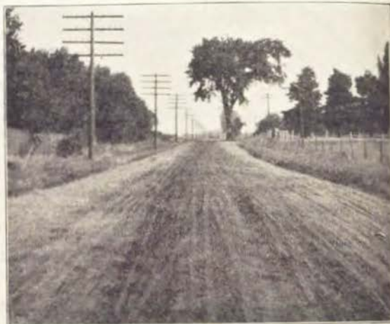
Ankeny-Des Moines Oiled Cinder Road—This view shows the condition of this important road about two weeks after oil was applied. It shows that section on which ordinary road oil was used; other types of oil being used on other sections. The entire road later became so uneven and rough that it was scarified and reschaped.
