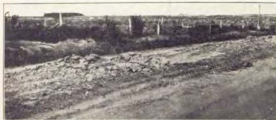
Gravel Humps on a Wavy Road Loosened by Scarifier—This view shows the wavy gravel road after the first passage of the scarifier. Successive passages tear up and loosen the whole surface of the road. The scarifier blade is then removed, the grader blade replaced and the loosened gravel reshaped. While the gravel is being repacked by traffic it is necessary frequently to reshape the surface to preserve the crown.
