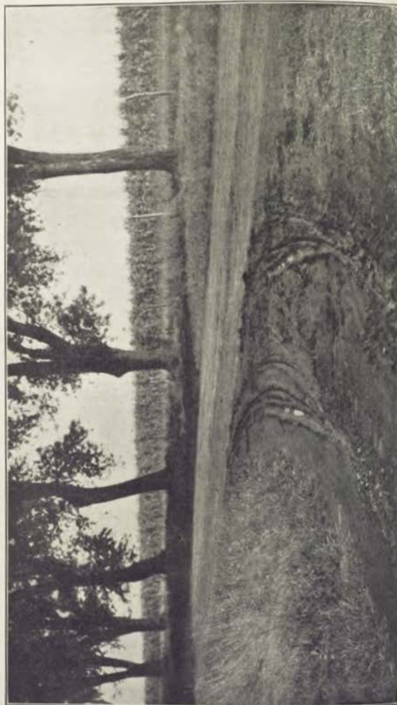
Oiled and Un-oiled Earth Road.—This view affords an excellent comparison. It was taken on the River-to-River road east of Grinnell a few hours following a heavy rain storm. There had been heavy traffic, even during and following the rain storm, over the oiled section, and but little traffic, not more than two or three vehicles over the un-oiled road.
