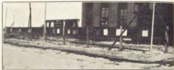
Paint Service Tests —This view shows the method of testing paints under actual service conditions as conducted by the Engineering Experiment Station at Ames, under the direction of the State Highway Commission. The panels shown on the long rack are each painted with a well known brand of paint, and a complete record of the results of the tests on each panel is kept.
