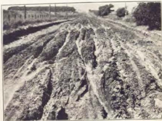
Poorly Graded and Drained Earth Road—This photograph provides a typical view of a poorly graded, inadequately drained earth road. This happens to be a township road, but no doubt there are many equally as bad stretches on county road system. It is a waste of money to attempt to place such a road in serviceable condition by the addition of gravel or stone. Side ditches should be provided and the roadway crowned so as to drain the surface water into the ditches.
