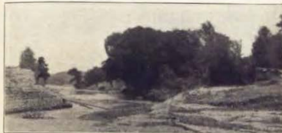
Site of the Clermont Arch—This photograph shows all that was left of the pony truss which formerly occupied the present site of the Clermont arch shown in a previous picture. Every particle of the old bridge was washed away, including even the abutments.
