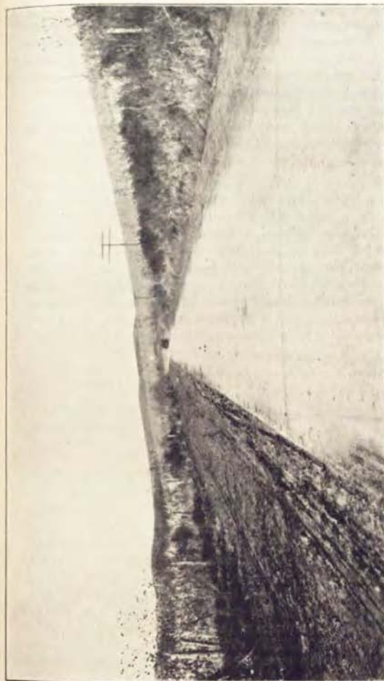
An Iowa Paved Country Road—This photograph gives a view of a 36' concrete road built under the Farr Paving Law district plan. Under this plan, Sioux City has constructed approximately 20 miles of concrete roadways. These roads have been built on the main travelled high ways leading into the city from five different directions. While inside the city limits, almost the entire mileage is through strictly rural territory. Note that on each side of the road in the picture, there are cornfields. The entire mileage cost approximately $300,000.
