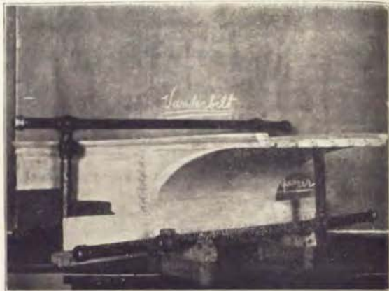
Curved Wing Wall Model—This photograph shows the model of a bridge on the Vanderbilt estate in New York. It was prepared for the suit of Luten vs. State of Iowa. It was used to illustrate the idea of using the curved wing wall to curb the top of the slope of approach fills.
