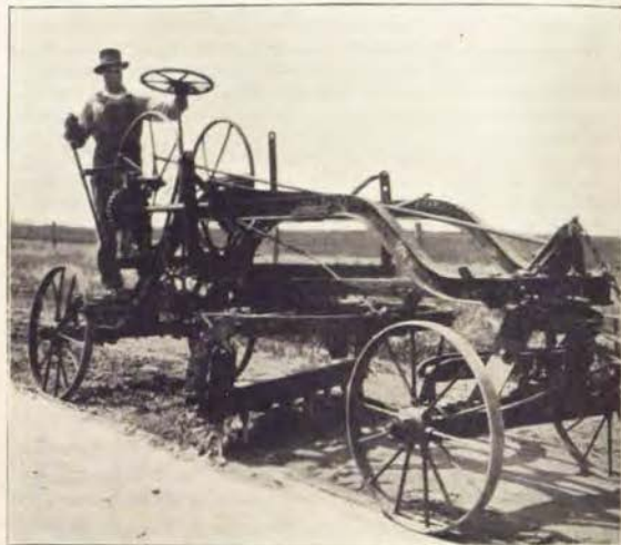
Scarifier Attachment on Blade Grader—This type of machine does very efficient work. The view shows the scarifier in action on the wavy road shown on a previous page.
