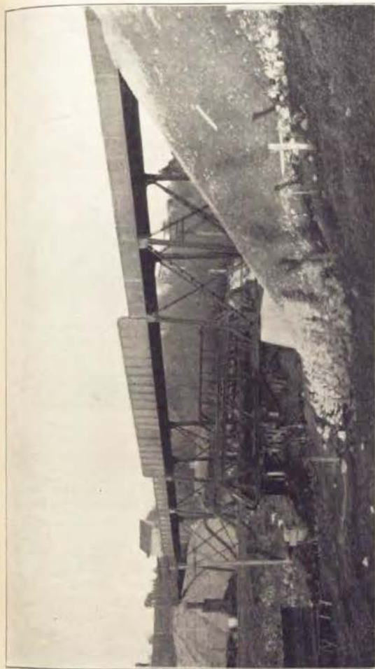
Center Grove Railroad Crossing—The Center Grove viaduct which carries the Dubuque-Dyersville Post road over the Illinois Central railroad tracks, a short distance west of Dubuque, is the most important separation of highway and railroad grade yet attempted in Iowa. This is a triple crossing. At the same point at which the highway crosses the railroad track, Cat Fish branch down beneath the railroad bridge. The bed of the creek, the Illinois Central low riveted truss bridge, the steel highway viaduct and the old steel through truss which formerly carried the road over the creek, are all visible in the photograph. Cost of improvement was $24,000.
