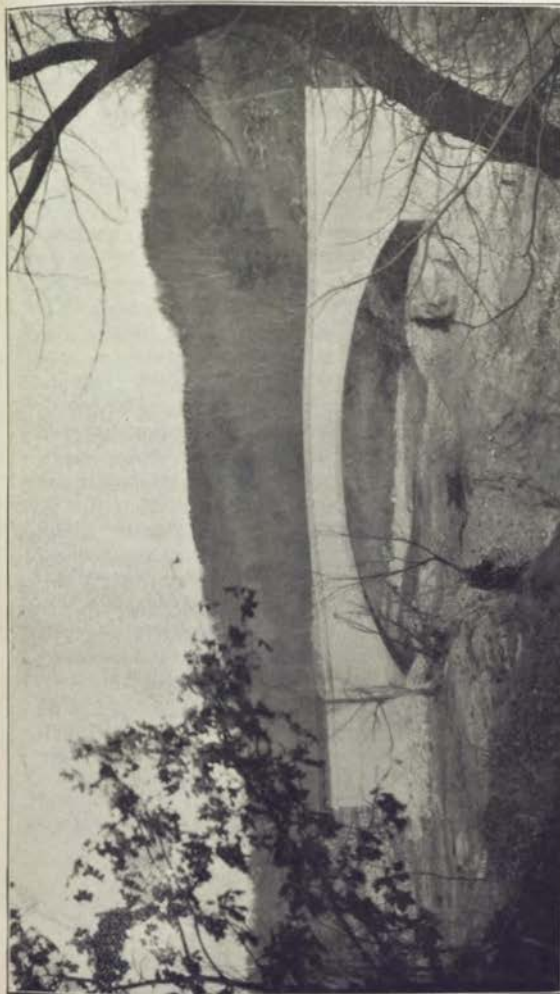
Clermont Concrete Arch Bridge—A flood June 1, 1916, swept away the light steel truss which spanned Dibble Creek in the edge of the town of Clermont, Fayette county. The old truss and abutments were completely destroyed. Notes were secured for a new design and plans prepared by the Commission. The contract for the new bridge was awarded June 23d, the contract price being $2,000 for the 60' arch. Bridge was completed September 25, 1916.
