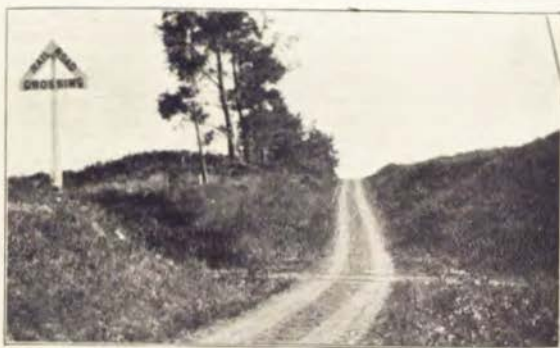
Dangerous Type of Grade Crossing. —The type of grade crossing on which both the railroad crossing and the highway, are both in cuts, is in general, the most dangerous of grade crossings. This view shows a crossing on the Great Northern R. R., five miles north of Perkins in Sioux county. It is No. 86 in the list of crossings scheduled by the Highway Commission for improvement. Present day traffic demands the elimination of the dangerous railroad crossing of this kind.
