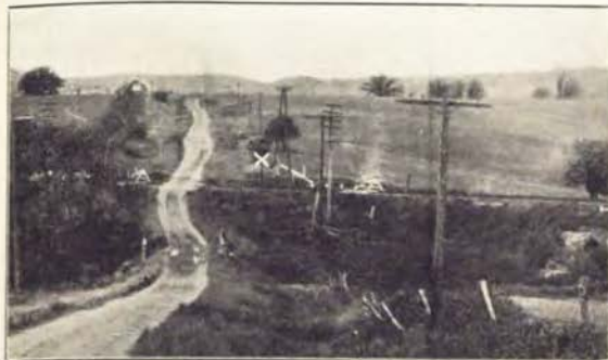
Julien Crossing on Dubuque Post Road—This view shows the old road and the site of the present 180' wooden viaduct which carries the Dubuque Post road over the Illinois Central railroad tracks near Julien. At the point where the creek crosses the highway in the foreground a 4'x4' box culvert, 140' in length has been constructed. The fill at this point is 25' high.
