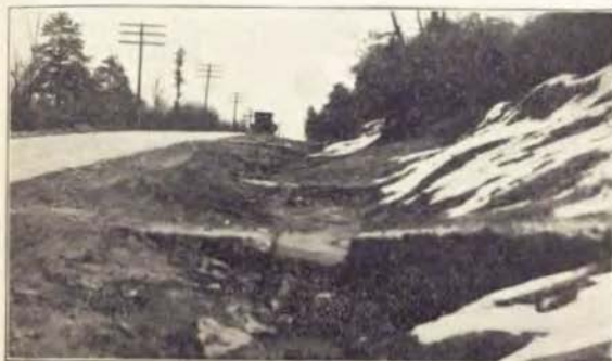
Preventing Erosion in Side Ditches—This view illustrates the method of preventing erosion in the side ditches on hillsides on a Maryland state road. At frequent intervals walls or dams are constructed across the side ditches. The top of each wall is placed at the proper elevation to retard the flow of water, and yet not force the water out of the ditch. The slope of the ditch between excessive dams is flat enough to prevent washing. This same scheme can be cheaply applied to Iowa roads by using plank or logs to form the dams.
