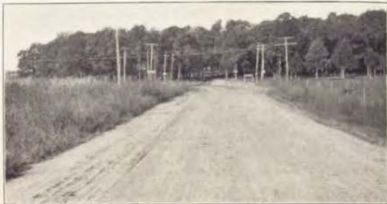
Class "A" Gravel Road—This is a view of the Spirit Lake-Arnold's Park experimental gravel road. Class "A" gravel road requires approximately 2,450 cubic yards of gravel per mile for a 16' roadway. Specifications require that it be built upon a standard cross-section, permanently graded earth road. The lower course of gravel is placed in a trench 9' wide and 5" deep. The top or wearing course of gravel is distributed over a width 16' and 5" deep. A roller is used to compact the earth subgrade and both courses of the gravel.
