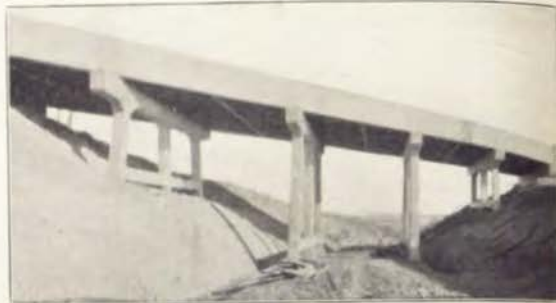
Concrete Pile Trestle Viaduct—The construction of the viaduct shown above was made necessary by the building of a switch track across the State farm to the institution buildings at the State Hospital at Cherokee. The viaduct carries the Hawkeye Highway over the railroad tracks. Prison labor was used throughout and the workmanship is first class.
