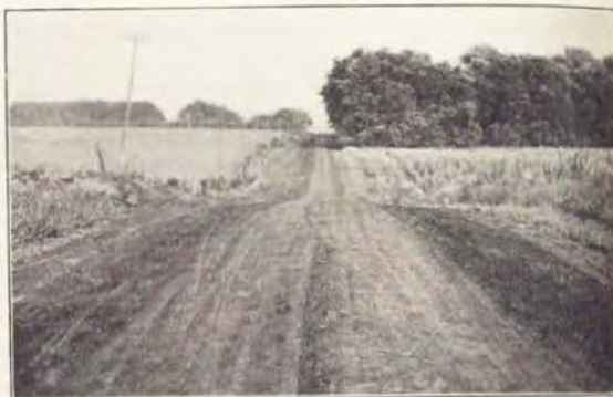
Oiled Earth Road.—This view shows a portion of the 8-mile section of the River-to-River road east of Grinnell, which was oiled during the season of 1916. This road was properly prepared before the oil was applied. The roadway being properly crowned the oiled surface easily sheds the water into the side ditches. During rainy weather the road was never in bad condition for travel.
