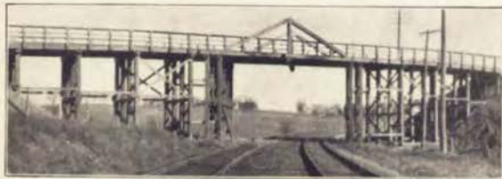
Wooden Overhead Crossing—This photograph shows the wooden structure which carries the Dubuque Post road, which is also a portion of the Hawkeye Highway, over the Illinois Central R. R. tracks near Julien in Dubuque county. This overhead bridge eliminates by grade separation a very dangerous double track crossing on this important highway. It also materially reduces the amount of rise and fall on the mile of road on which it is located.
