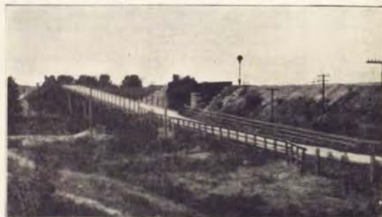
The Nevada Crossing Project—This photograph shows a general view of the Lincoln Highway crossing over the Rock Island R. R. tracks, east of Nevada. The highway is carried over the track on a poorly constructed combination of wood and steel viaduct. The floor of the viaduct is at a very steep incline. A short distance beyond the point shown in the extreme right of the photograph, the highway is carried again at a steep grade over the North-Western tracks on a grade crossing. Plans have been prepared for the replacing of the viaduct over the Rock Island and the construction of an undergrade crossing under the North-Western tracks. Negotiations are pending at the present time with the Rock Island, but have been completed with the North-Western. The estimated cost of the entire improvement is $50,000.
