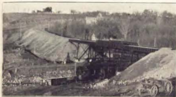
General View of Center Grove Crossing Project—This photograph shows the extensive fill and the steel viaduct which carries the Hawkeye Highway over the Illinois Central railroad at the Center Grove crossing west of Dubuque. The white house shown in the distance was moved from down in the valley because of the high fill which has been constructed. The fill near the far end of the viaduct is approximately 30' in height. This viaduct with the earth approaches was constructed by the co-operation of the Federal government, Illinois Central R. R. and Dubuque county. The railroad constructed and maintained the viaduct. The county and Federal government constructed and will maintain the earth approaches.
