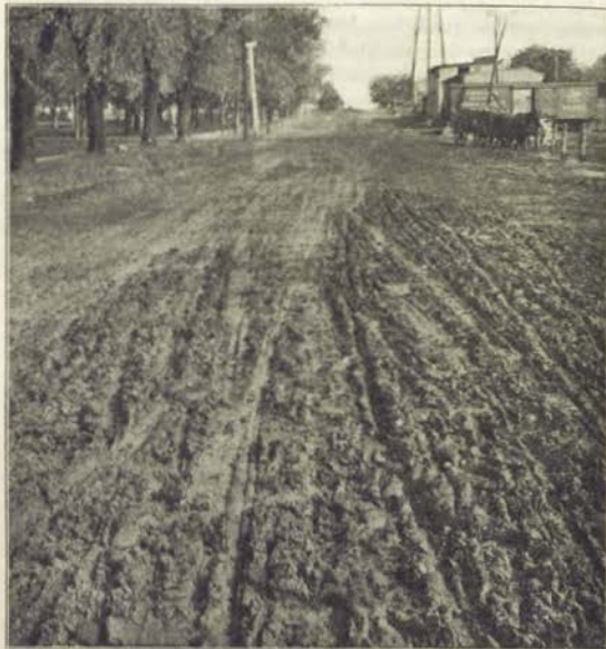
This view affords an excellent comparison of an oiled and unoled earth road. The background shows a portion of the road that has received an oil treatment. In the foreground appears the untreated road. The use of oil not only abates the dust nuisance, but in a large measure checks the penetration of water into the road surface and this tends to eliminate a rutted condition during wet weather.
