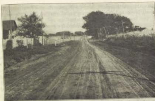
View of an oiled road a few days after a hard rain. When the roads in the surrounding sections were badly rutted during periods of extended rain, this road was never in worse condition than shows in the above view. It is quite possible by thorough and efficient application of the proper quality of oil, to render an earth road capable of better withstanding the wet seasons of the year.
