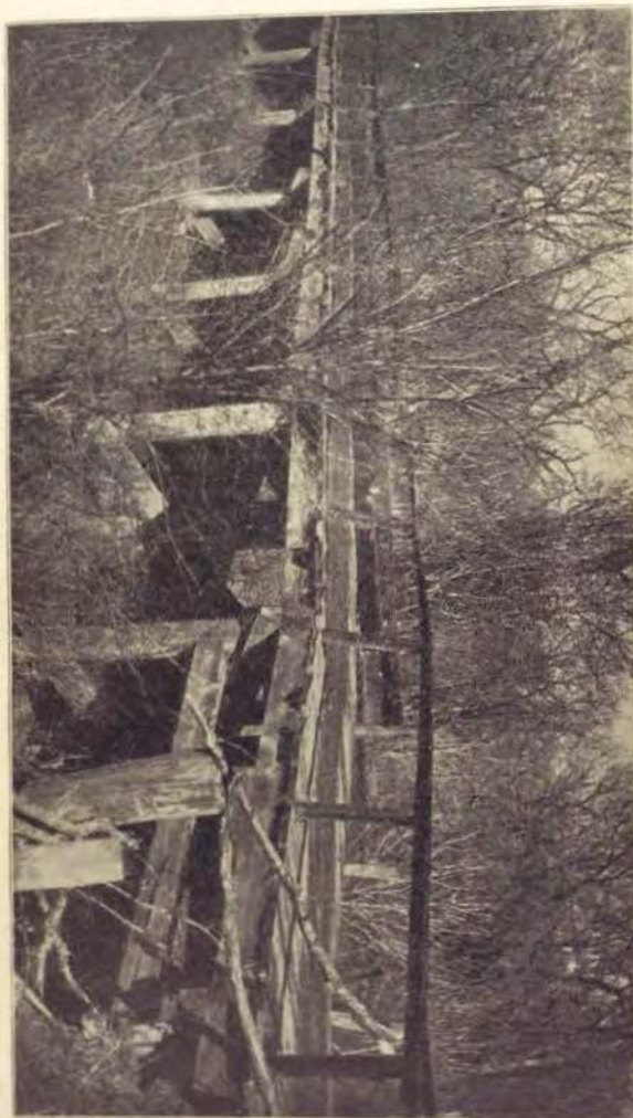
WOOD PILE TREESTLE BRIDGE. This type of construction is rapidly being replaced by permanent structures on the highways of this state. At the time this photograph was taken, three years ago, the county in which this bridge was located had 20,000 line ft. of this type of construction on its highways.
