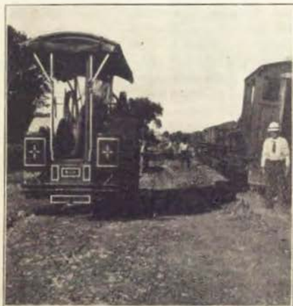
A view on the Dubuque-Dyersville post road. This photograph shows one of the work trains on the industrial railroad installed for the purpose of hauling material from the gravel pit at Farley.
