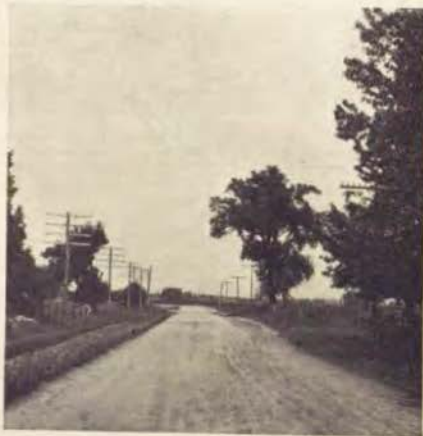
View of the old Military road in Dubuque county running southwest from Dubuque to Cascade. This road was built of the native limestone and has been in use many years. During the season of 1916 it is proposed to improve this stretch of road which extends out for about eleven miles from Dubuque and to gravel the remaining distance to Cascade.
