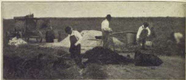
Convict culvert building crew at Woodward.
