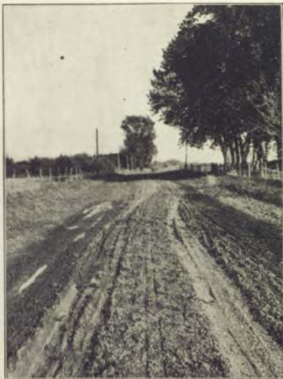
This picture shows the end of an oiled section on the Cedar-Fremont oiled road in Mahaska county. Note the clear line of demarcation where the oiled section leaves off.
