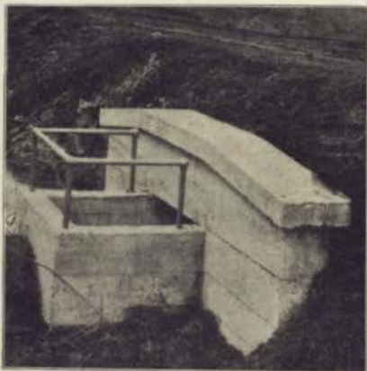
CONCRETE HEADWALL CONSTRUCTION.
