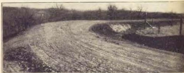
This view shows a typical rounded corner built according to the Iowa standard in Crawford county, during the season of 1915.
