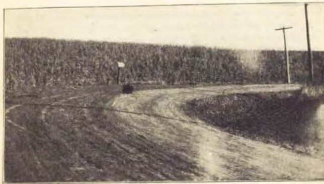
Crawford county has made it a rule to round all corners on all permanent work on county road system. This view shows a typical one of the rounded corners. Note that the traffic is almost entirely inside the original fence corner which is marked by the camera case. To round a corner like this it requires about 1-30 of an acre, fences being cut back thirty feet on each side from the corner.
