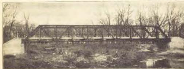
This cut illustrates the standard pony truss steel bridge. Approximately 250 of these structures were built in Iowa during 1915. This is a 90' span built in Chickasaw county.
