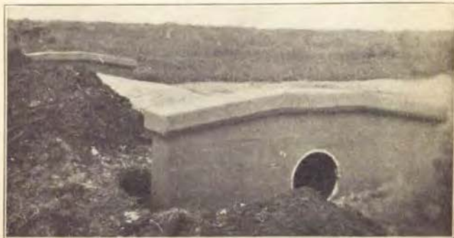
This culvert was built by convict labor. It is on one of the new roads built during 1915 at the Iowa Colony for Epileptics at Woodward. It is of the circular type, concrete, with straight bulkheads and coping.
