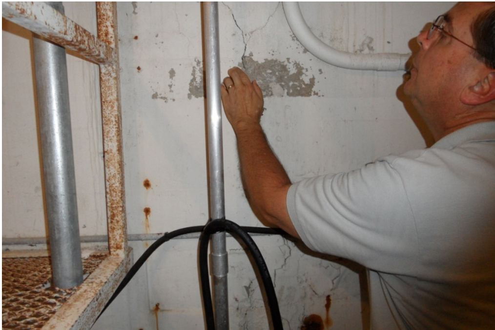
2.11 – Cracking in north wall of Control Room
