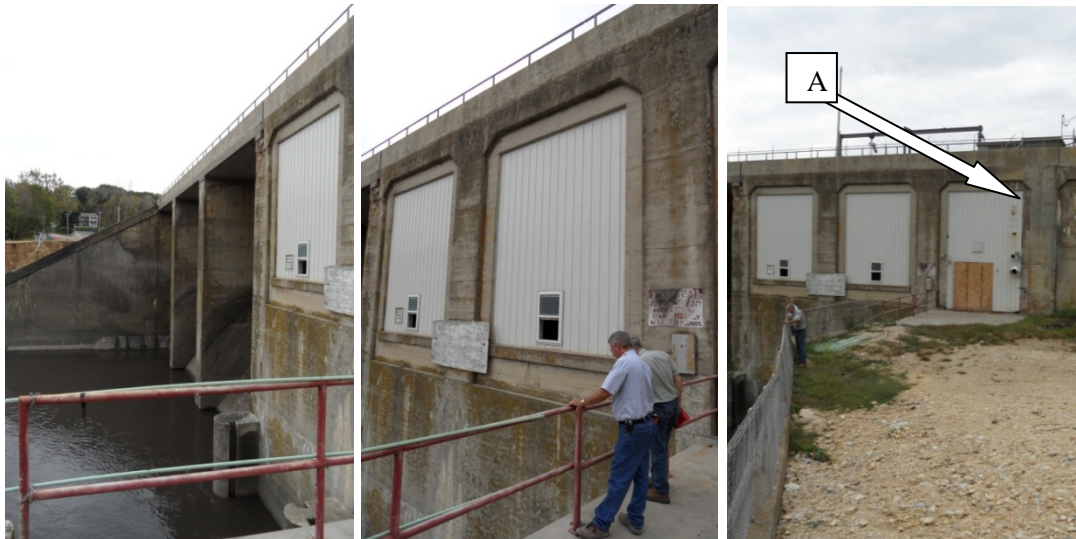
2.5, 2.6, 2,7 – Downstream side of Powerhouse – Concrete deterioration cracking and deterioration observed at location A
