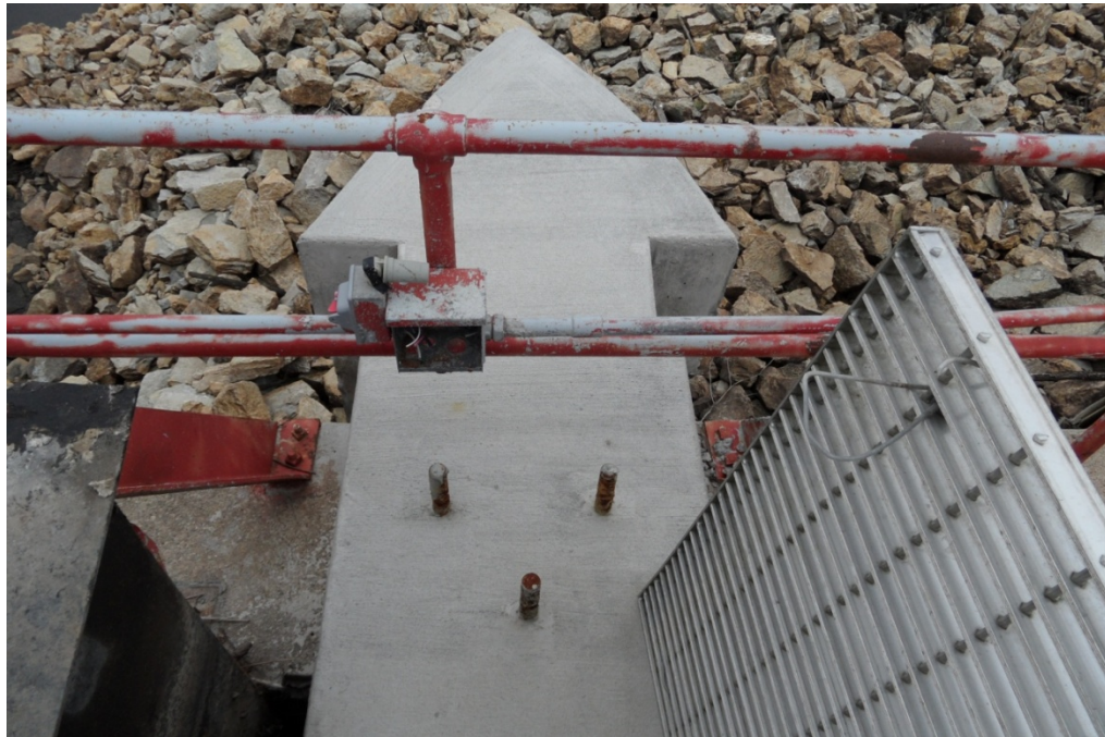
3.21 – Top of typical reconstructed pier with new equipment anchor bolts
