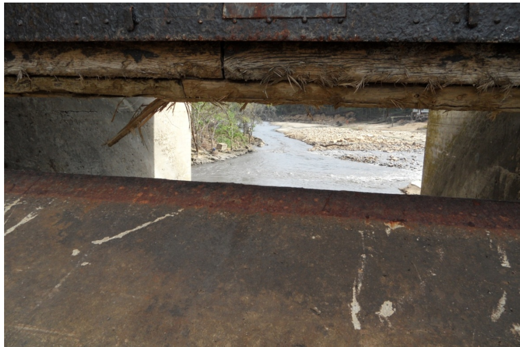
3.3 – Abrasions on the upstream side of a typical spillway
