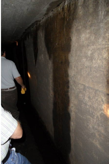
4.5 – Moisture and lime deposits on tunnel walls
