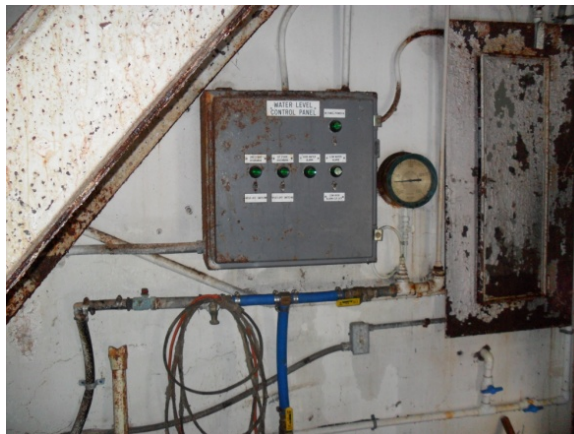
Water Level Control Panel Figure 2-9
