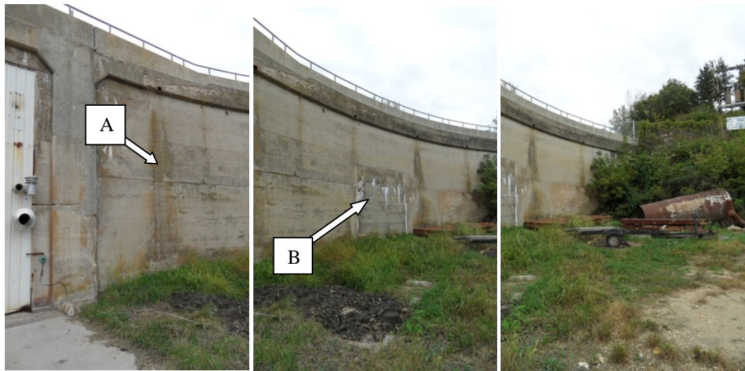
1.5, 1.6, and 1.7 – Downstream retaining wall – Note diagonal wall crack at location A – Note efflorescence at location B.
