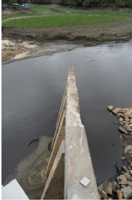
3.14 – Damage to top of upstream abutment wall
