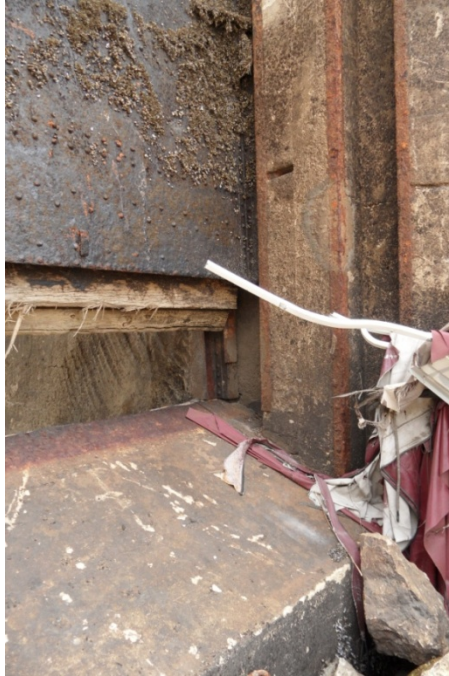
3.4 – Abrasions on the upstream side of a typical spillway
