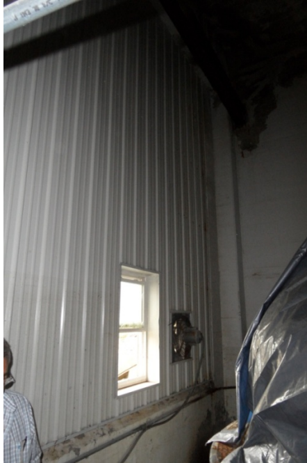
2.12 – Metal panels installed along downstream wall
