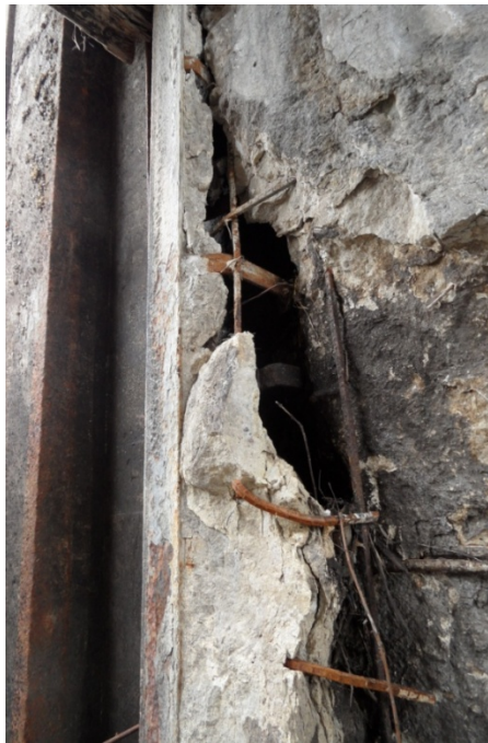
3.9 – Severe concrete deterioration in left pier at Gate 3 – Note how embedded steel guide slot has been pushed away from pier and is out of plumb
