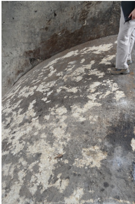
3.5 – Abrasions and erosion in downstream surfaces of a typical spillway
