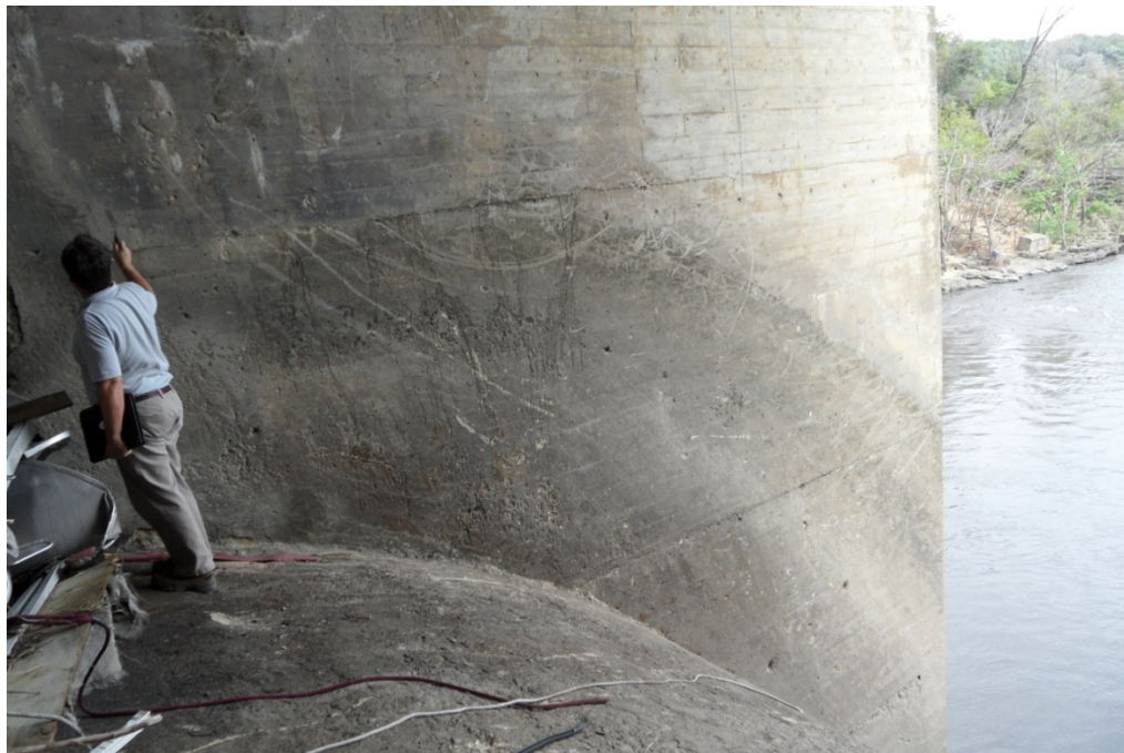
3.7 – Hollow sounding concrete when tapped with hammer at Gates 1 and 2
