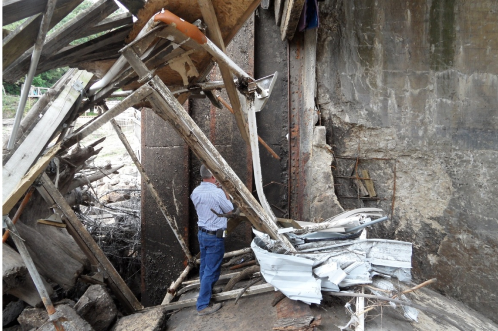
3.8 – Severe concrete deterioration in left pier at Gate 3
