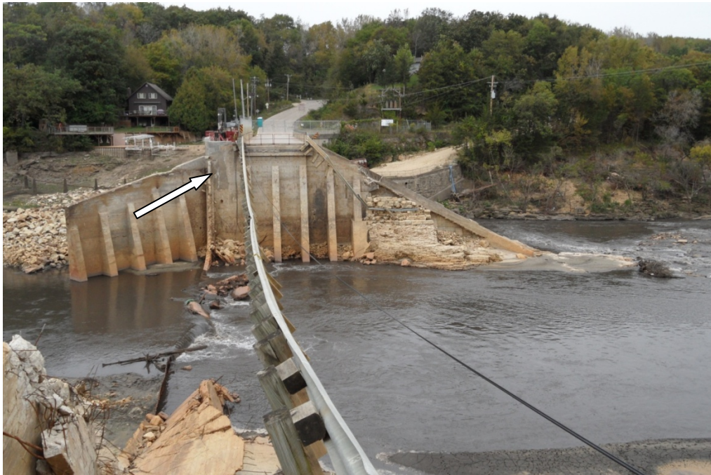
3.15 – View of abutment wall from south bank – Note area of previously patched concrete adjacent to remnants of cutoff wall
