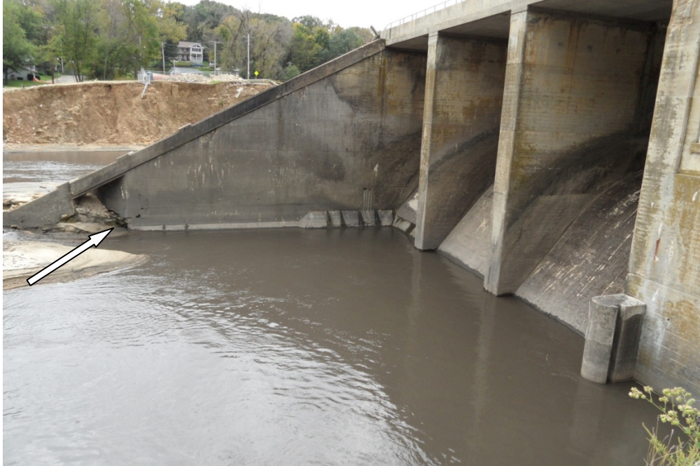
3.12 – Erosion of bedrock foundation under downstream end of abutment
