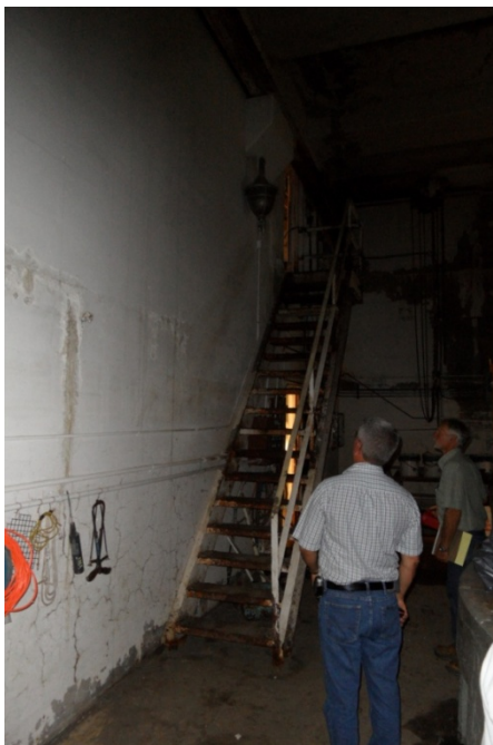
2.14 – Random cracking and efflorescence on upstream wall of Turbine Room
