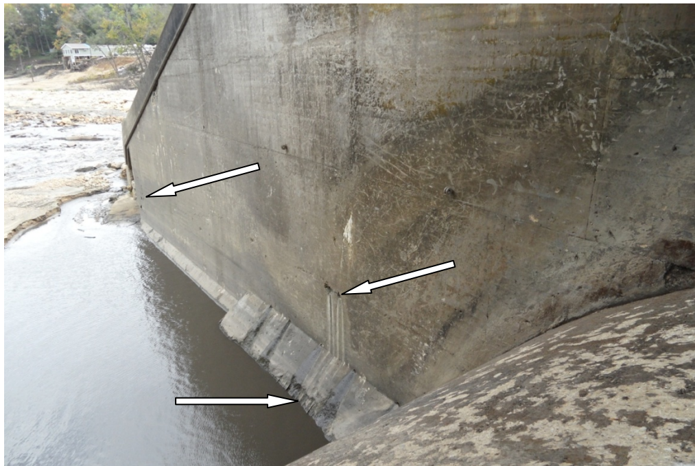
3.11 – Exposed reinforcing and holes in abutment wall downstream of spillway
