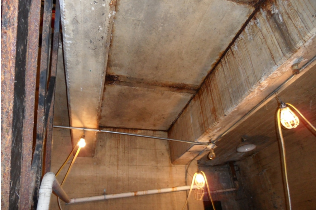
2.20 – Removable floor panels between Turbine Room and Mechanical Room – Note heavy corrosion on steel stairs and railings on the left
