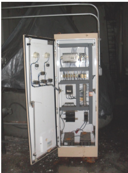
Hydroelectric Generator Control Panel Figure 2-10
