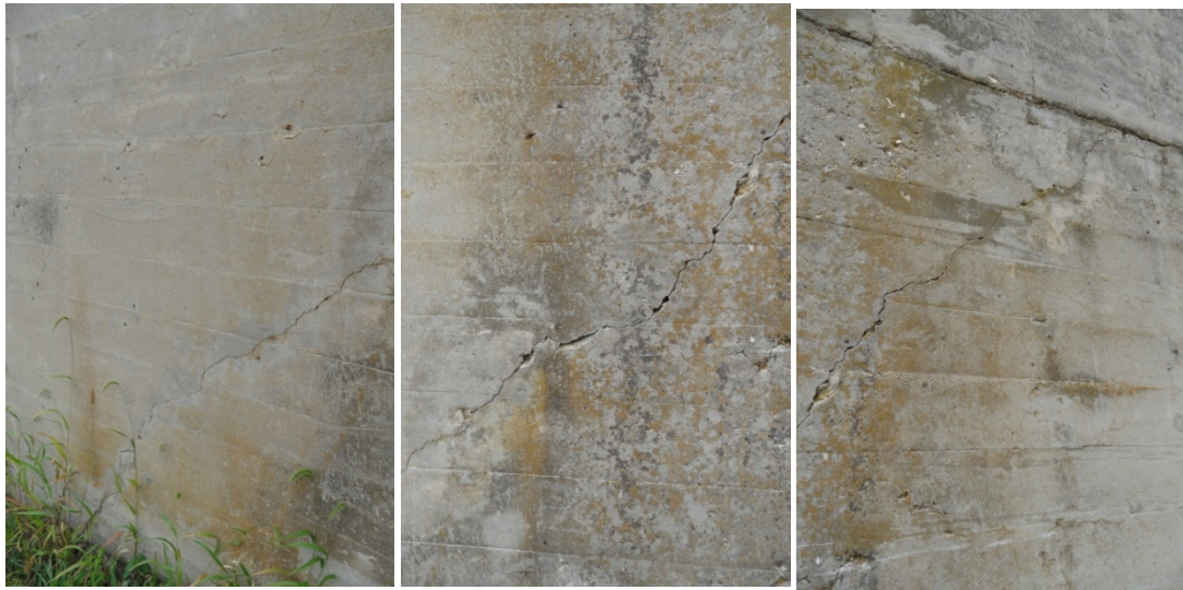
1.9, 1.10, and 1.11 – Diagonal crack in downstream retaining wall
