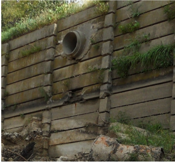
Photo 1.3 – Storm drainage pipe penetration through retaining wall – Note damaged concrete below pipe
