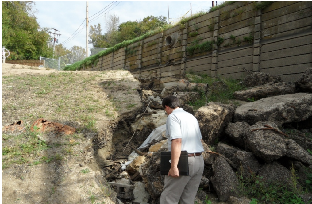
Photo 1.1 – Upstream retaining wall adjacent to north approach roadway – Note eroded area in front of wall partially filled with riprap
