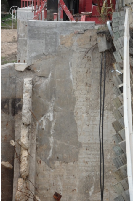
3.16 – Close-up of abutment wall repair area
