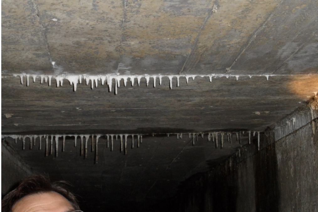
4.3 – Moisture and lime deposits on tunnel walls
