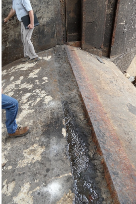
3.10 – Typical condition of embedded steel guide slots and seal plates
