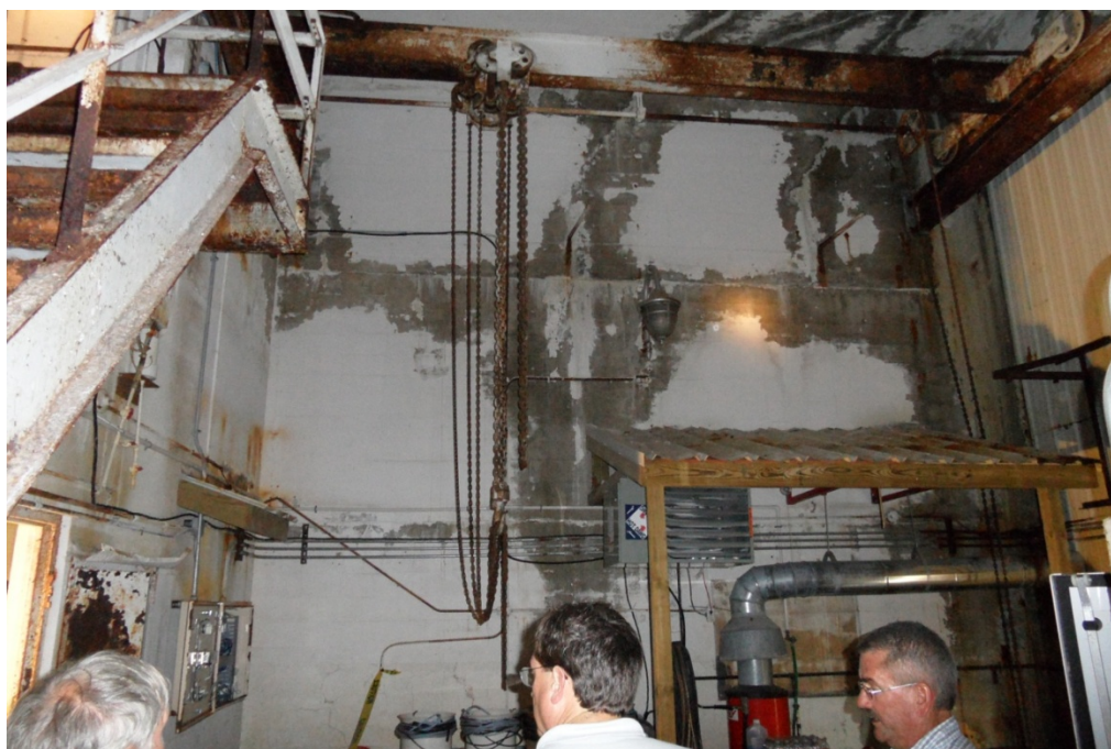
2.15 – Cracking in north wall of Turbine Room
