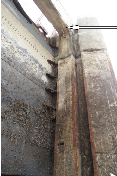
3.22 – Cracking in beams on upstream side of operator's deck
