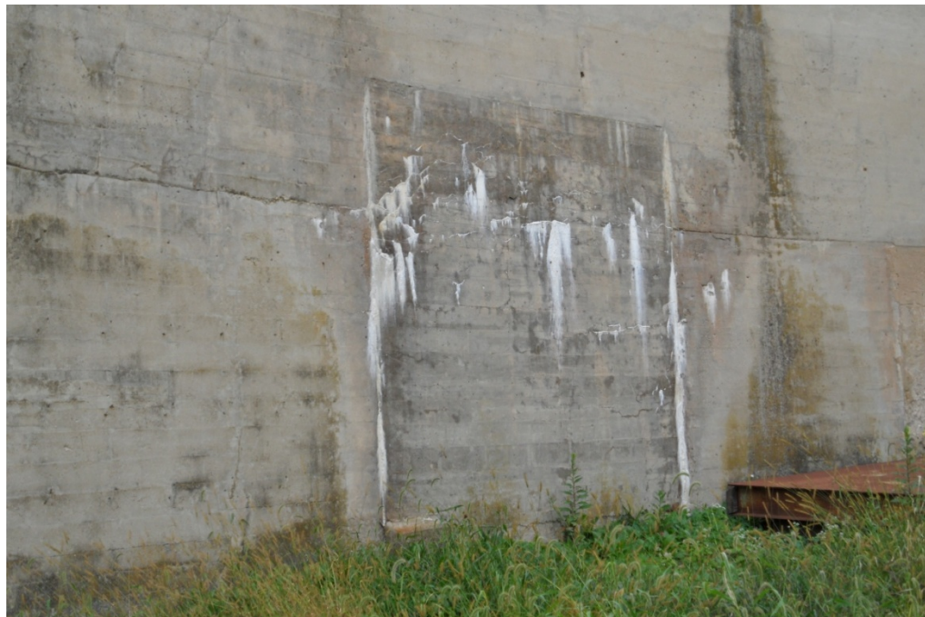
1.9 – Efflorescence around cracks in downstream retaining wall
