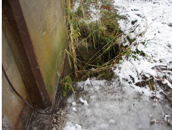
Material Loss Downstream of North Embankment Wall Figure 2-3
