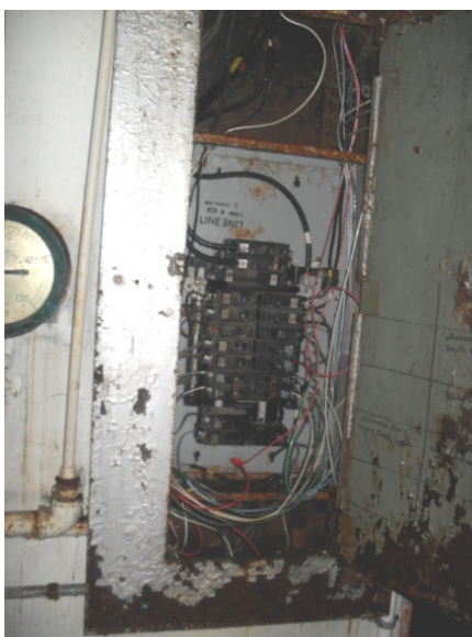
Distribution Panelboard with No Cover Plate Figure 2-7
