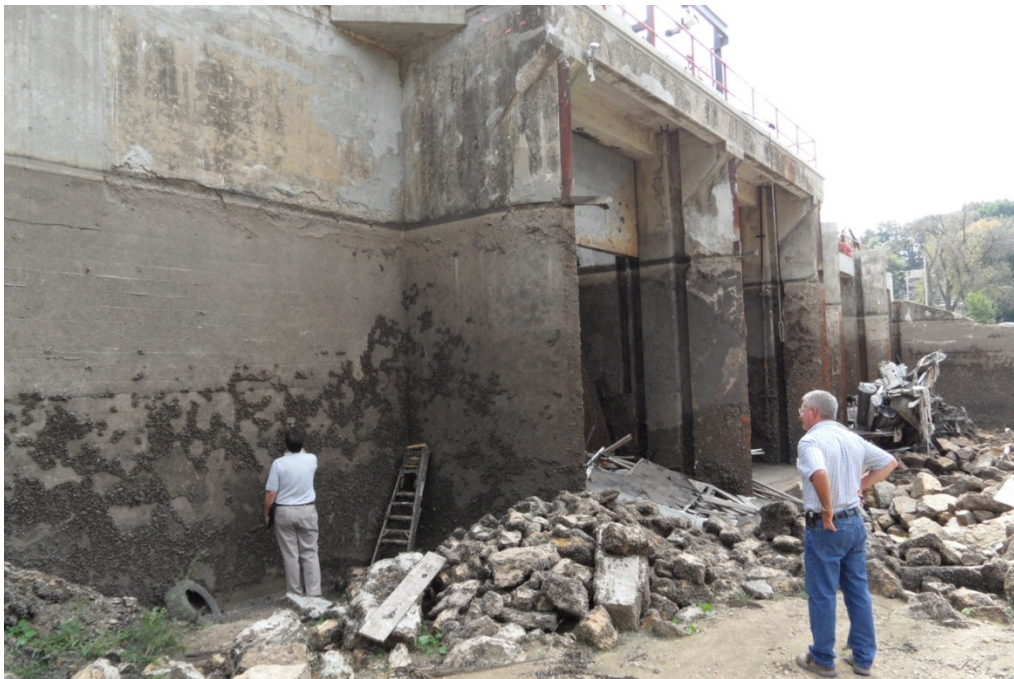
2.3 – Upstream side of Powerhouse – Note apparent spalling and past repairs above original waterline
