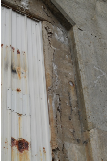
2.8 – Deterioration in downstream wall of Powerhouse
