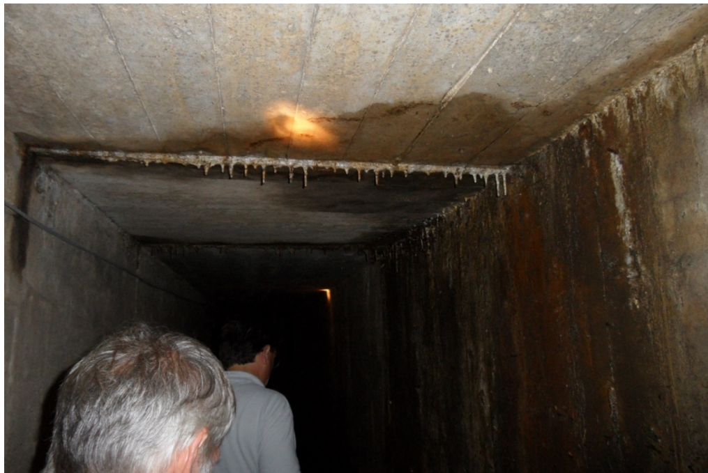
4.2 – Moisture and lime deposits on tunnel walls
