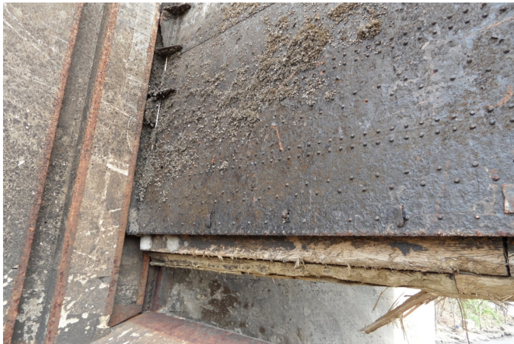
3.19 – Typical timber gate bottom seal
