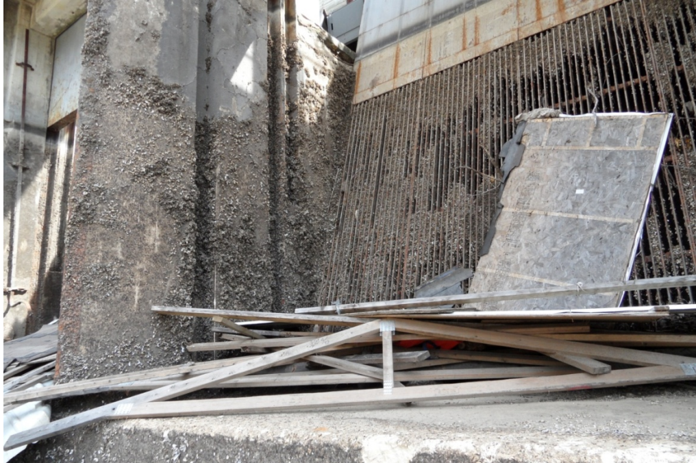
2.4 – Debris and marine growth on upstream side of turbine bays
