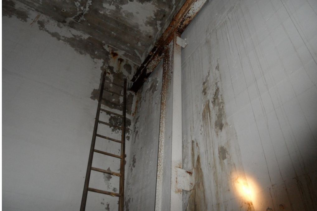
2.16 – Cracking near top of south wall of Turbine Room
