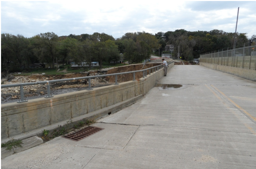
Photo 1.2 – Storm water intake in approach roadway
