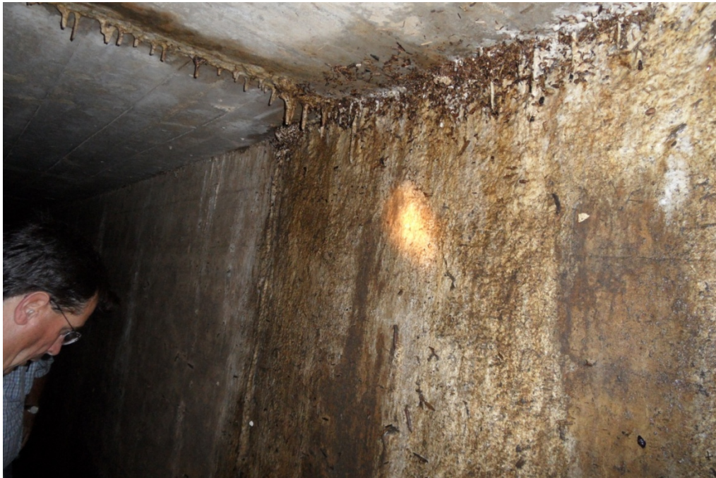
4.4 – Moisture and lime deposits on tunnel walls
