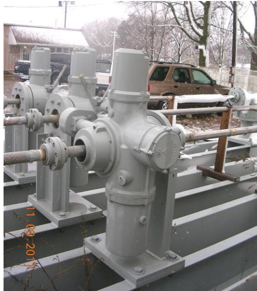
New Gate Hoisting Mechanism
