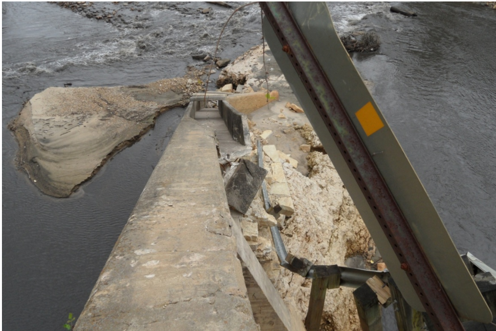
3.13 – Top of downstream abutment wall – Note remnants of abandoned fish ladder structure built into wall
