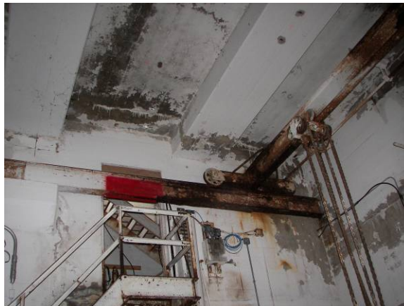
Powerhouse Roof Seepage Figure 2-2
