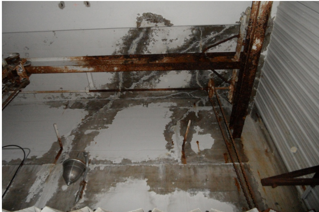
2.17 – Cracks in Turbine Room roof and north wall
