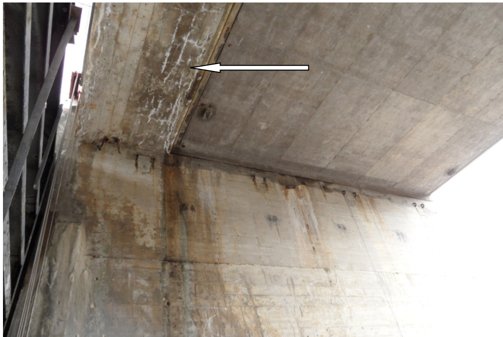
3.23 – Cracking and efflorescence in concrete beams on downstream side of operator's deck
