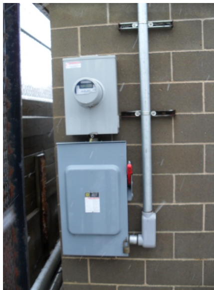
Meter and Main Service Disconnect Figure 2-4
