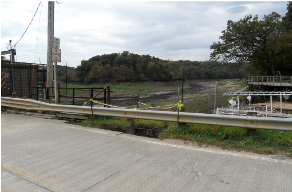
Photo 1.4 – Cracking and settlement in the approach roadway – Note the loss of shoulder material beyond the edge of roadway
