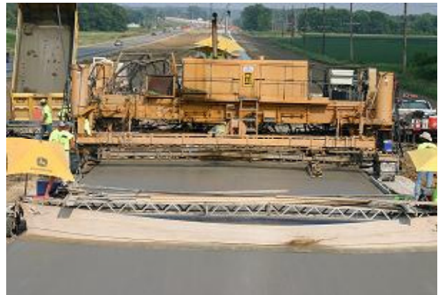
Burlap drag attached to paver
