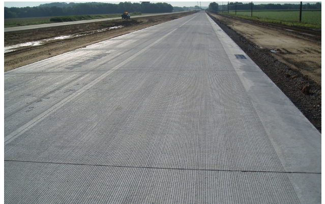
Longitudinal texture on concrete pavement
