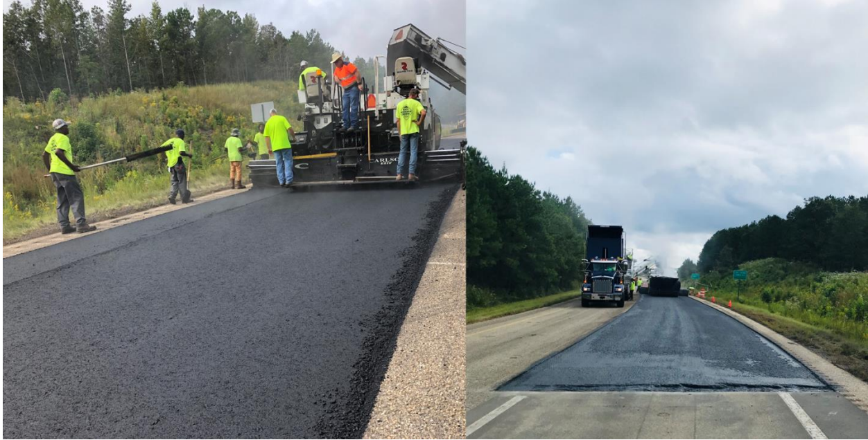
Figure 14. NCAT Test Track paving and compaction using biopolymer-modified asphalt mixture
