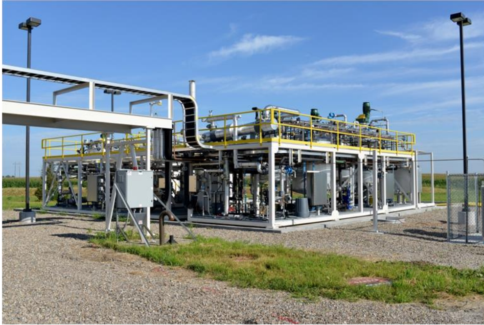
Figure 13. Iowa State University's vegetable-based biopolymer pilot plant facility
