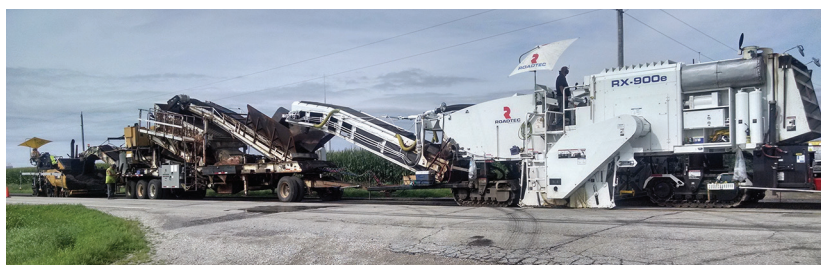
Roadway test section showing application of holding strategy treatment
